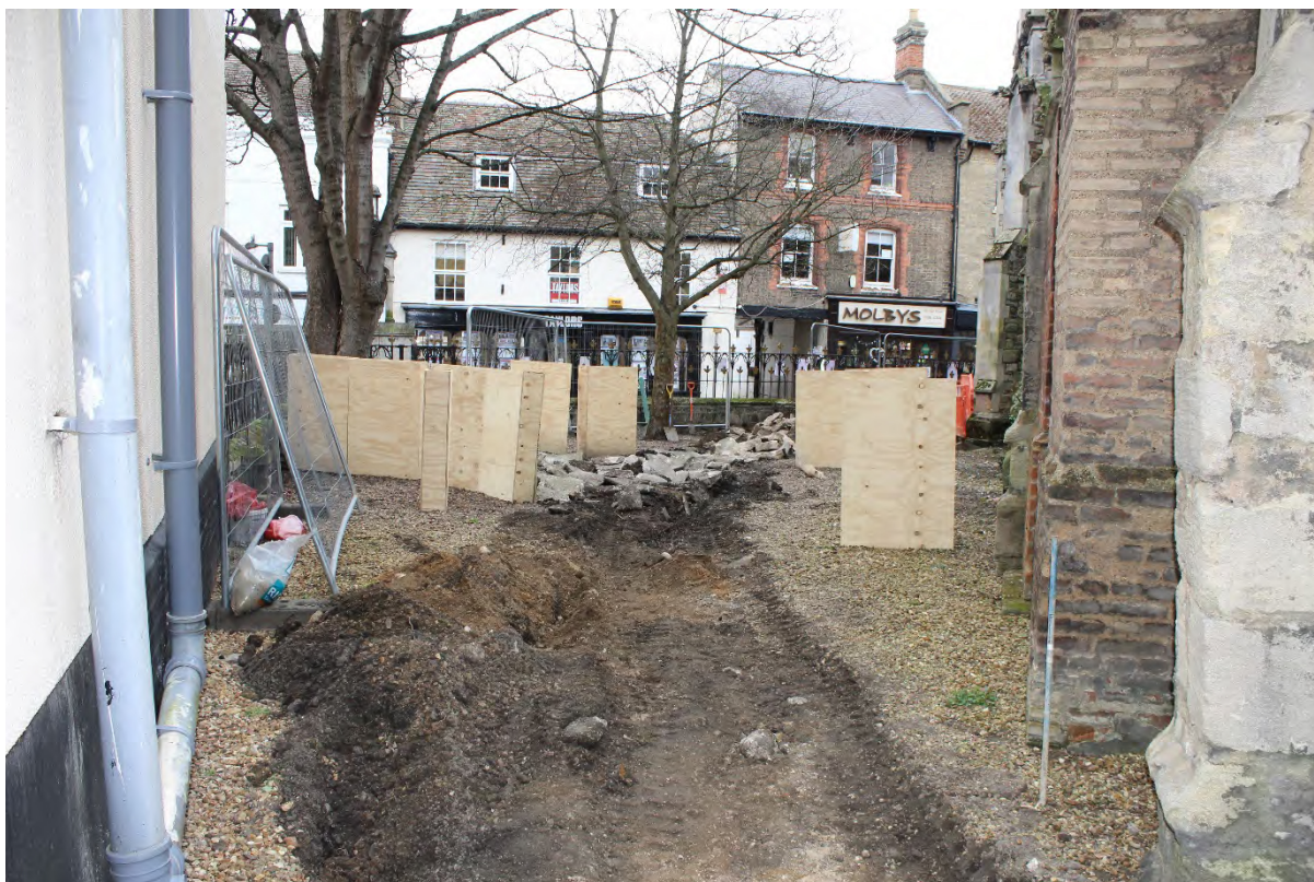
Plate 1: The site after removal of the concrete path, view north-east
