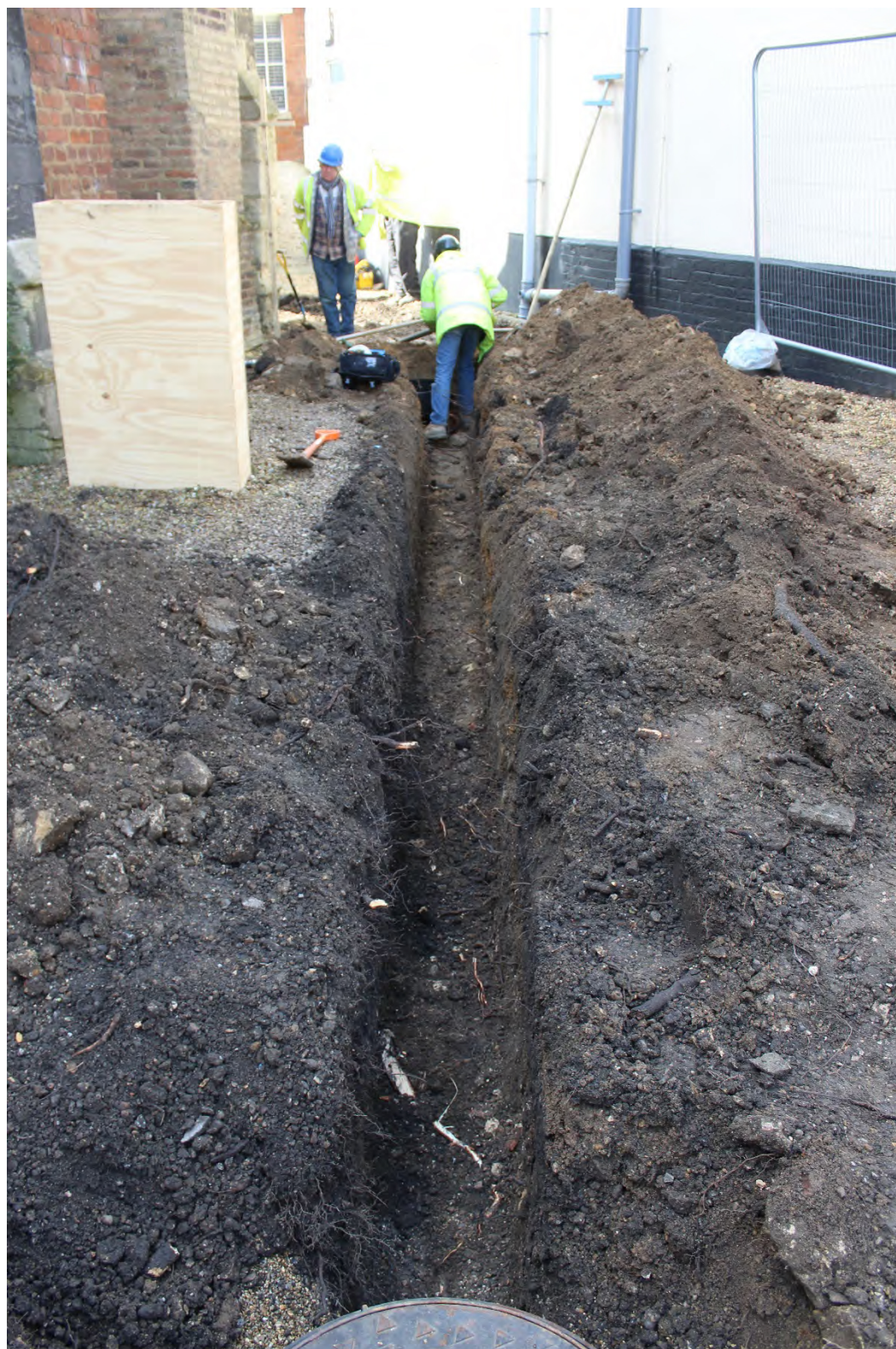
Plate 3: Drain trench, view south-west
