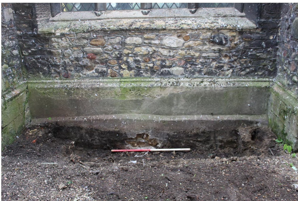
Plate 5: Ground reduction between buttresses on northern elevation, view south-east
