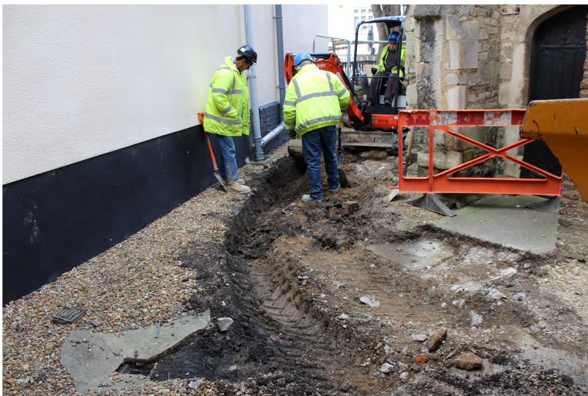
Plate 2: Excavation of the trench, view north
