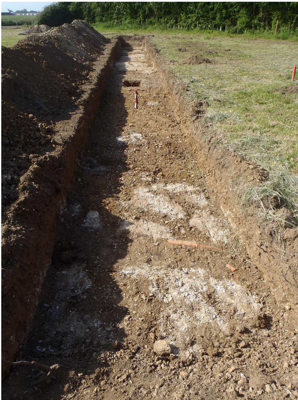
Plate 3 South facing view of Trench 5 (ditch [012] shown)
