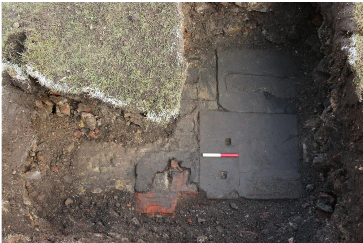
Plate 3: Tr 1B: Showing SW corner of Victorian guardhouse, looking north
