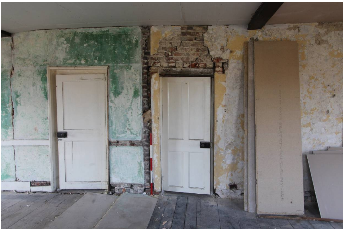
Plate 26 Removed partition wall between FF1 (left) and FF2 (right), looking south-west
