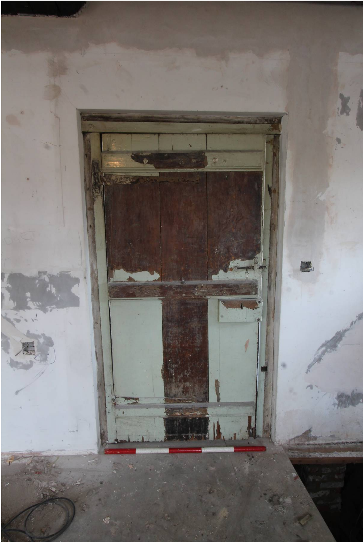
Plate 24 Plank door to GF3, looking south-west
