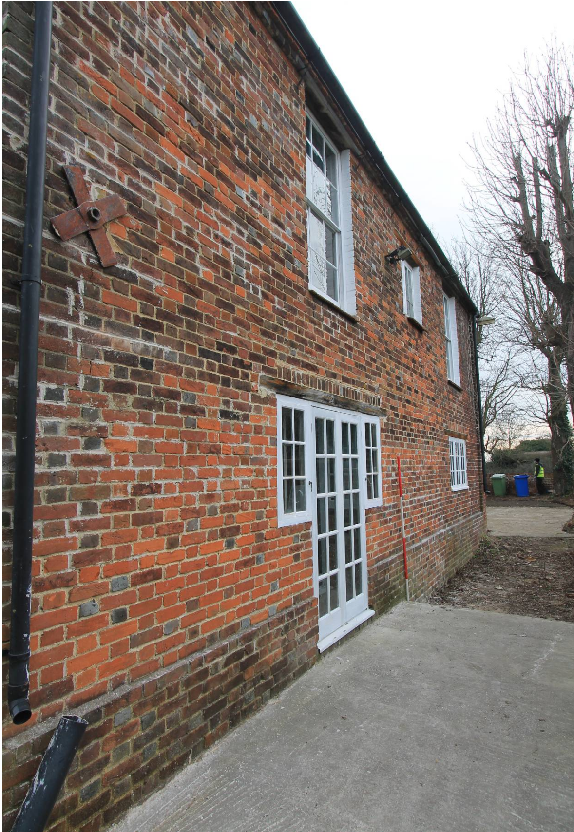
Plate 9 South-west elevation looking south-east
