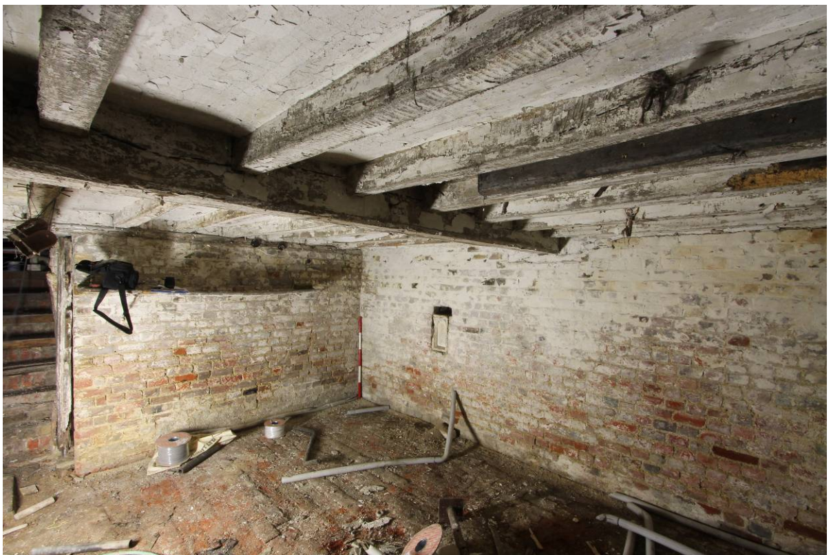
Plate 47 Basement looking east
