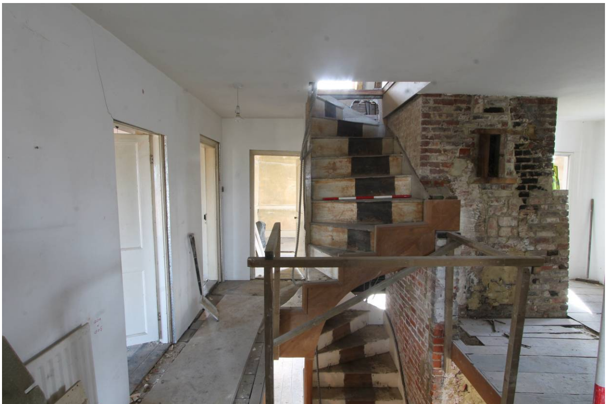
Plate 32 Former Bedroom FF4 looking south-east towards the staircase
