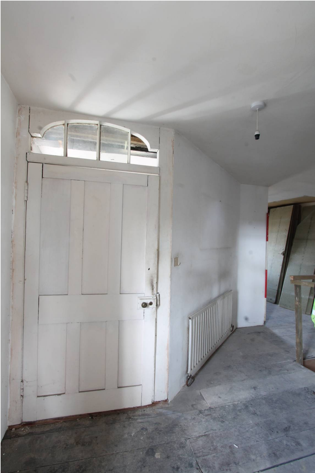
Plate 36 Former Bathroom FF5, looking north-west from FF4
