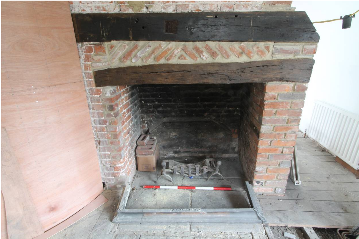
Plate 12 Open hearth fireplace in GF1 showing rebuilding, looking south-east
