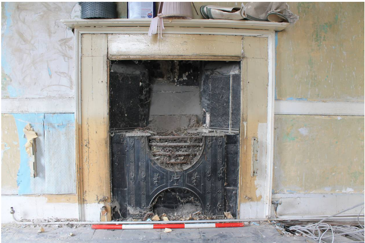
Plate 30 Fireplace in Bedroom FF3, looking north-west
