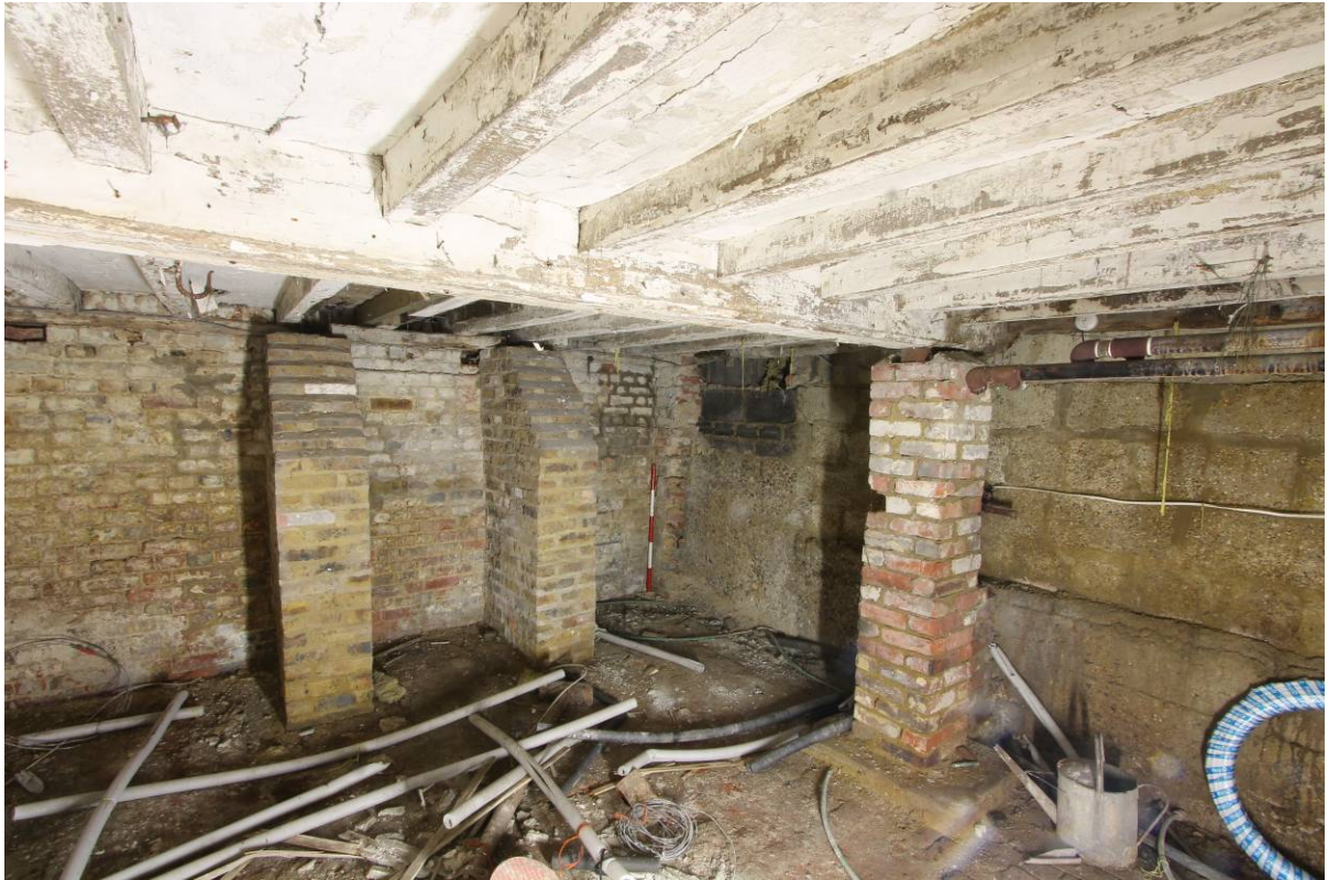
Plate 46 Basement looking west
