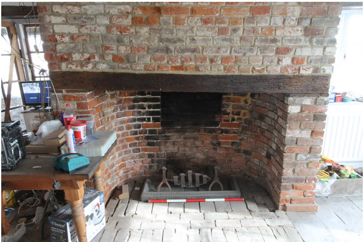
Plate 21 Inglebrook fireplace in GF4 showing rebuilt south-east side, looking north-east
