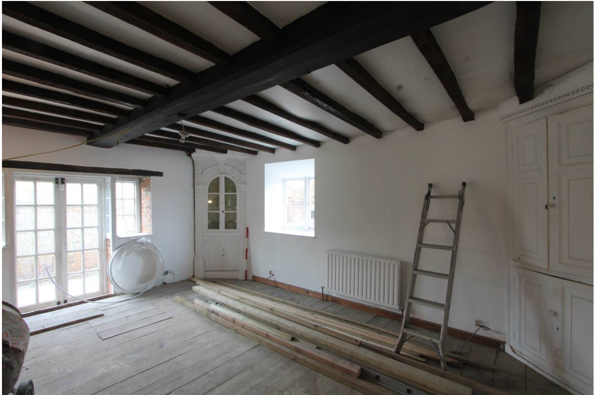
Plate 10 Room GF1 showing display cupboards, looking west
