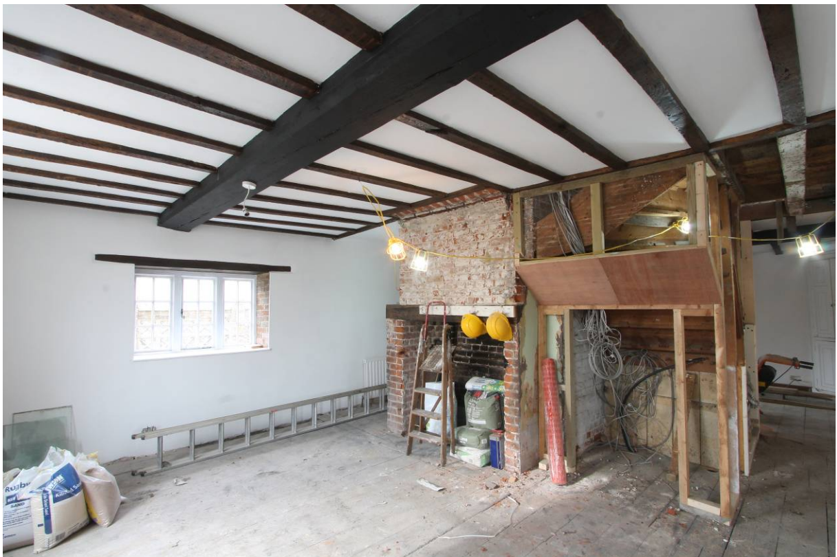
Plate 15 Room GF2 looking west
