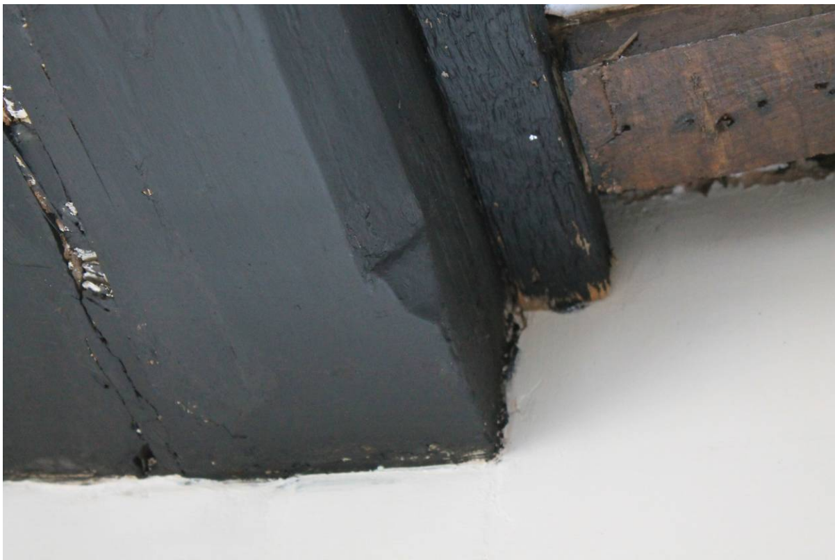
Plate 17 Chamfer and ogee stop to binding joist in GF2, looking south
