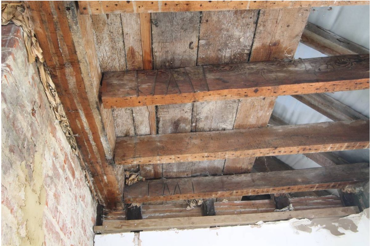
Plate 34 Heavy ceiling joists with Baltic marks over Room FF4, looking south-east
