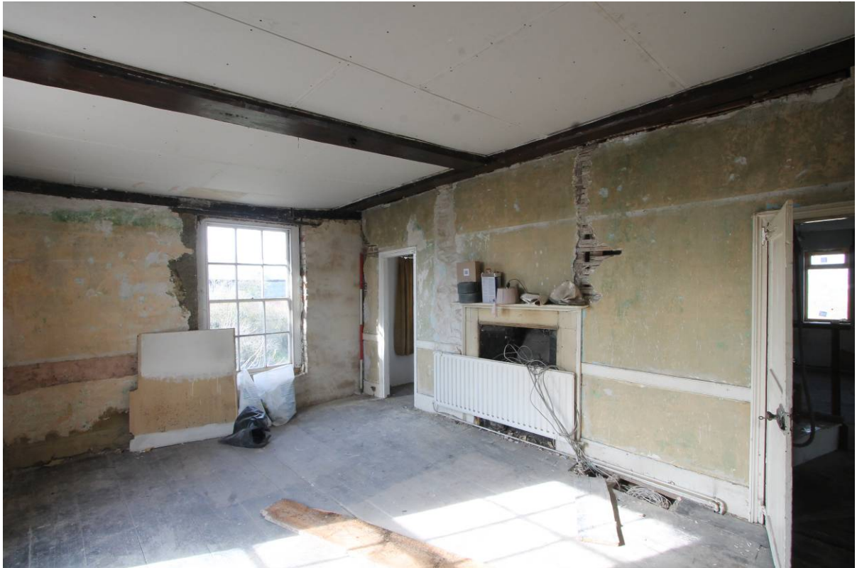
Plate 29 Bedroom FF3, looking west (before the removal of the radiator)
