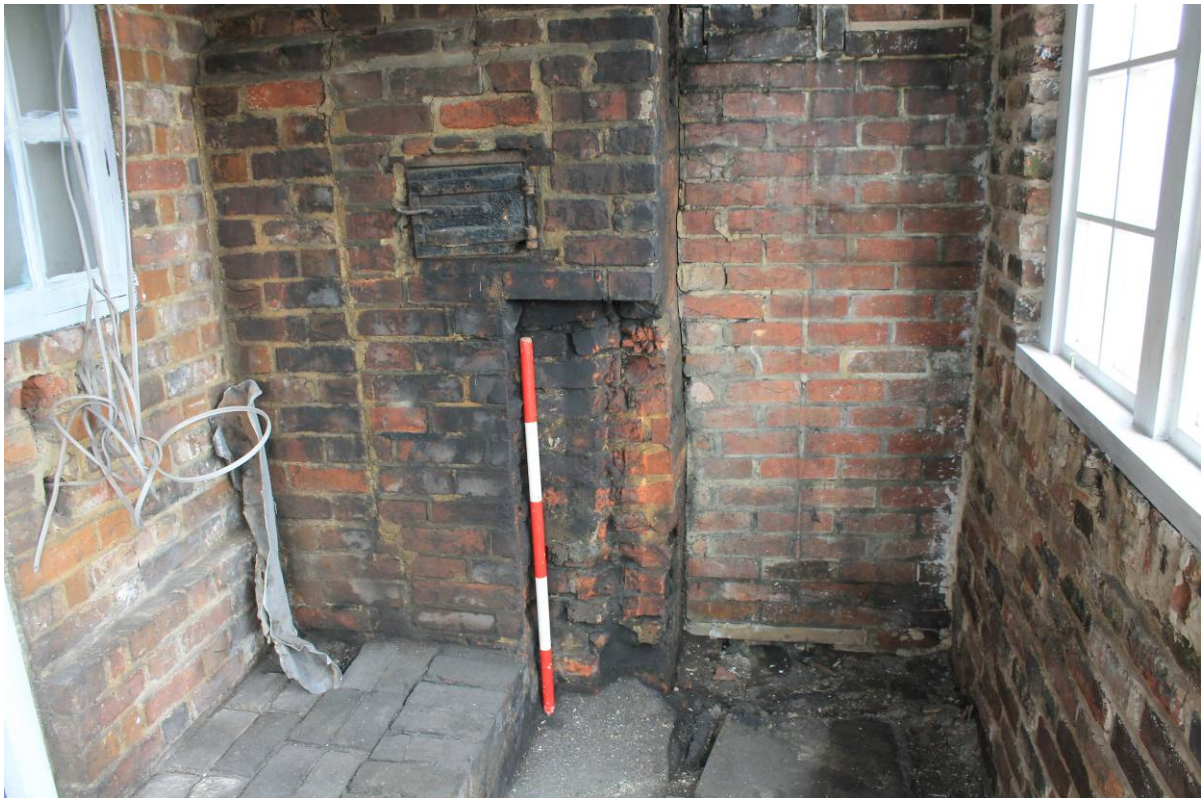
Plate 5 Flue for boiler in northern porch, looking north-west
