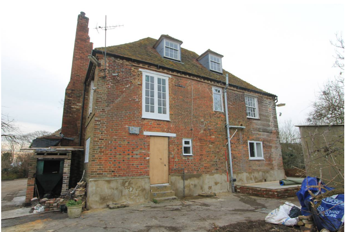
Plate 7 North-west (rear) elevation looking south-east
