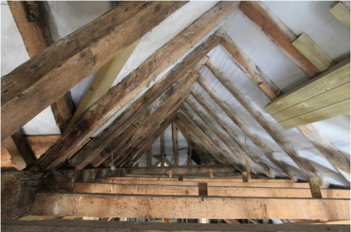
Plate 42 North-eastern roof pitch with central well to the left, looking north-west
