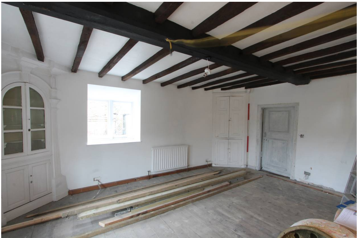
Plate 11 Room GF 1 showing display cupboards looking north
