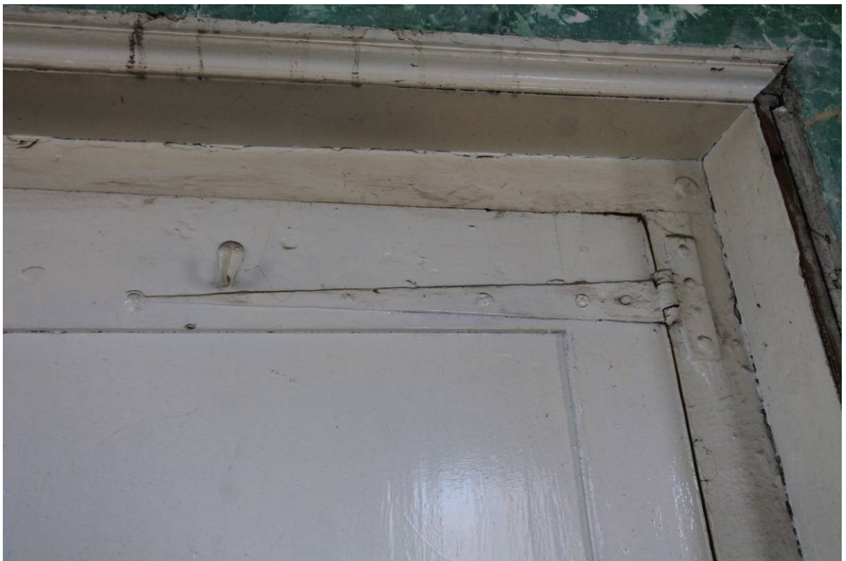
Plate 28 Eighteenth century strap (T) hinge on door to FF1, looking south-west
