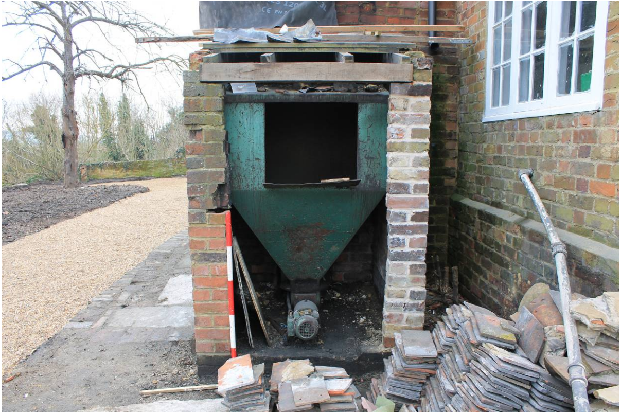
Plate 6 Coal hopper, looking south-east
