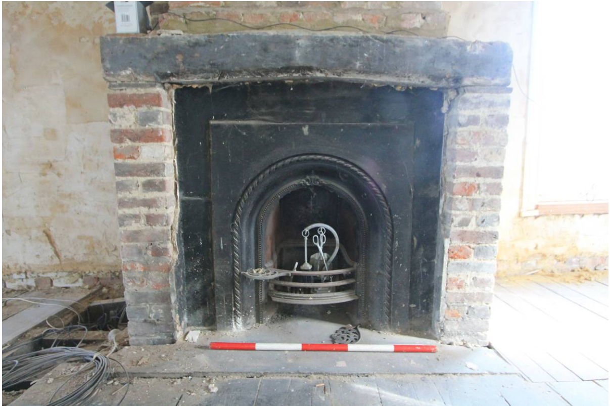
Plate 27 Inserted mid-late 19 th century cast-iron fire surround in Room FF1, looking north-east
