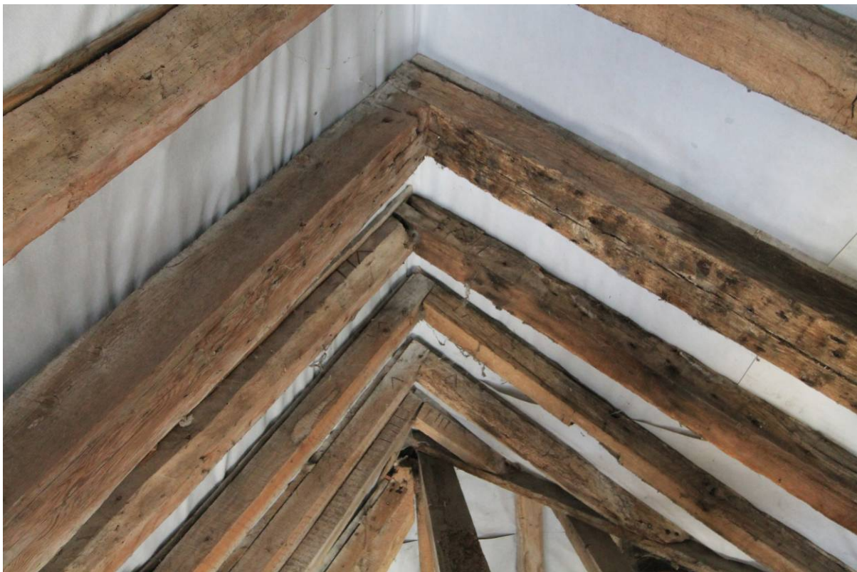
Plate 43 Roman marking to common rafters in south-eastern roof pitch with central well to the right, looking south-west
