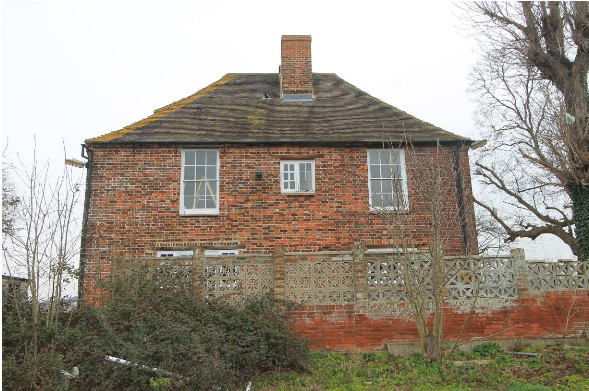
Plate 8 South-west elevation looking north-east
