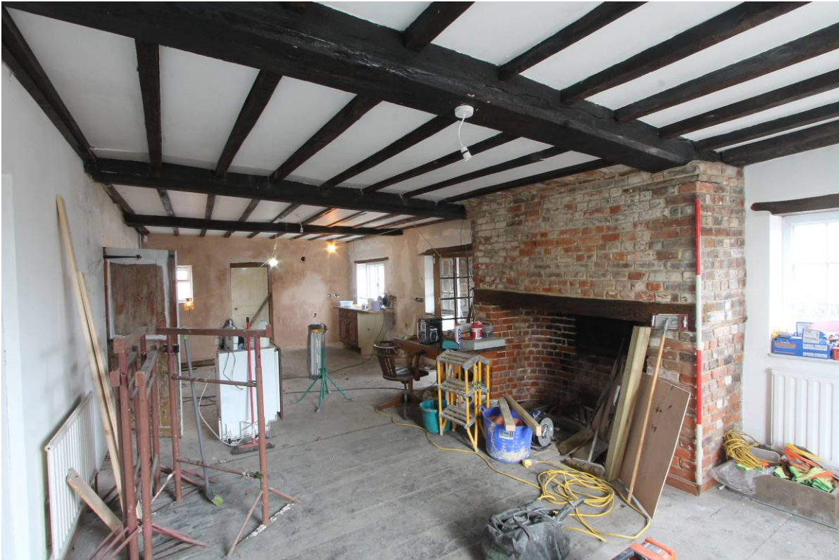
Plate 20 Rooms GF3 and GF4, looking north
