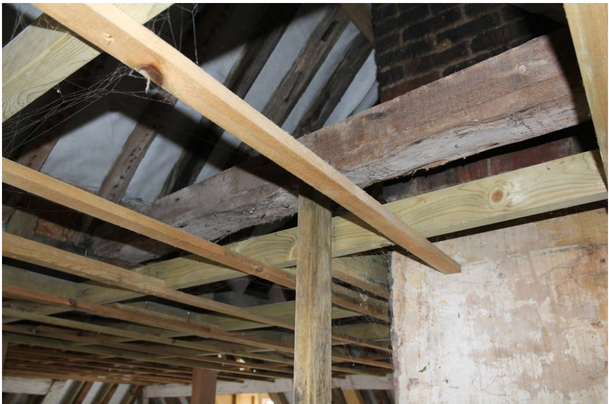
Plate 45 Timber conduit holding drainage pipe from central roof well, looking south-east
