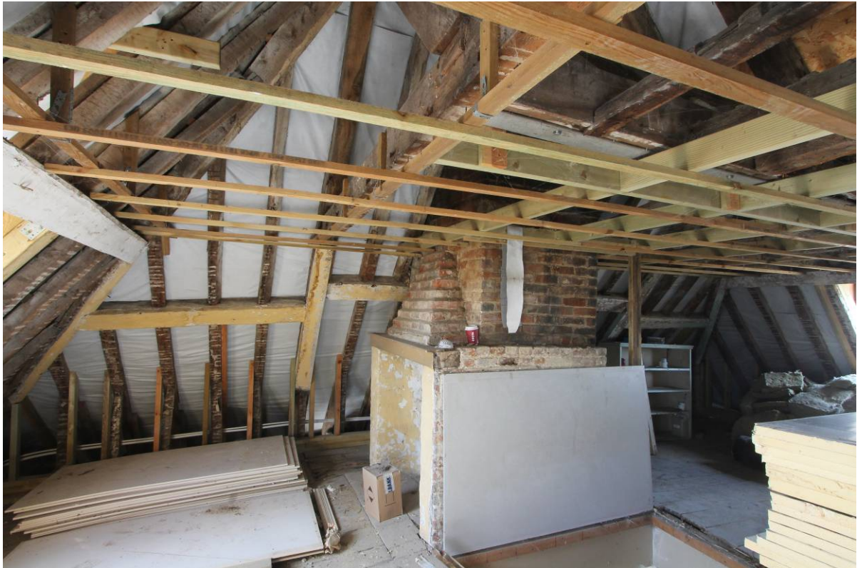
Plate 39 Attic floor showing fireplace and joggled butt purlins, looking south-west
