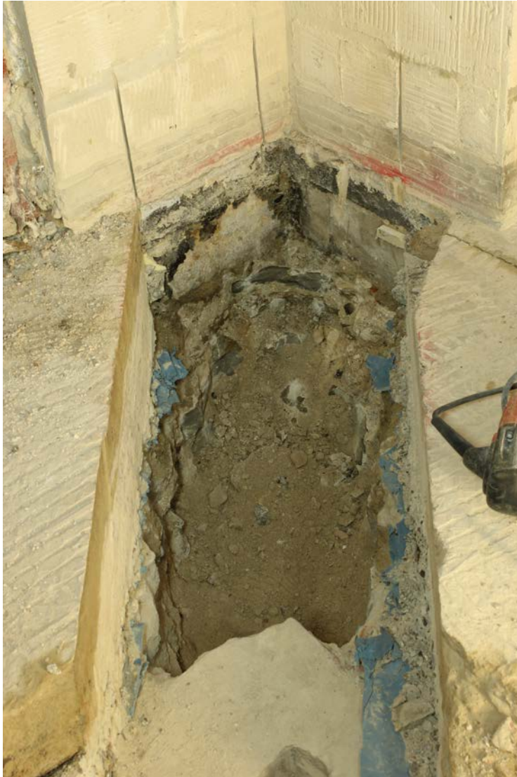
Plate 5: Trench 5 facing northeast
