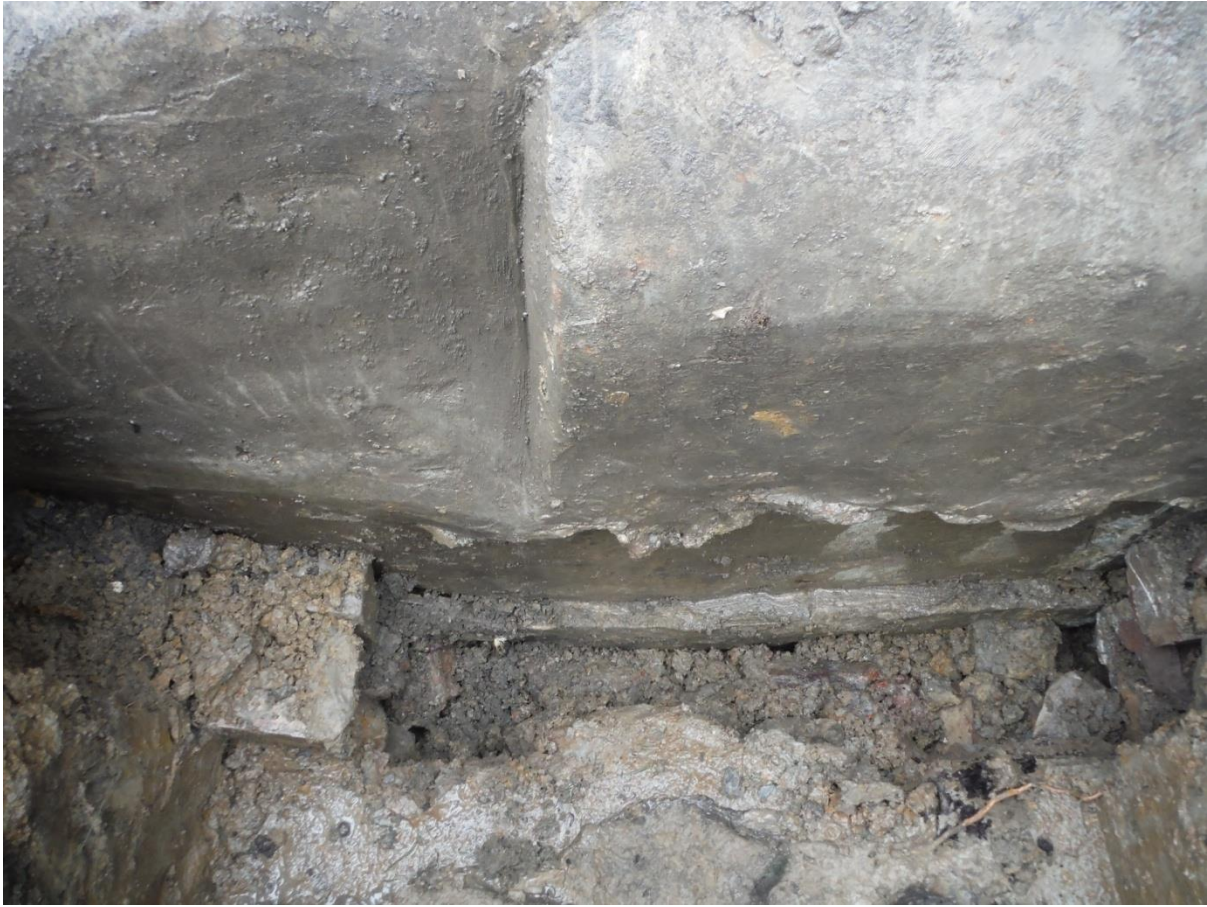
Plate 6: South view of exposed screen wall in sondage (no scale)
