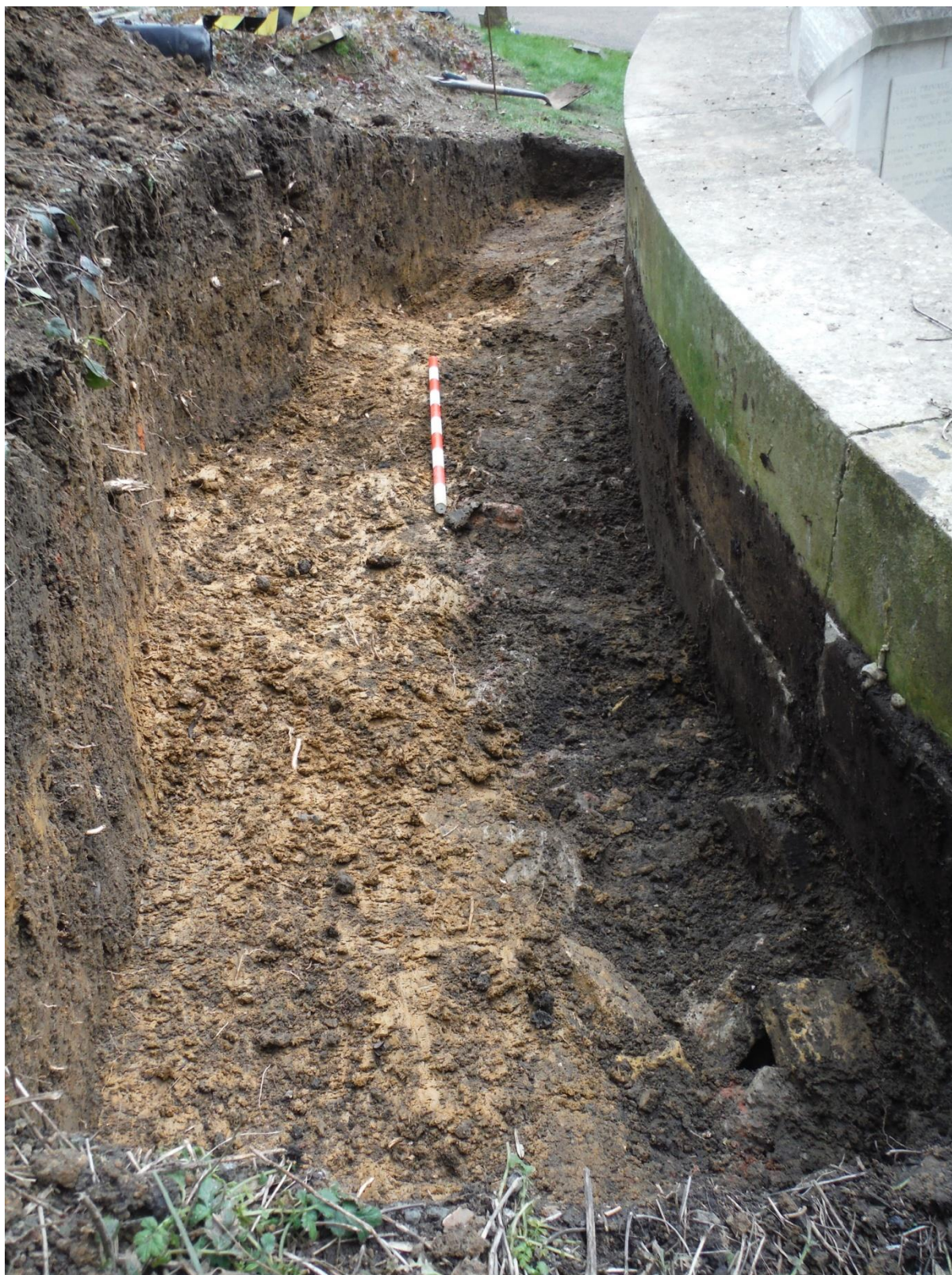
Plate 2: East view of test trench (1m scale)
