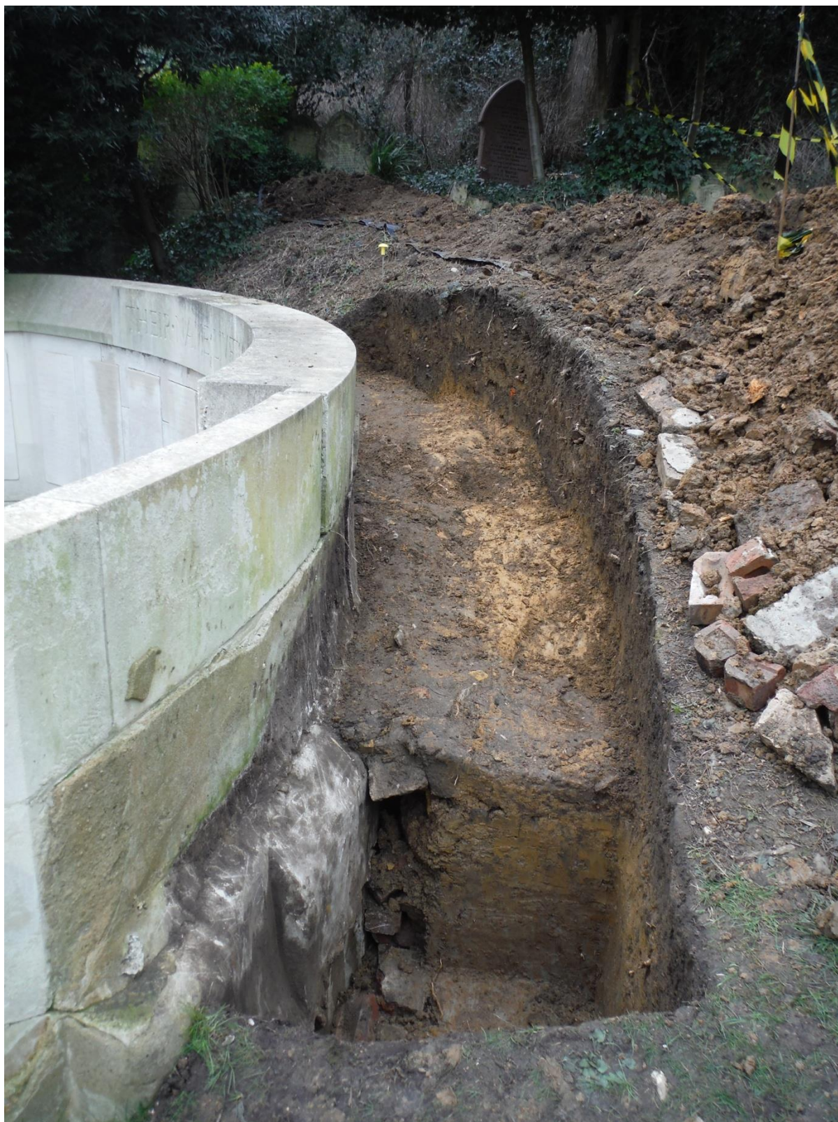
Plate 3: West view of test trench (no scale)
