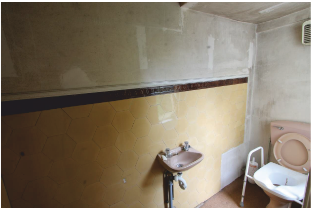
Plate 49 WC (FF7), looking north-west
