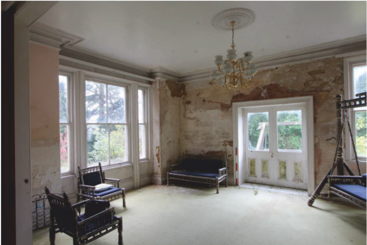
Plate 23 Double Drawing Room (GF2), looking south-east
