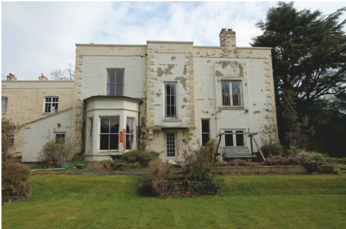
Plate 9 Southern elevation, looking north
