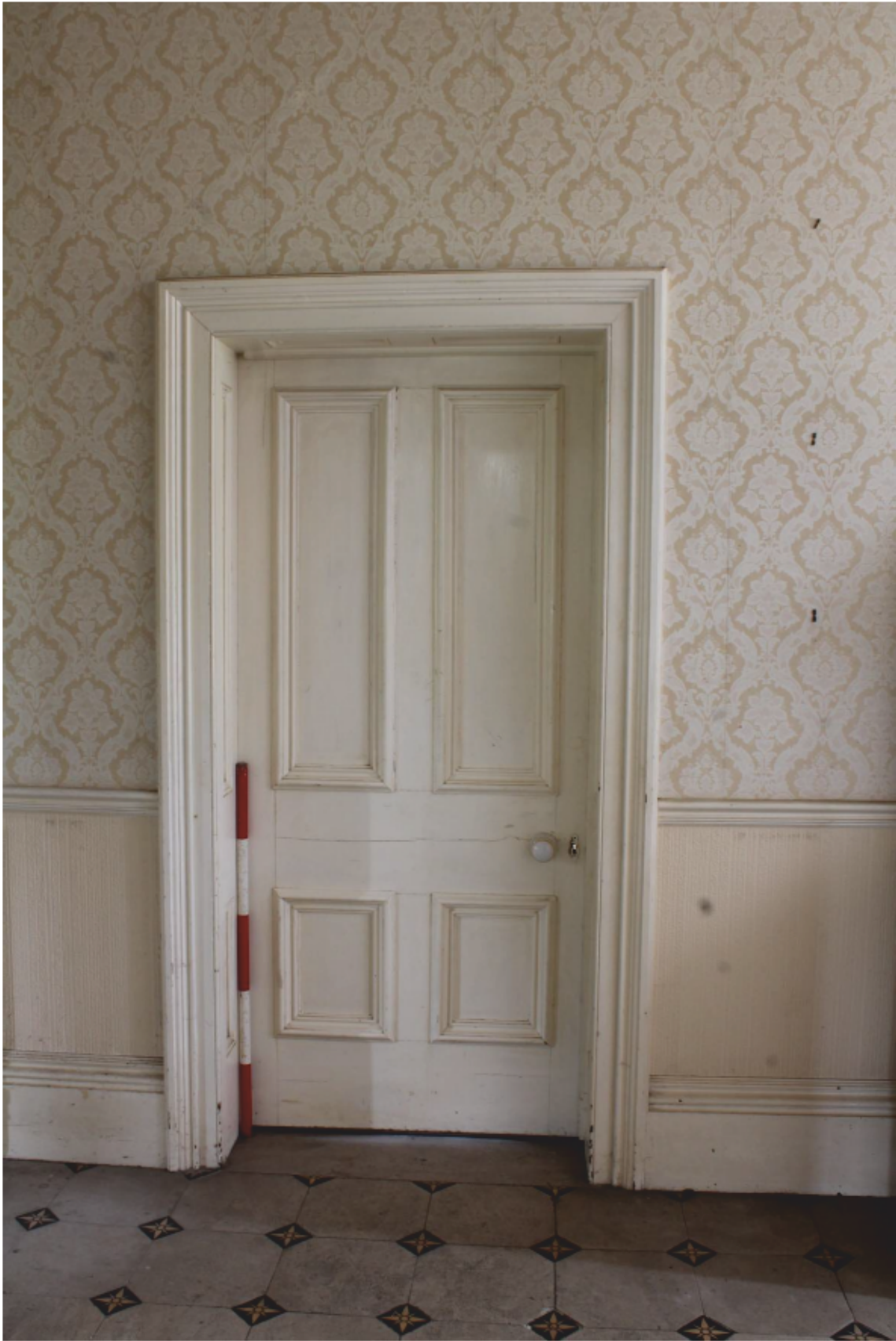
Plate 19 Typical door and architrave from Hall (GF1) into (GF3), looking east
