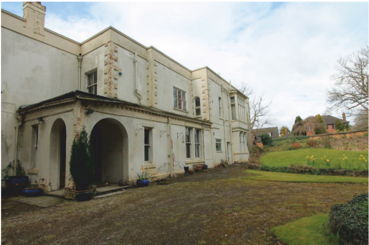
Plate 2 North elevation, looking south-west
