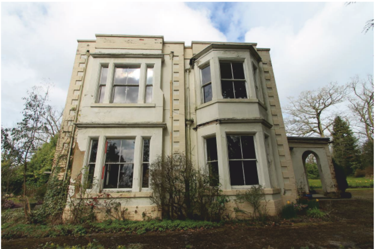
Plate 14 Eastern End Elevation, looking west
