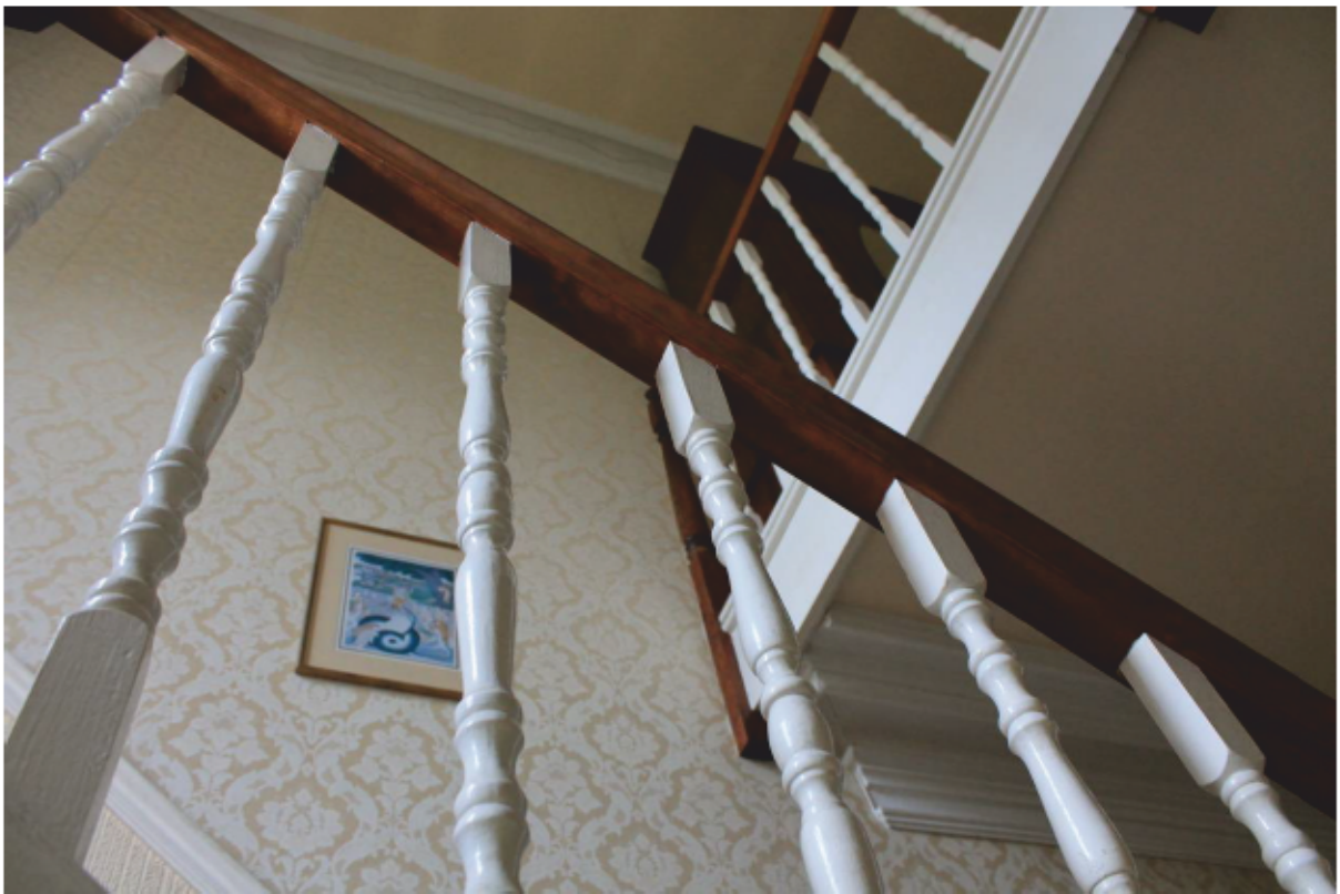
Plate 18 Detail of Balustrade in (GF1), looking west
