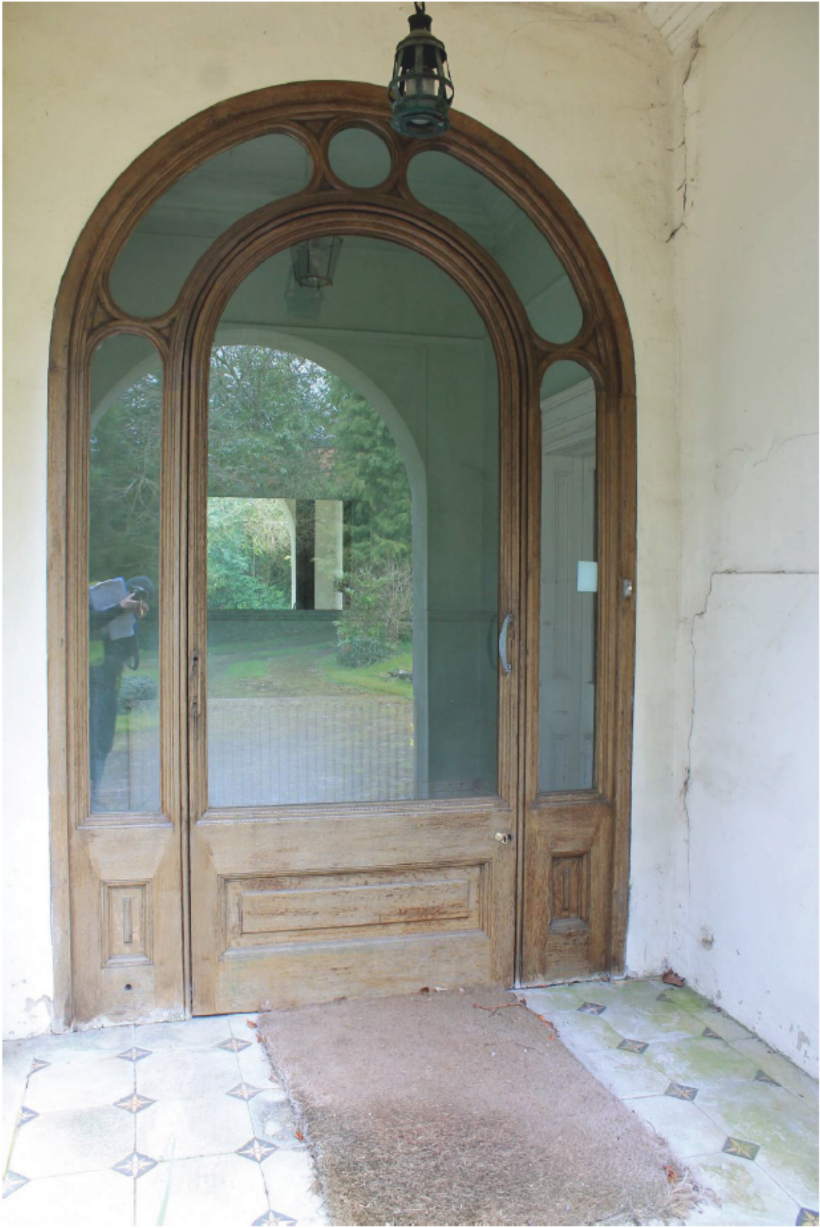
Plate 7 Art Nouveau style glazed entrance to outer hall, looking south
