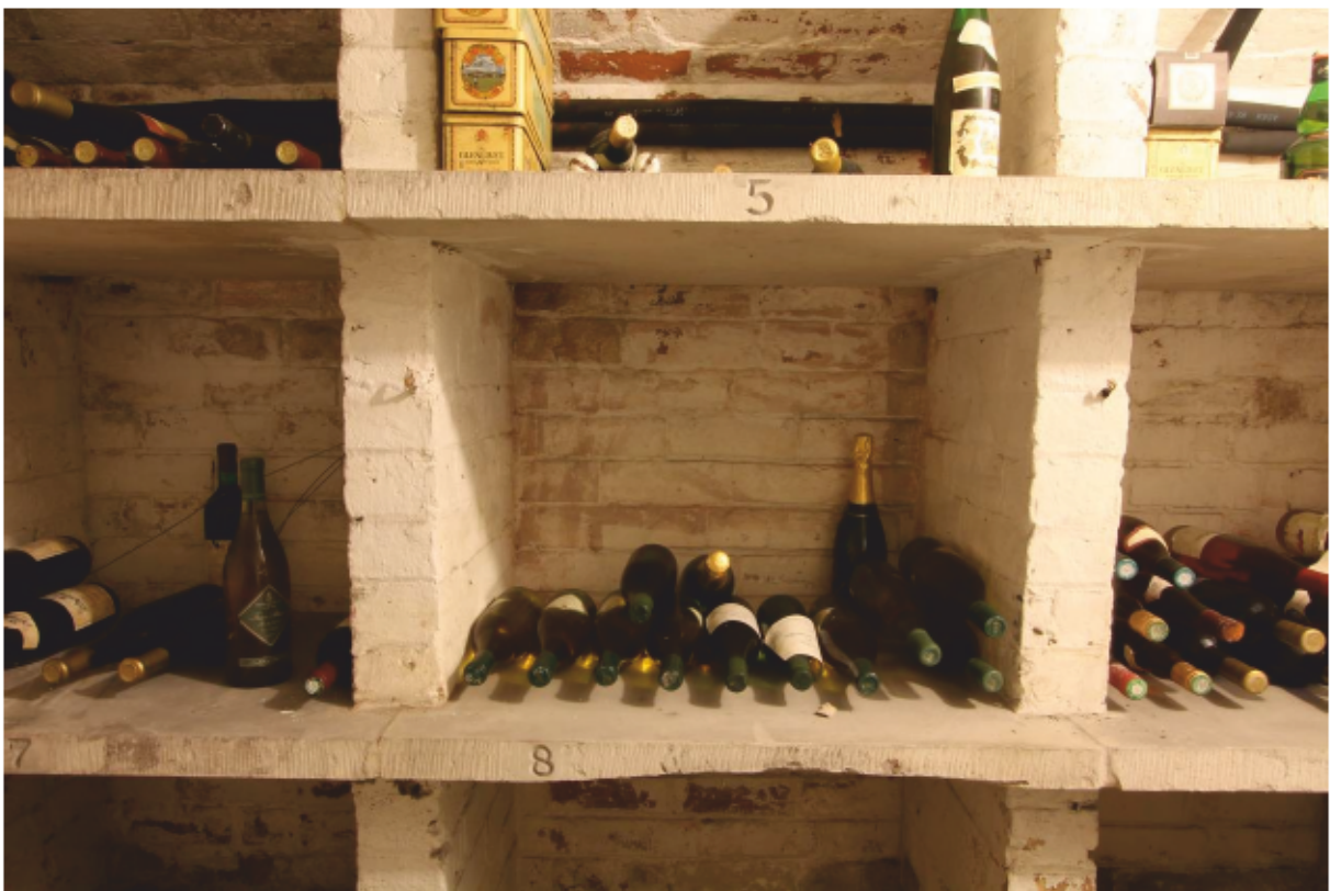
Plate 59 Detail of bins in wine cellar (B4), looking east
