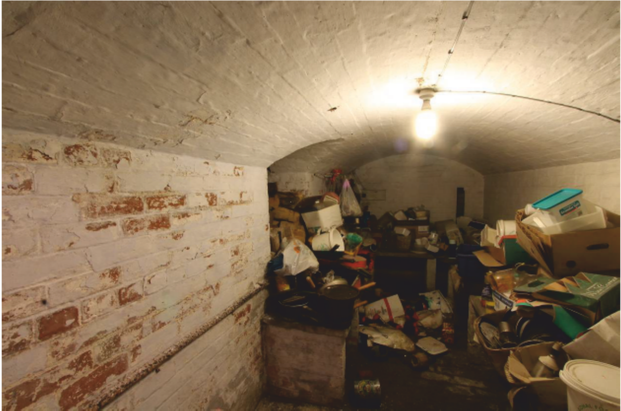
Plate 56 Cellar vault (B2), looking east
