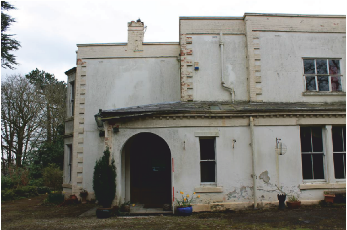
Plate 3 Eastern part of the north elevation, looking south
