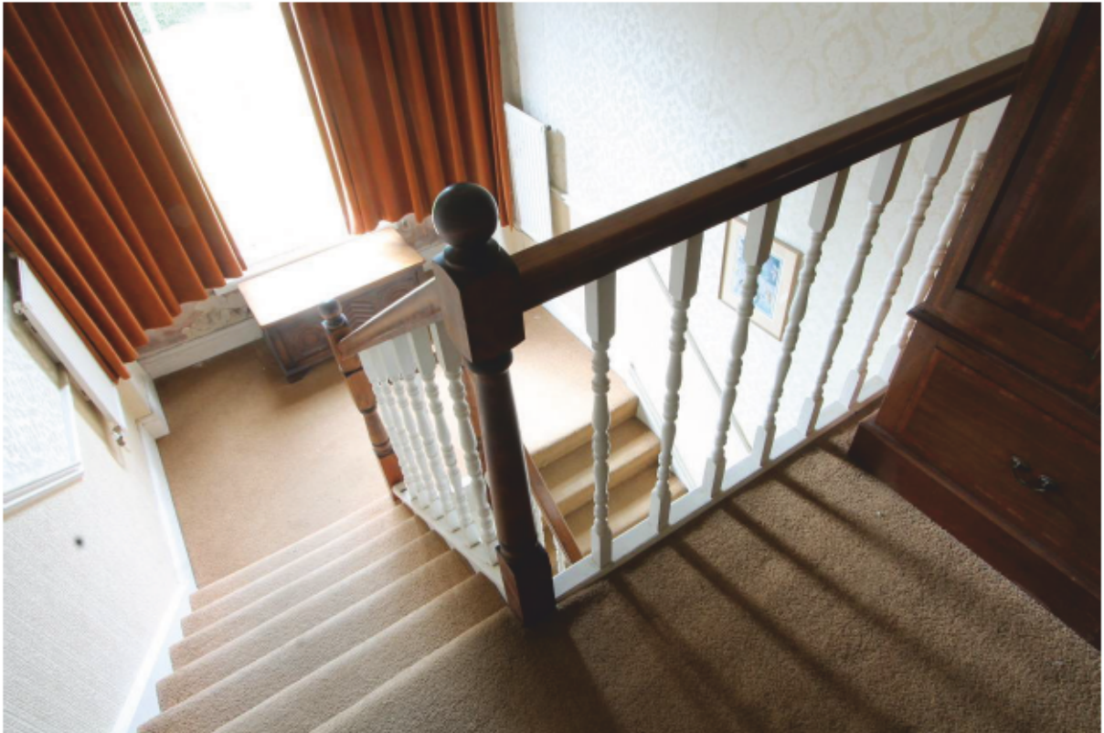
Plate 42 Open well stair
