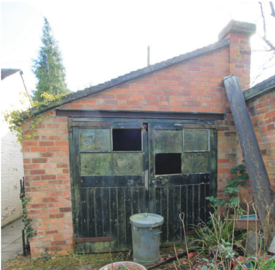
Plate 61 Garage, looking south-west
