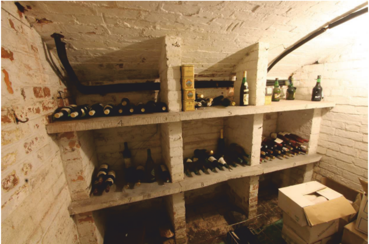
Plate 58 Wine cellar (B4), looking east
