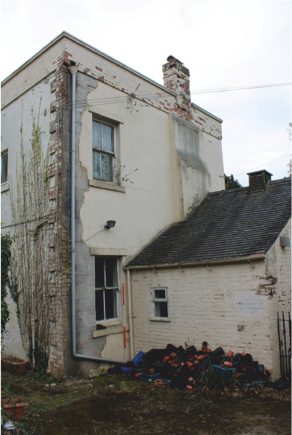
Plate 8 Western end elevation, looking south-east
