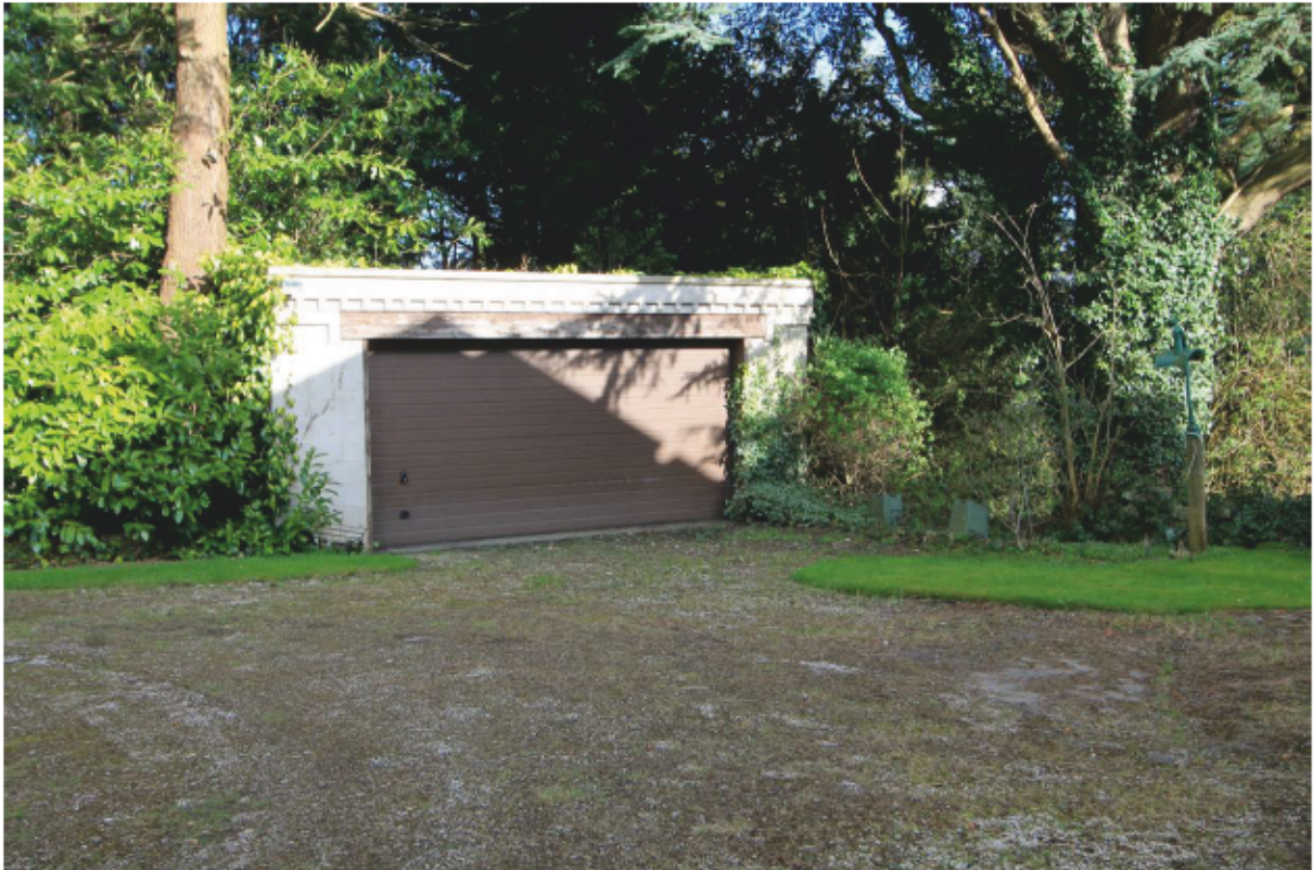
Plate 63 Modern blockwork double garage, looking west
