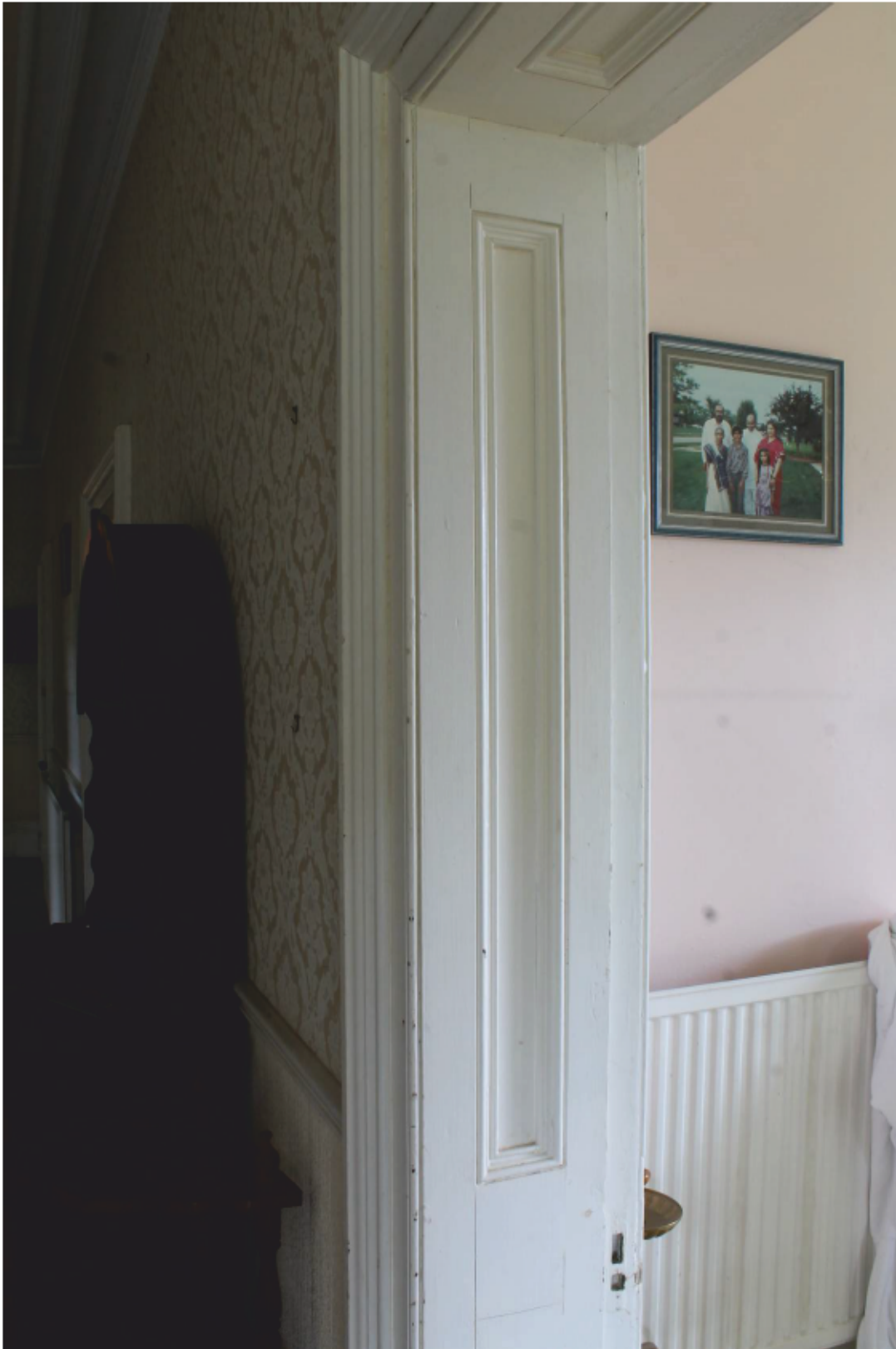
Plate 20 Typical panelled doorcase (to GF2), looking north-east
