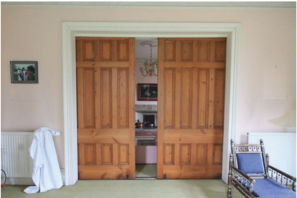
Plate 22 Double Drawing Room, showing internal sliding screen, looking north from (GF2) to (GF3)
