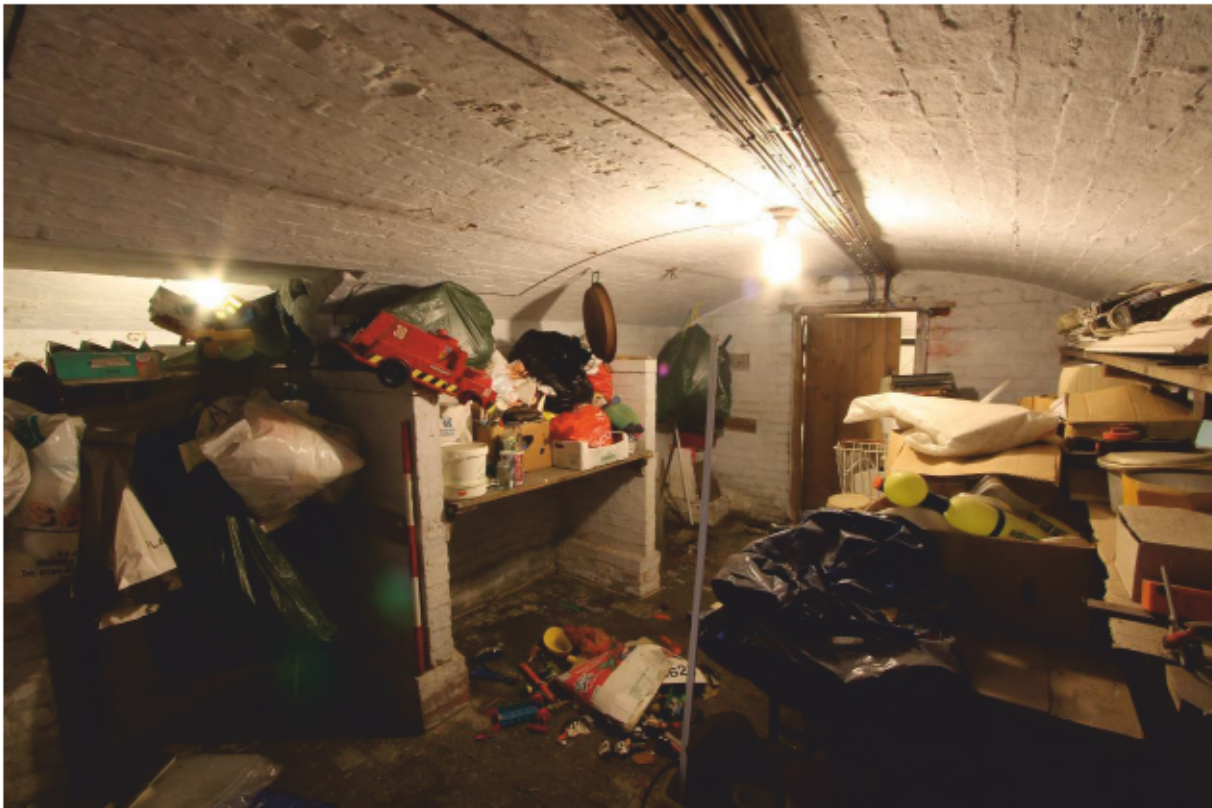
Plate 57 Cellar vault (B3), looking east
