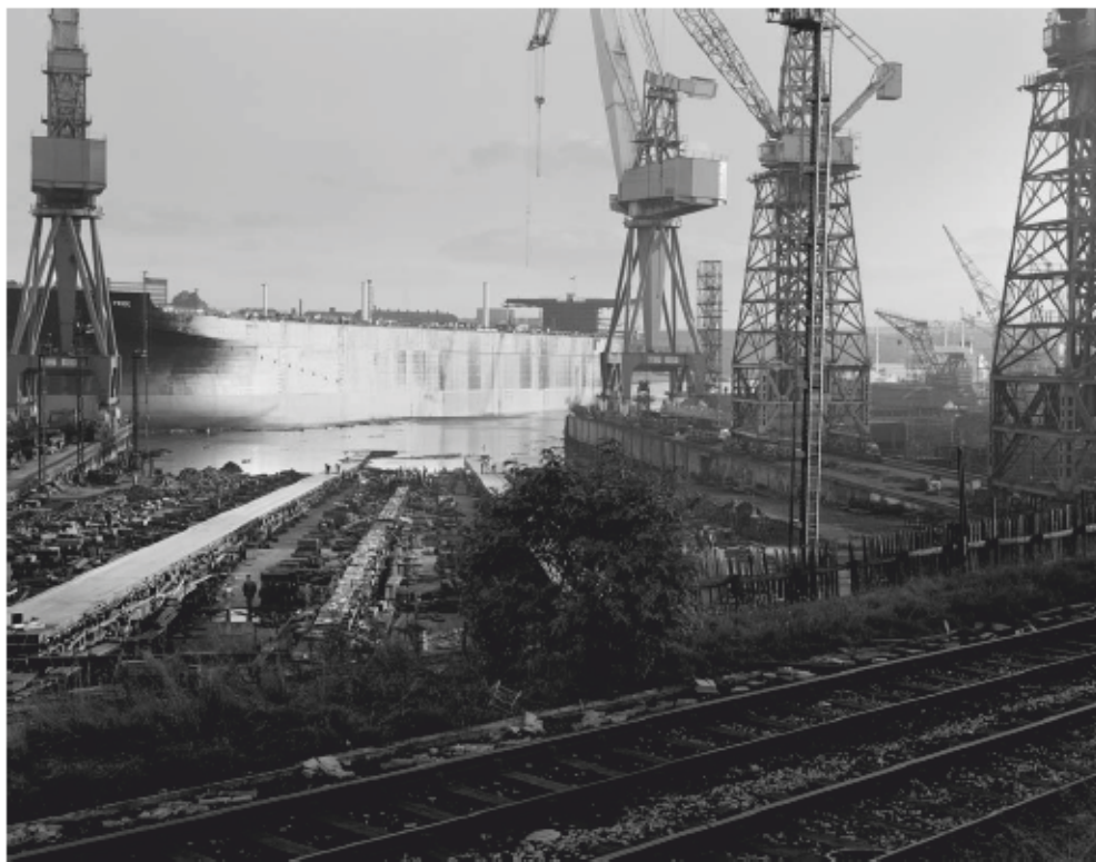
Plate F: Historic photograph showing cranes at Swan Hunter shipyard
