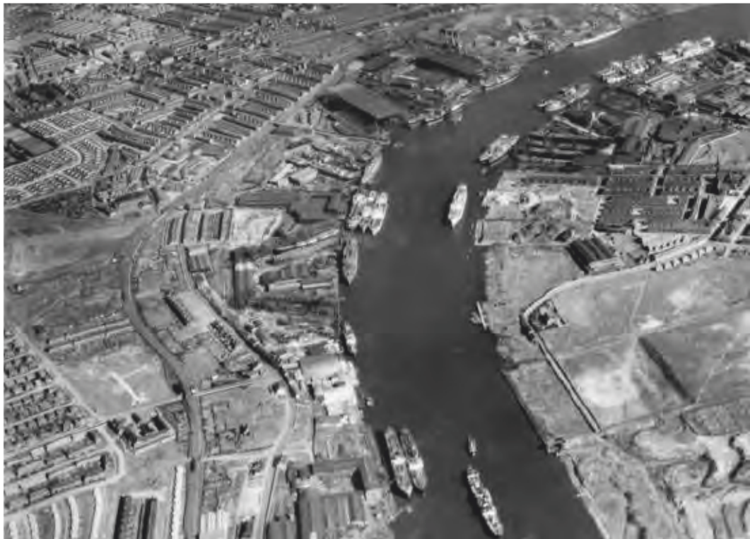
Plate B: Historic photograph of shipyards in Wallsend, 1947
