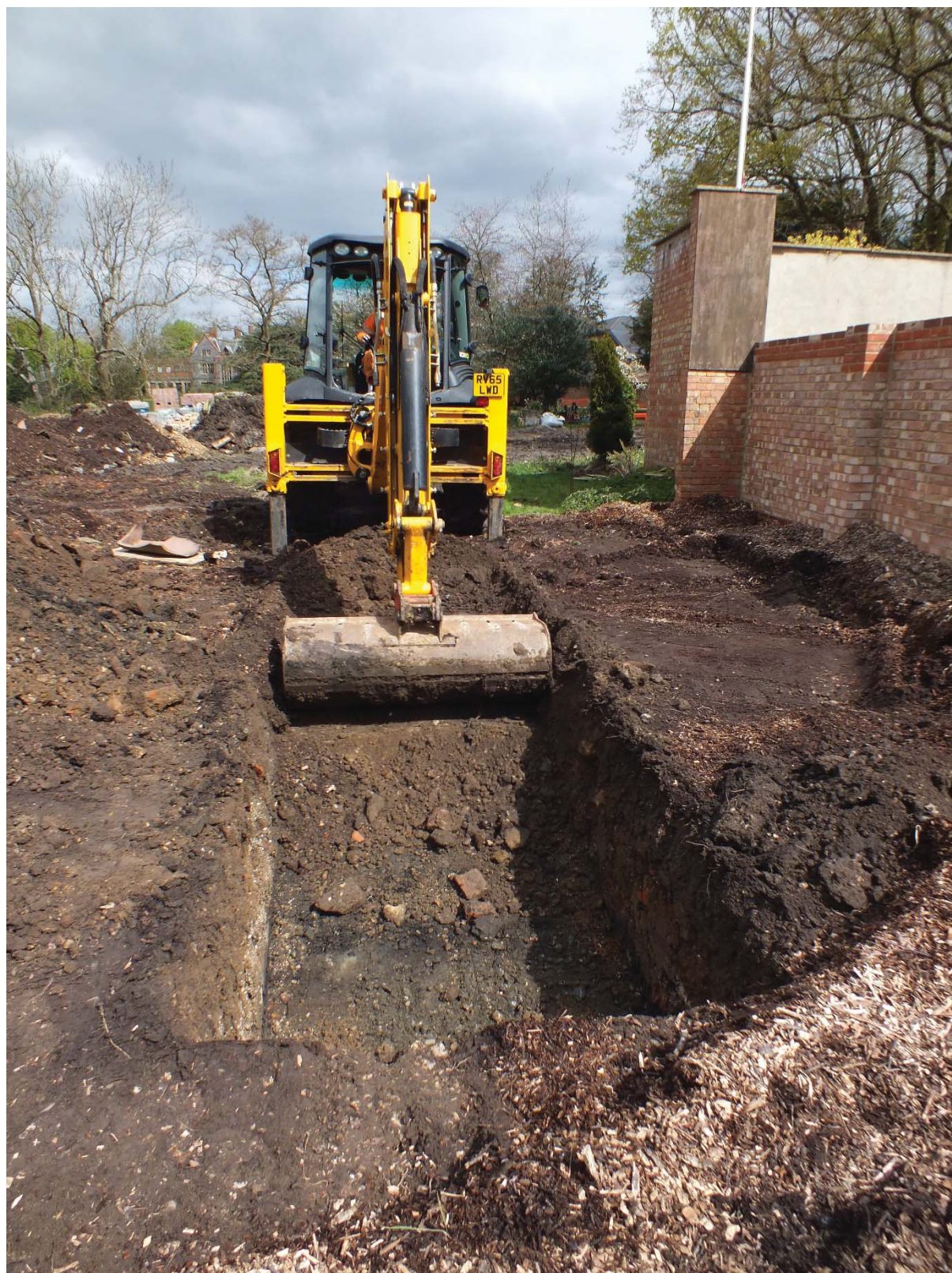
Plate 7: Trench 4 mid excavation, looking northeast (BRBS15 D3 016)
