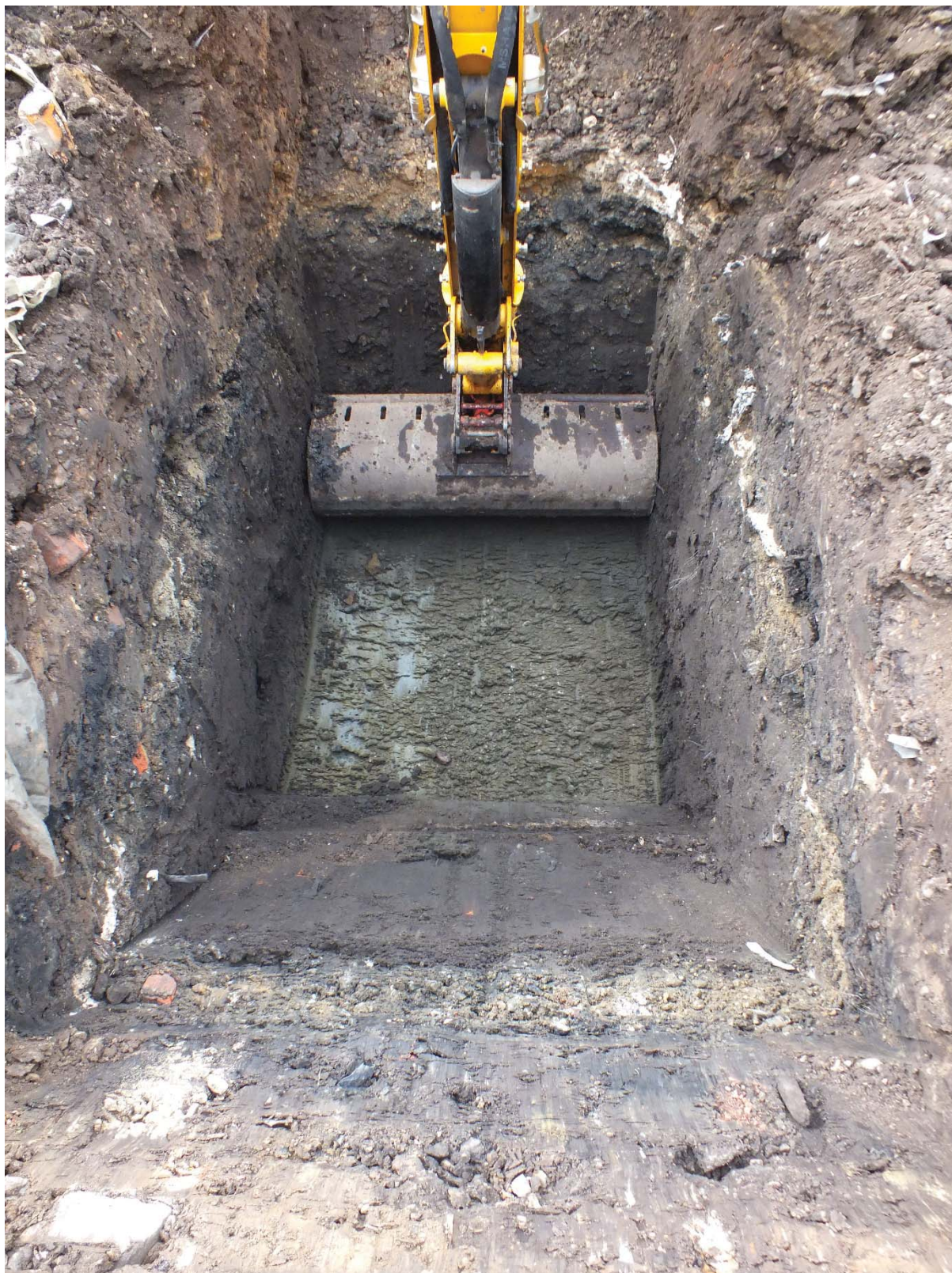
Plate 9: Overview of Trial Pit 2B, looking southwest (BRBS15 D3 052)
