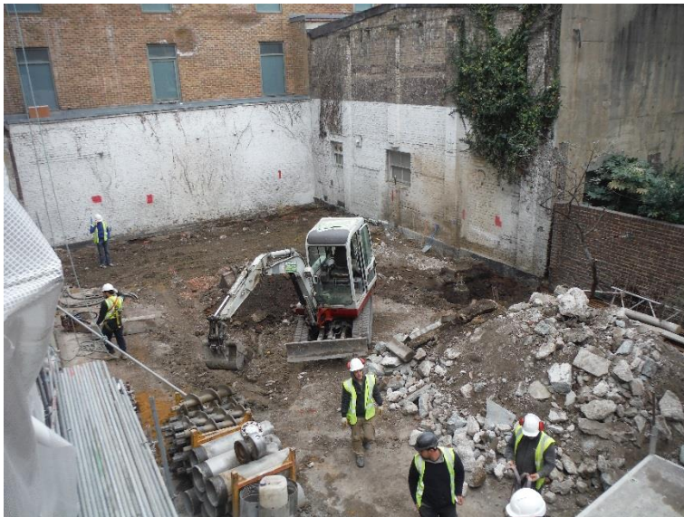
Plate 6: View north-west, general site arrangement
