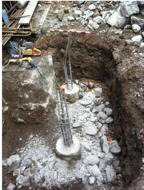
Plate 4: Pile-cap 1, view east
