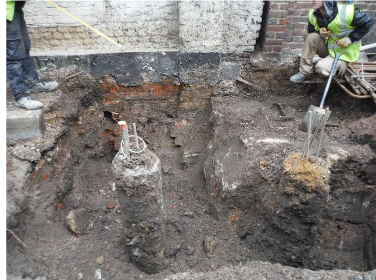
Plate 7: Pile-cap 2, view north
