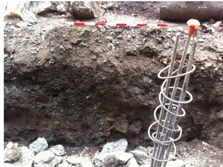
Plate 8: Pile-cap 3, view north
