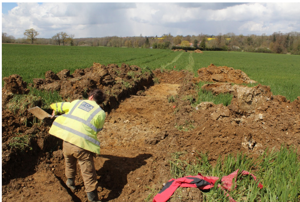
Plate 1: Pipeline route from Trench 16, view north-west.
