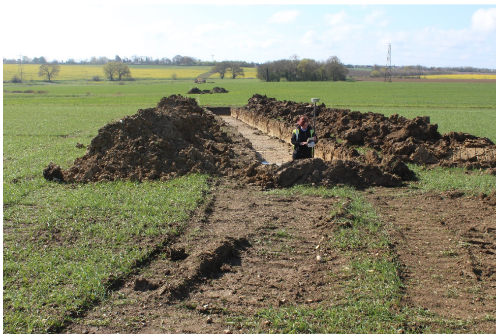
Plate 4: Pipeline route, view south-east.
