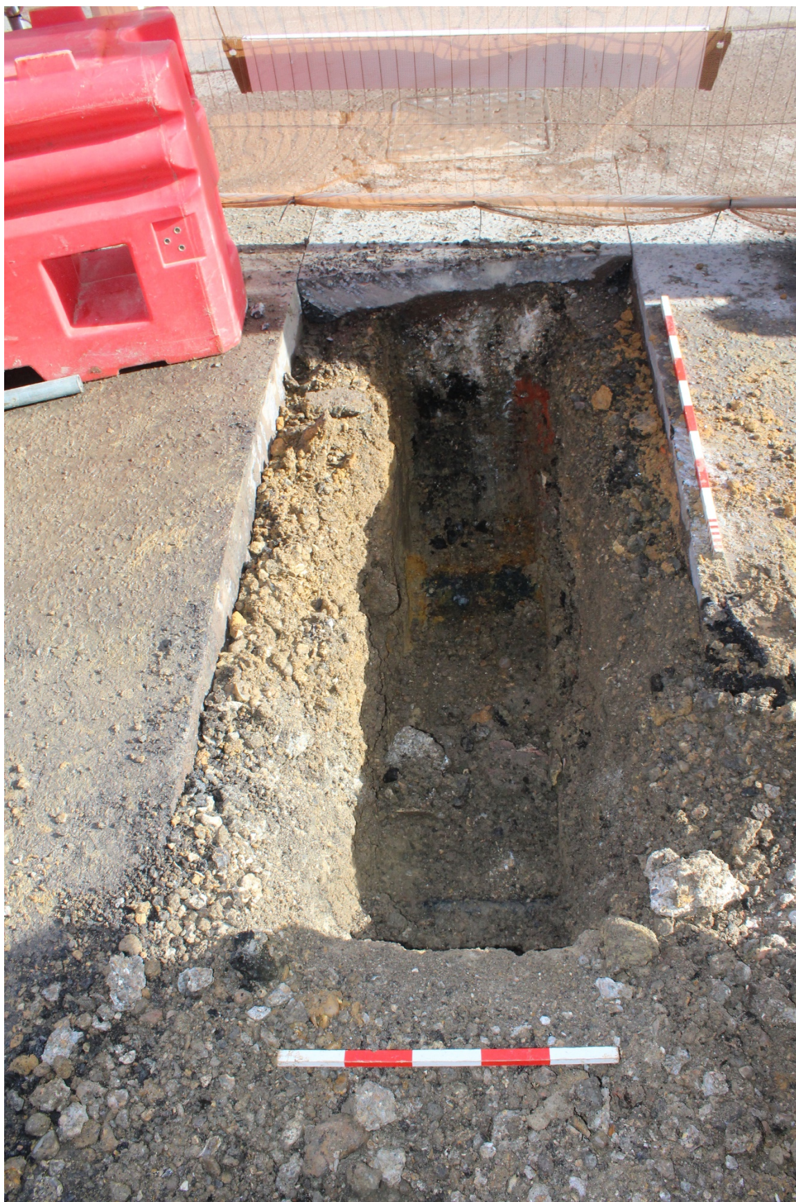
Plate 5 East facing view of monitored excavation (2016)
