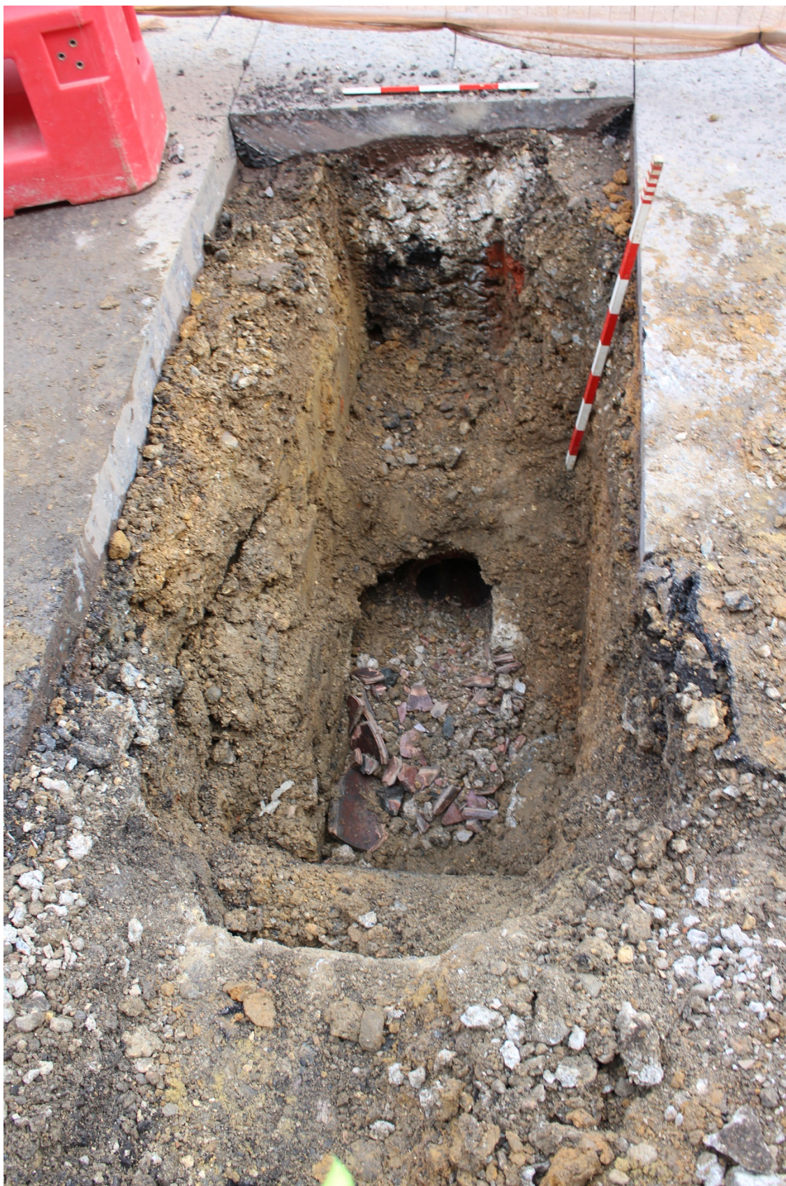
Plate 6 East facing view of accessed storm drain, showing extensive ground disturbance.
