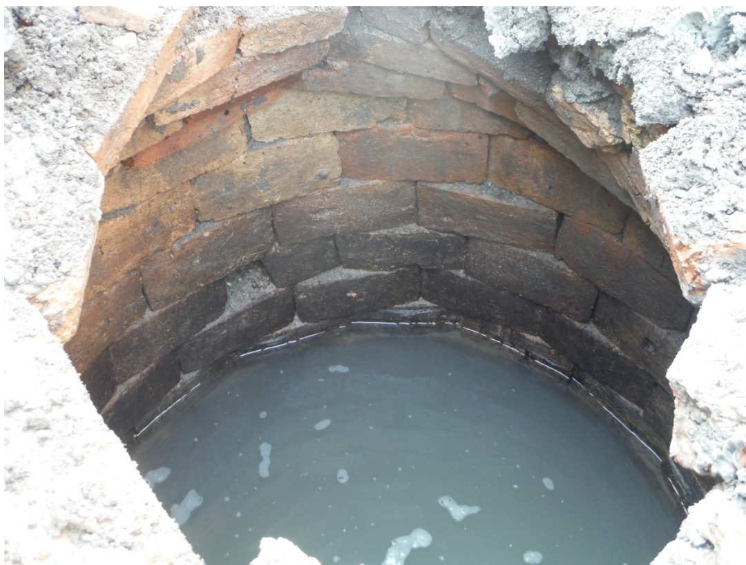
Plate 4: Well 103, internal view
