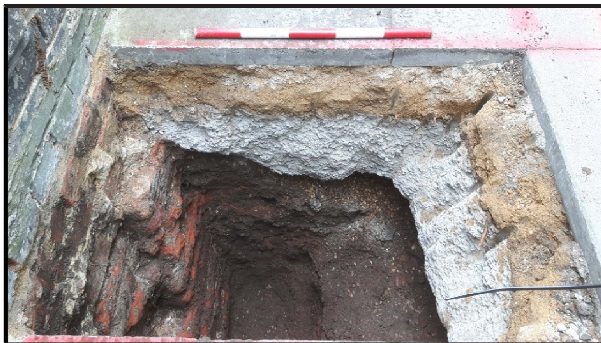
PLATE 11. SOUTHEAST FACING SECTION IN TP12 SHOWING WALL [13] TO THE LEFT OF THE IMAGE.
