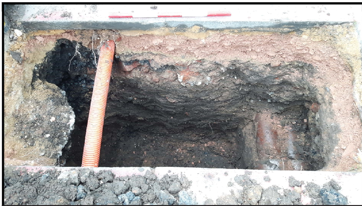
PLATE 7. SOUTH FACING SECTION OF TP8, SHOWING MODERN PIPING AND FEATURES TRUNCATING THE DARK BROWN VICTORIAN DUMP LAYERS WHICH EXTEND DOWN TO THE BASE OF THE TRENCH.
