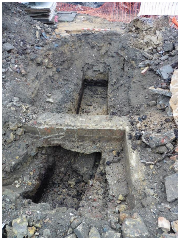
Plate 2: Trench 2 Looking South
