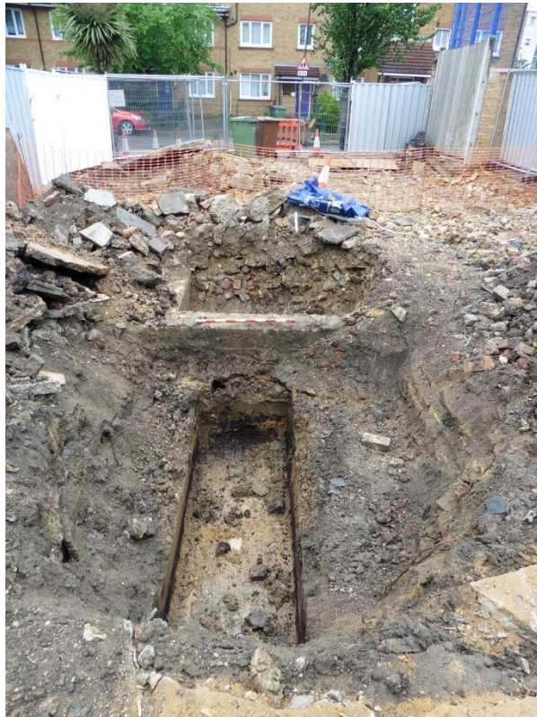
Plate 1: Trench 2 Looking North
