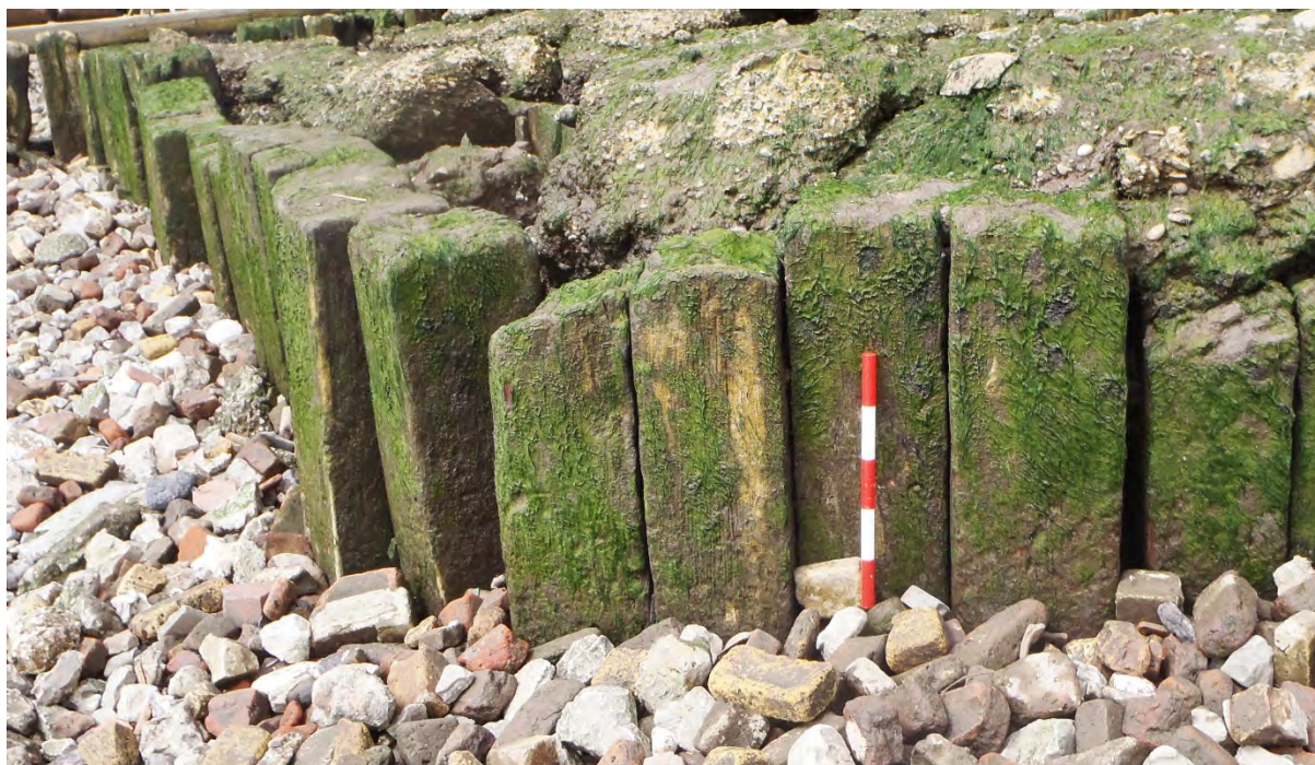
Plate 7: Post revetment [200]. View to north-west. Scale 0.5m
