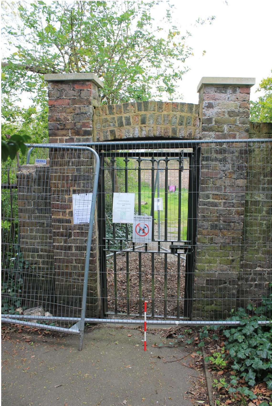
Plate 4 Gateway to churchyard looking west
