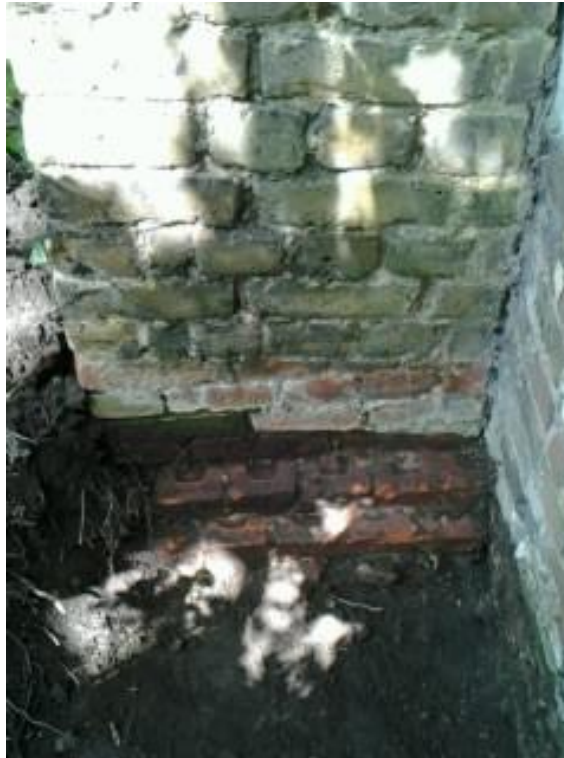
Plate 5: Footing [402] to later buttress [403] external to the Walled Garden
