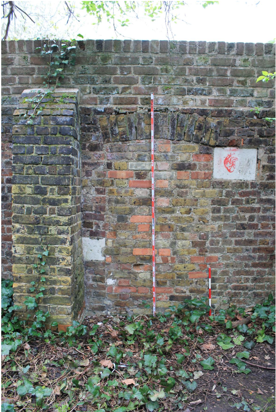
Plate 1 Blocked door opening in Southern Garden Wall (south side)
