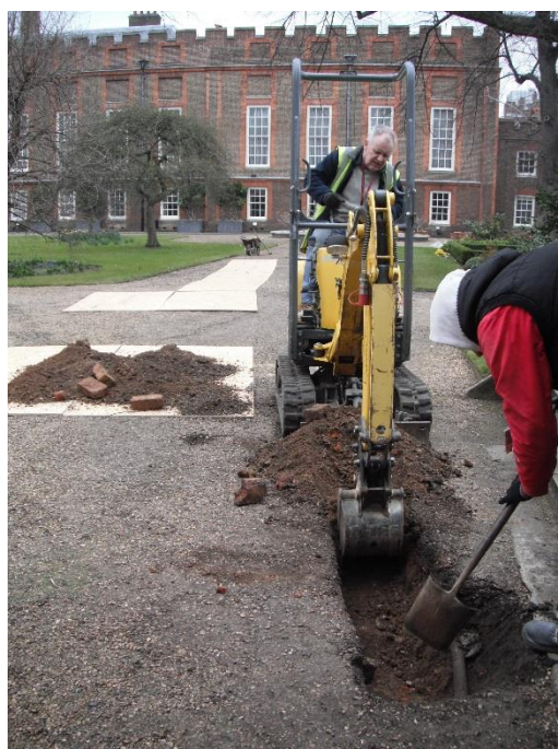
Plate 1: Excavation in progress, view north
