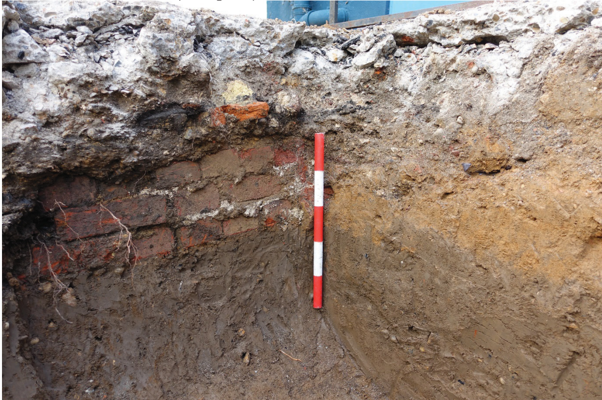
Plate 11: Section in Trench 3 (looking east)
