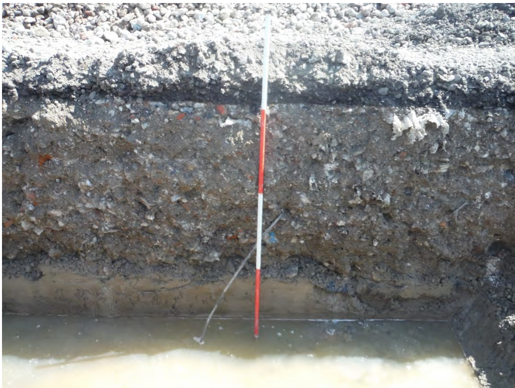
Plate 6: Trench 4 showing depth of trench and in particular the hard-core, view south-west
