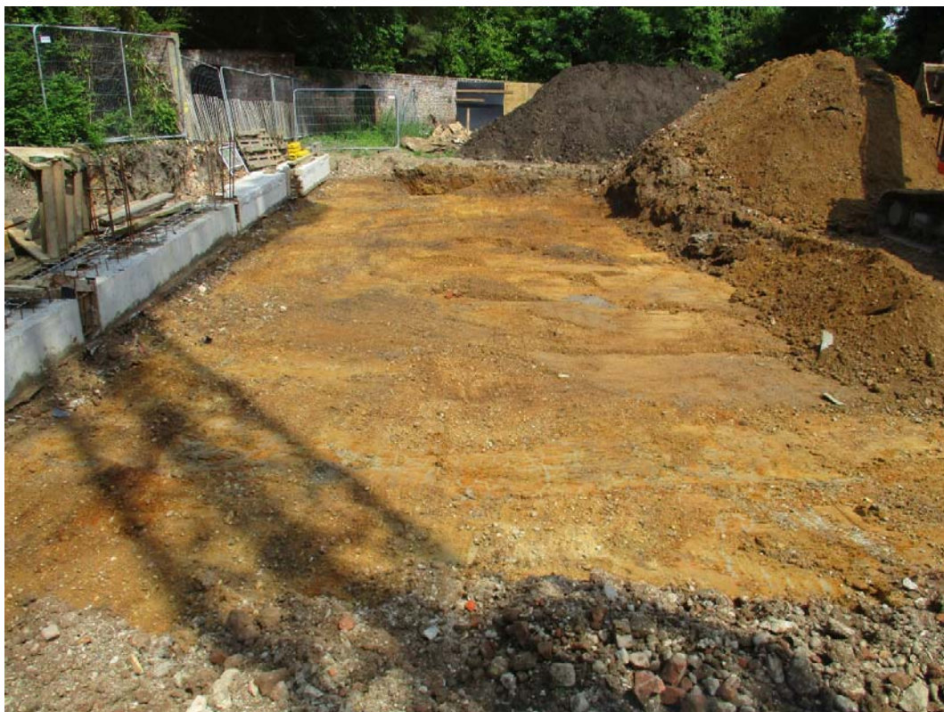
Plate 1. North facing shot of excavations showing recently exposed natural sands and gravels
