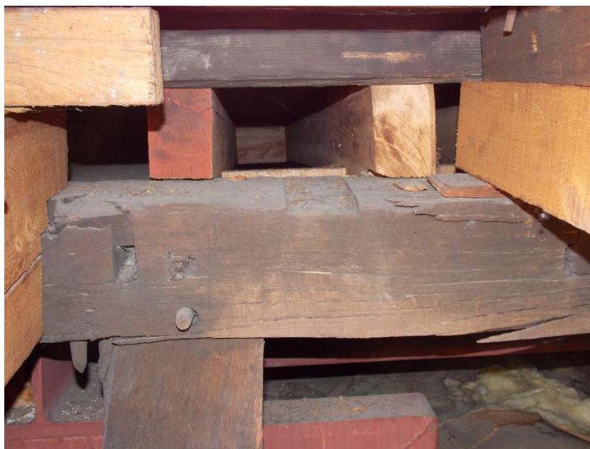
Plate 3: Three phases of roof construction, looking south
