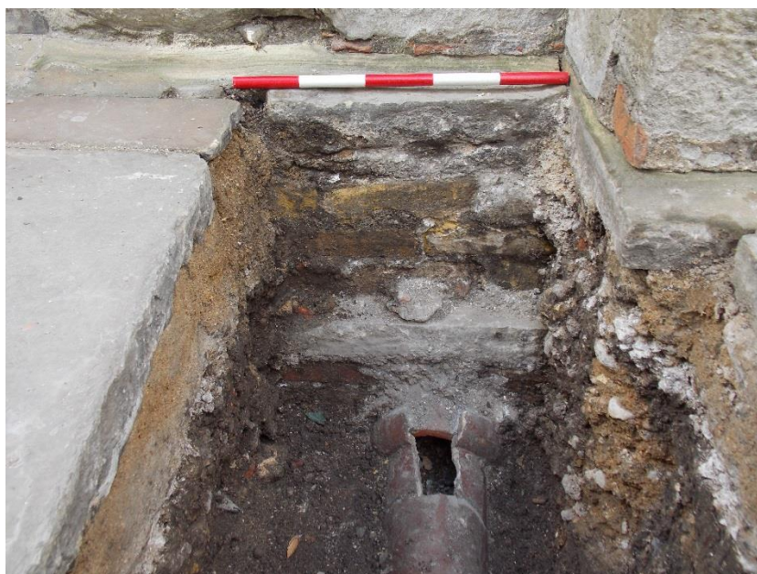
Plate 2: Brick footing for the Devereux Screen, looking west
