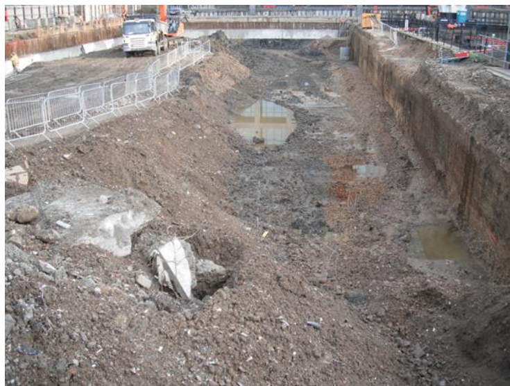
Plate 5. Partly demolished dock wall and excavation area, view east
