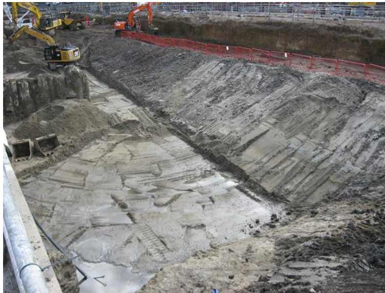
Plate 3: Bulk excavation showing sands and gravels
