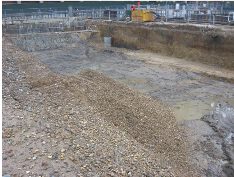
Plate 4: Excavation through alluvial deposits
