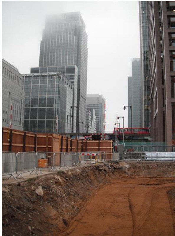
Plate 1: Watching brief excavation area, view east
