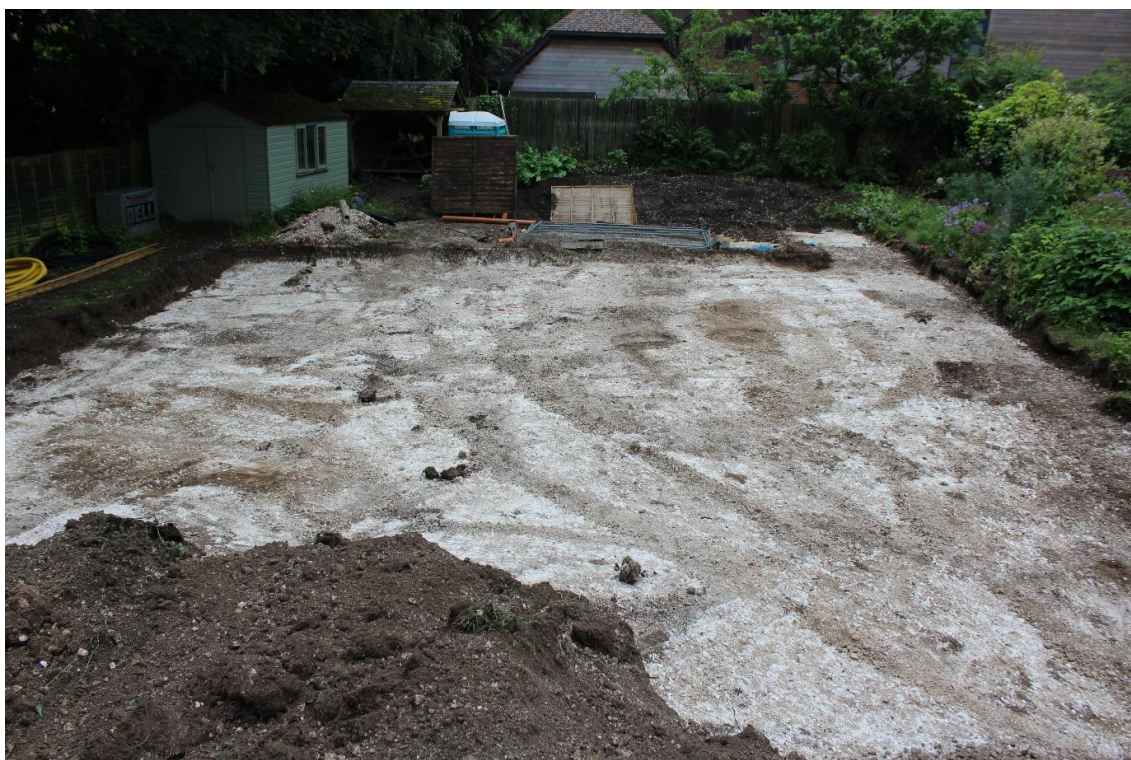
Plate 1 View of Main Area of Construction
