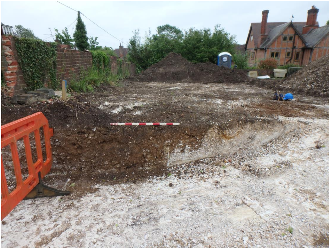
Plate 3: View of excavated and backfilled area behind boundary area, looking east
