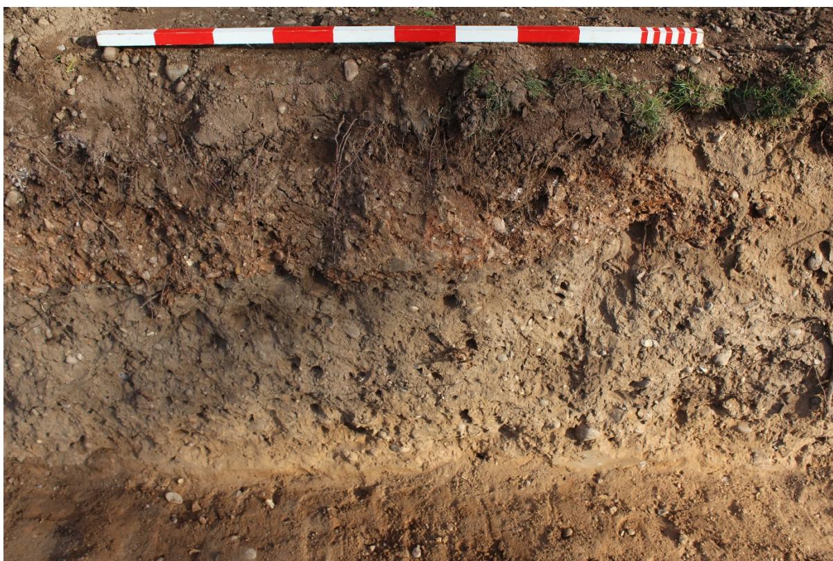
Plate 6: Northeast facing shot of Section 4.
