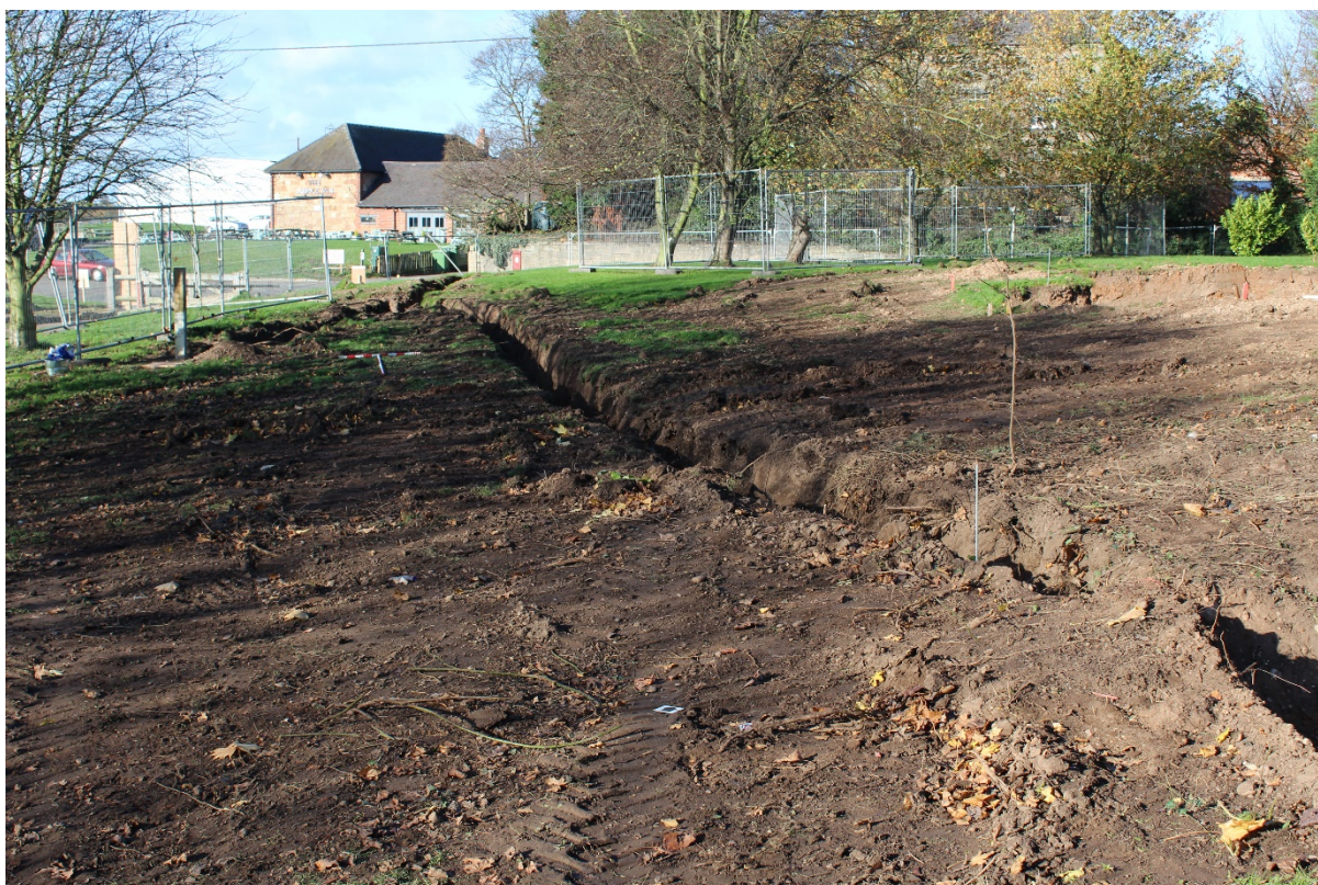
Plate 3: Northwest facing shot of trench cut for services.
