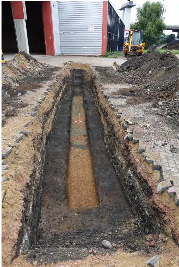
Plate 1: Natural brickearth in the base of Trench 1 (looking north-east)
