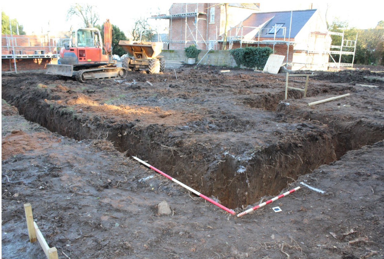
Plate 1: East facing shot across house footings area.
