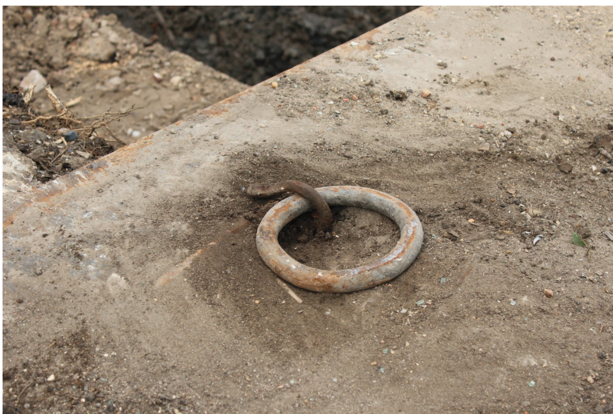
Plate 10: Looking north west, mooring ring attached to post war canal wall [7] Trench 4a.
