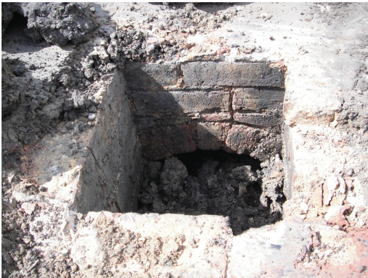
Plate 1: Looking north, brick inspection chamber for north-south drain [15] within area A.
