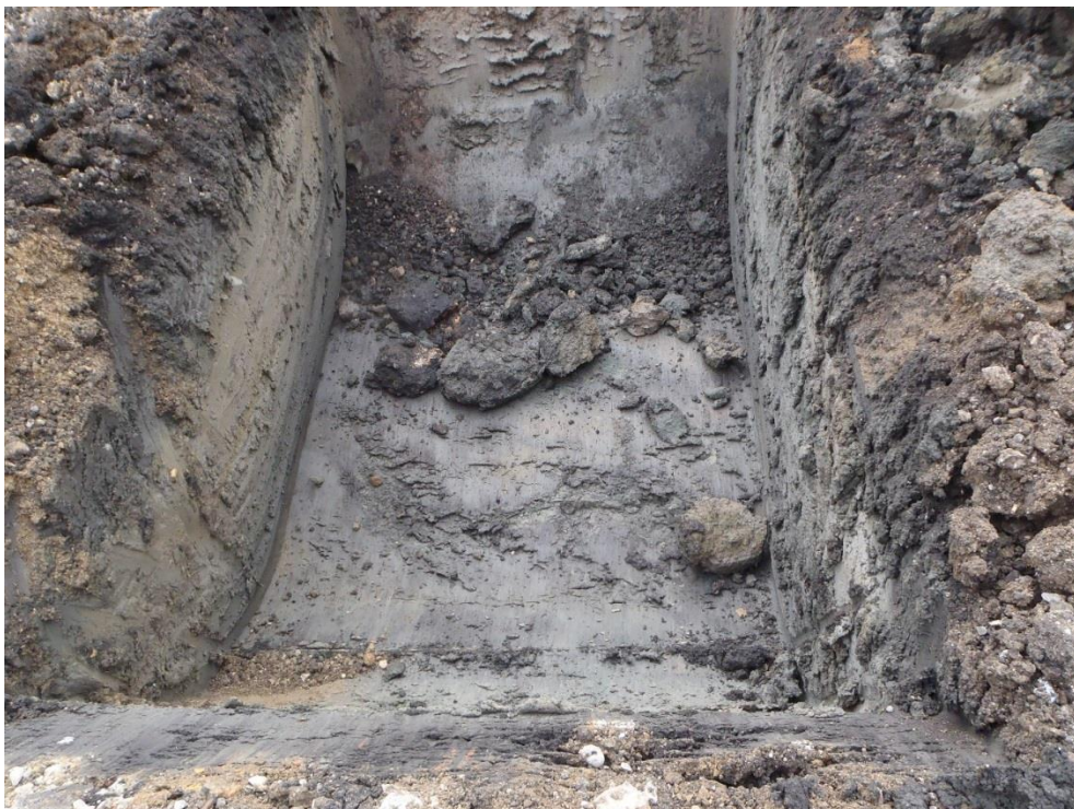
Plate 2: Looking north-east at part of trench
