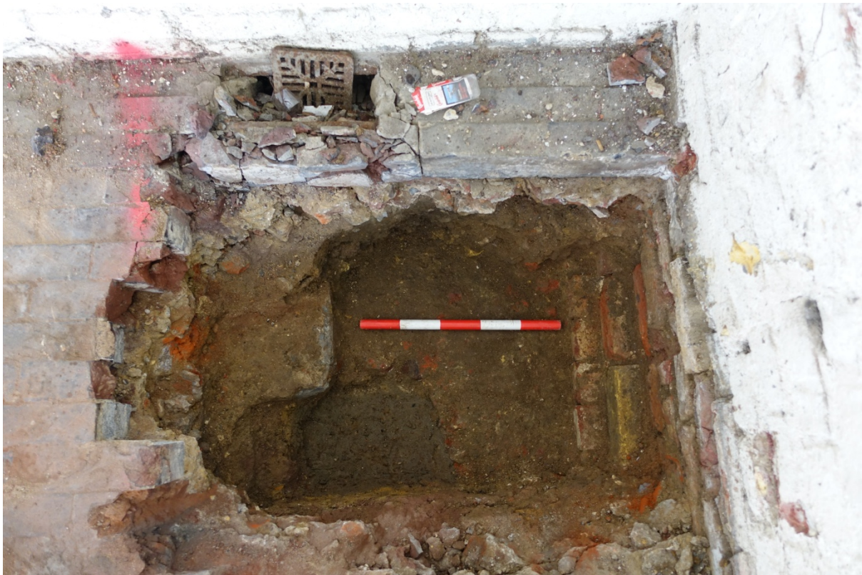
Plate 7: Base of Test Pit 3, showing [3] and current wall foundation (0.5m scale, looking north)
