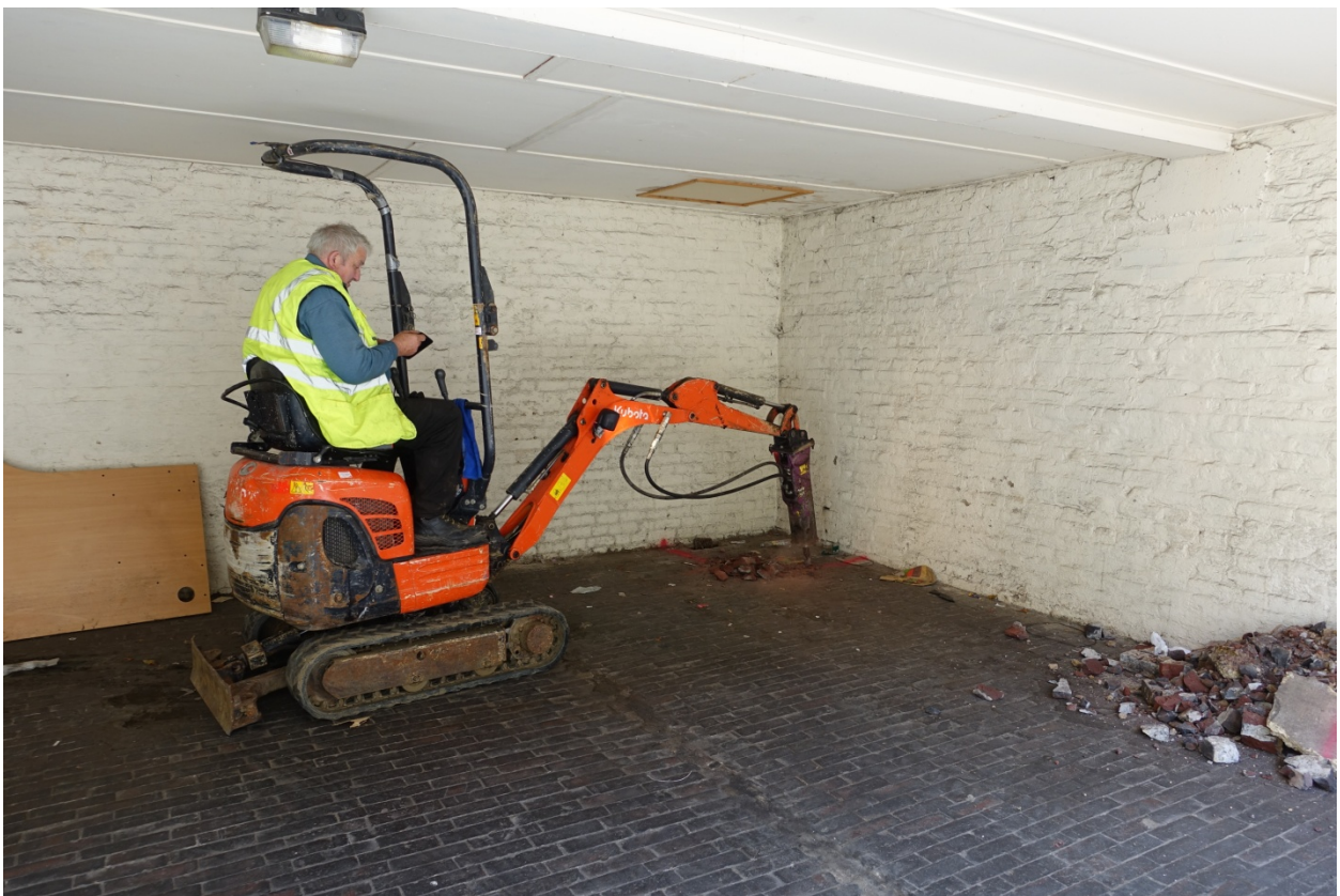
Plate 6: Test Pit 3 at the start of excavation (looking north-east)
