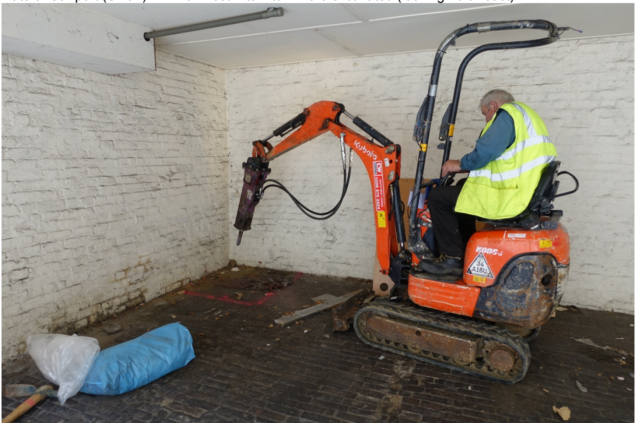
Plate 4: Test Pit 2 at the start of excavation (looking north-west)
