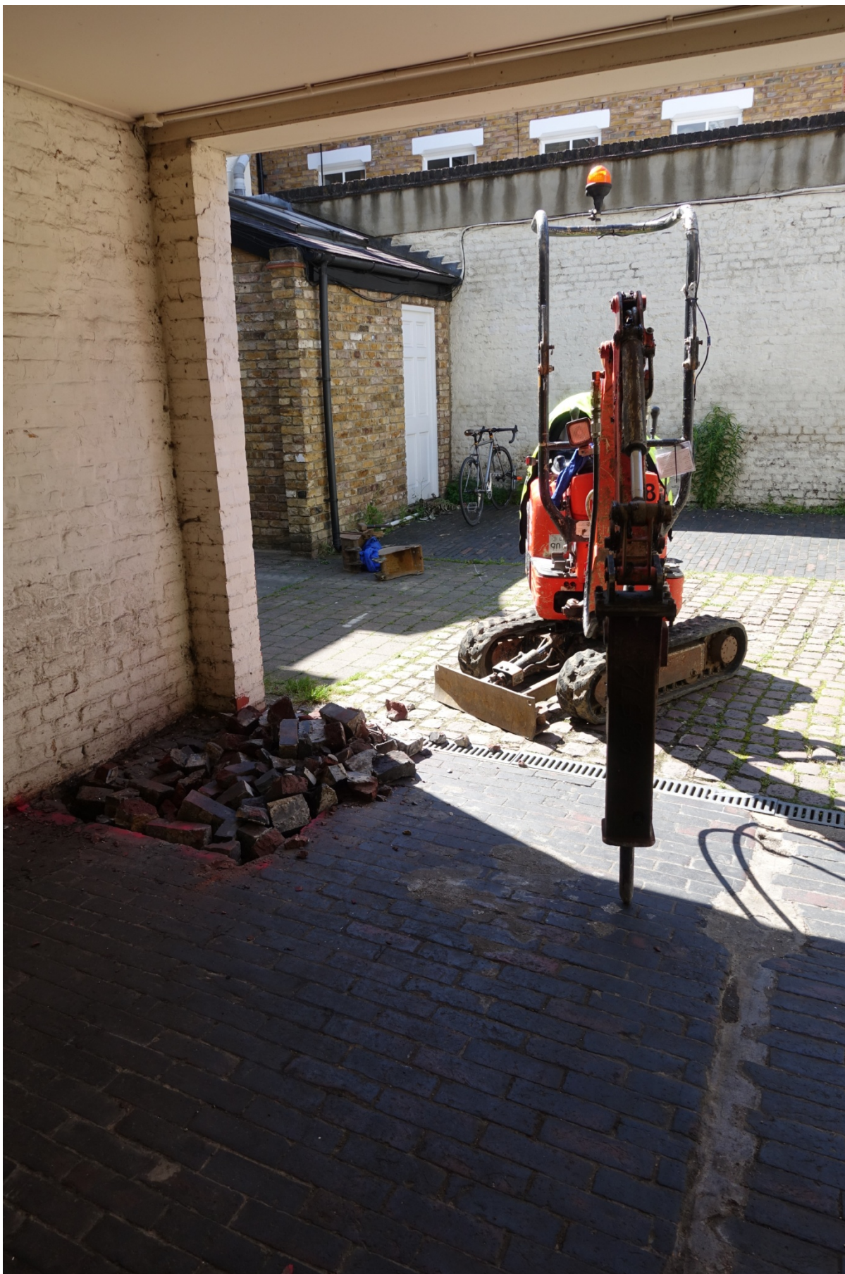
Plate 10: Test Pit 4 at the start of excavation (looking south-east)
