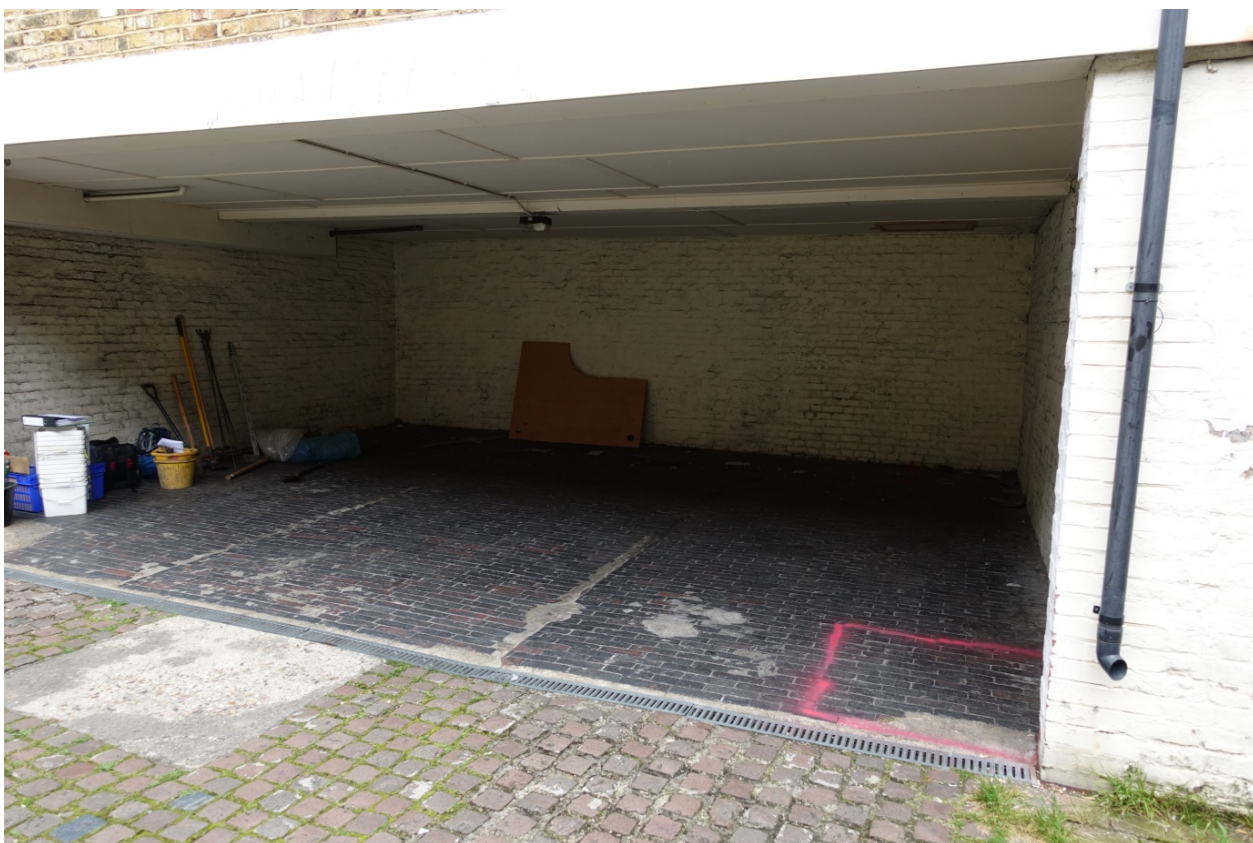
Plate 9: Location of Test Pit 4 before excavation (looking north-west)
