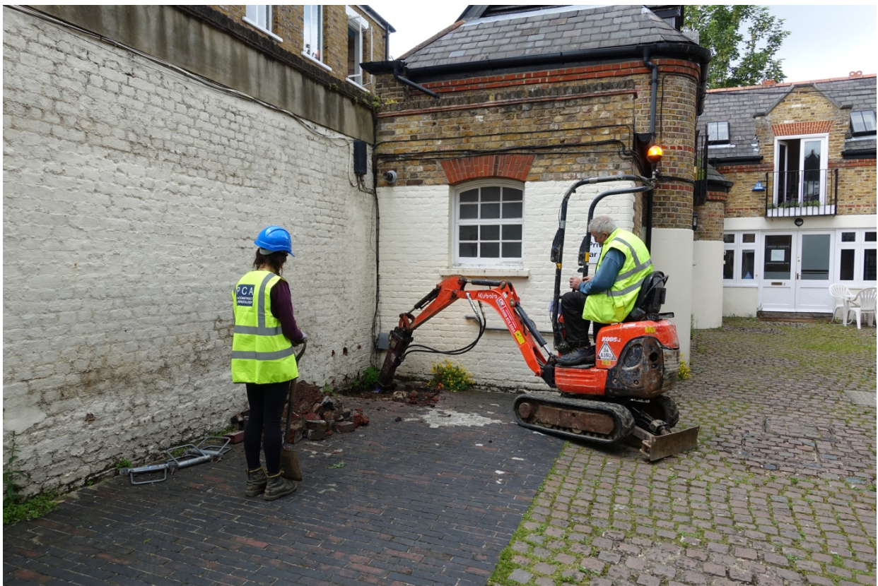
Plate 1: Excavation of Test Pit 1 (looking south-west)
