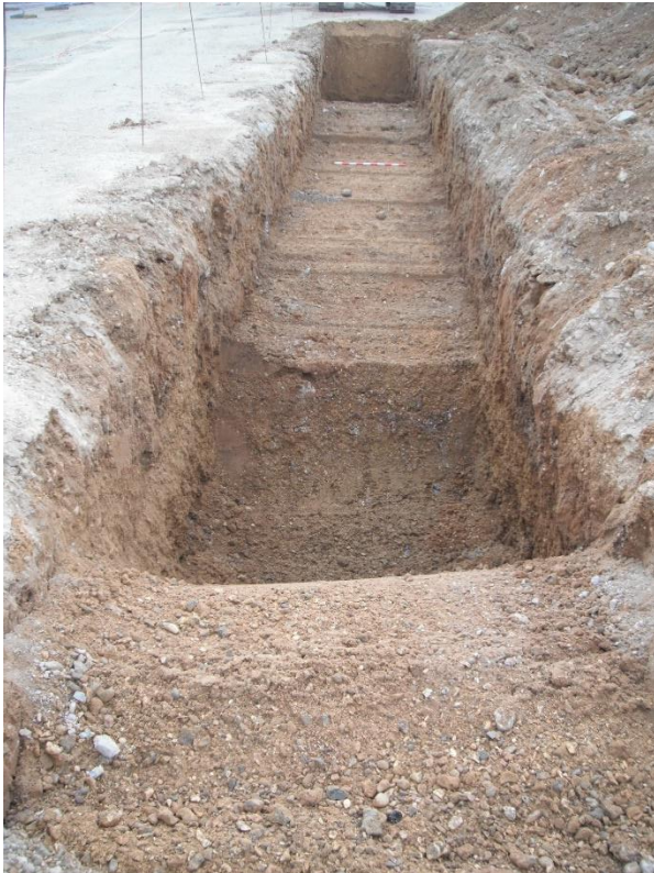
Plate 5: Looking west, Trench 3
