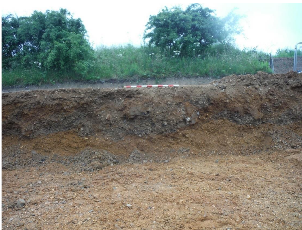
Plate 2: Looking south, Attenuation Tank north facing section [4] and [5]
