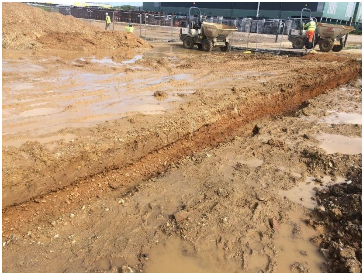
Plate 3: Looking north west, Access road drainage including subsoil [10]
