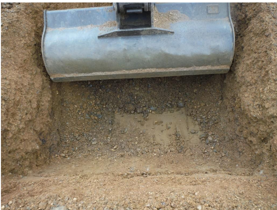
Plate 4: Looking east, natural sand [17] southern sondage in Attenuation Tank
