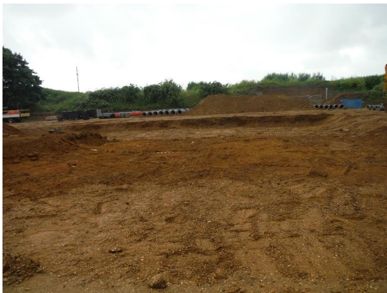
Plate 1: Looking south, Attenuation Tank
