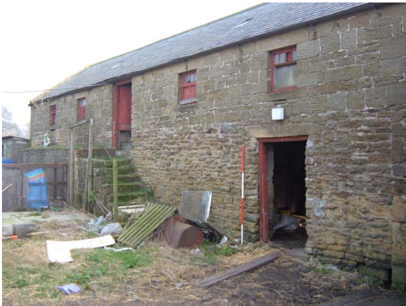
Plate 54. Hemmel/granary, north elevation – west part, from the north (2m scale).
