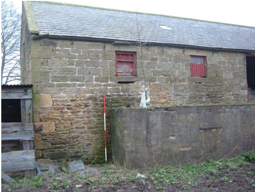
Plate 53. Hemmel/granary, north elevation – east part, from the north (2m scale).
