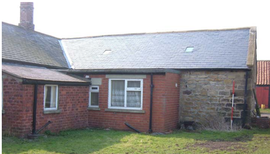
Plate 30. Stable and cottage (extensions), east elevation, from the east (2m scale).
