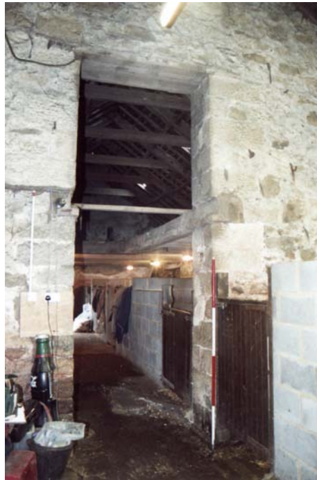
Plate 60. Threshing barn (ground floor), interior, from the north-west (2m scale).
