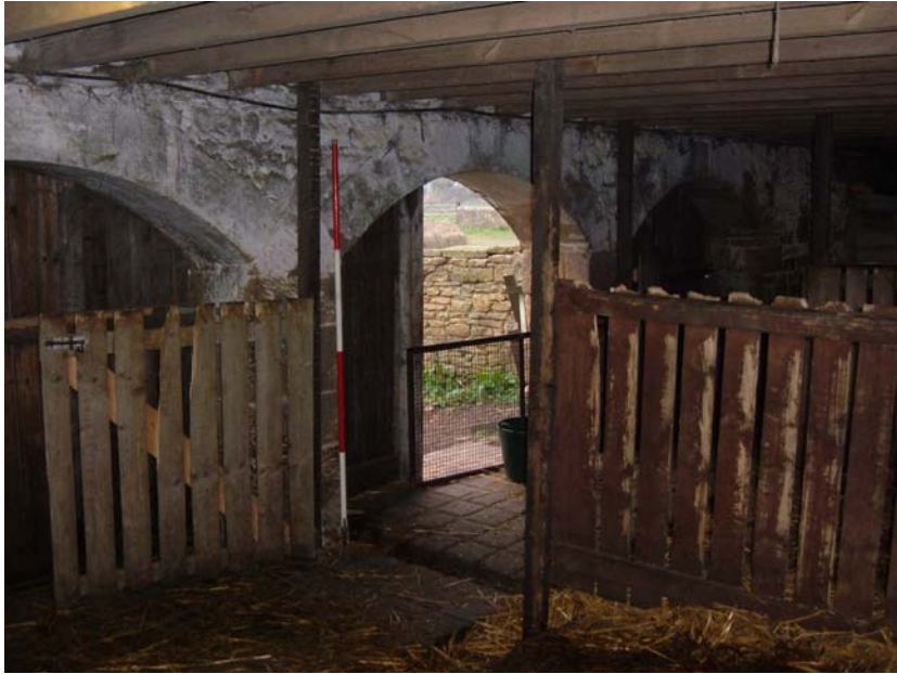
Plate 69. Hemmel, interior, south wall, arches, from the north-east (2m scale).
