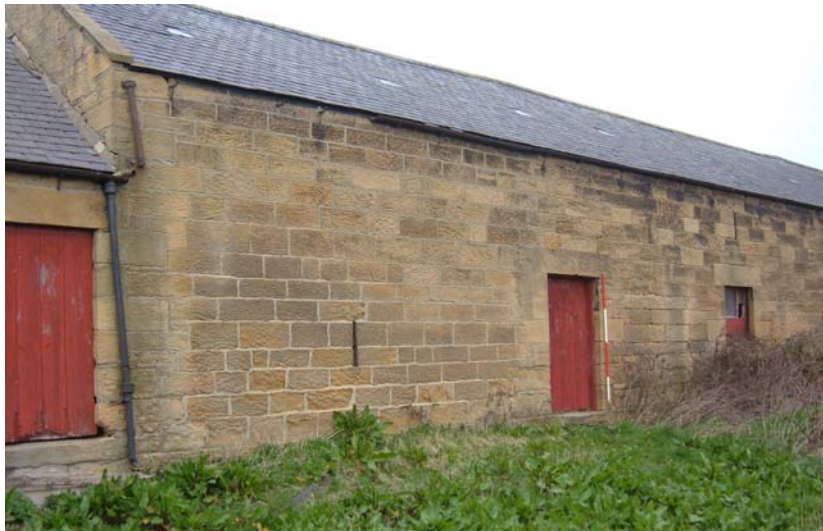
Plate 42. Threshing Barn, south elevation – west part, from the south (2m scale).
