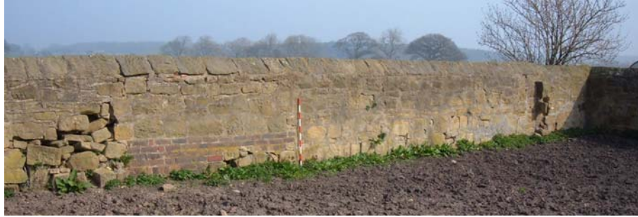
Plate 19. Fold yard, north wall, interior, from the south-west ( 1m scale ).
