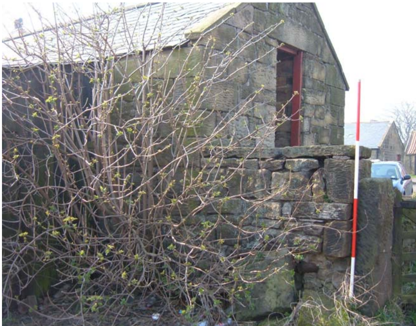
Plate 26. Piggery, east and north elevations, from the north-east (2m scale).
