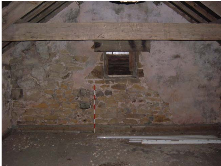
Plate 58. Granary, interior, east wall detail, from the west ( 1m scale ).
