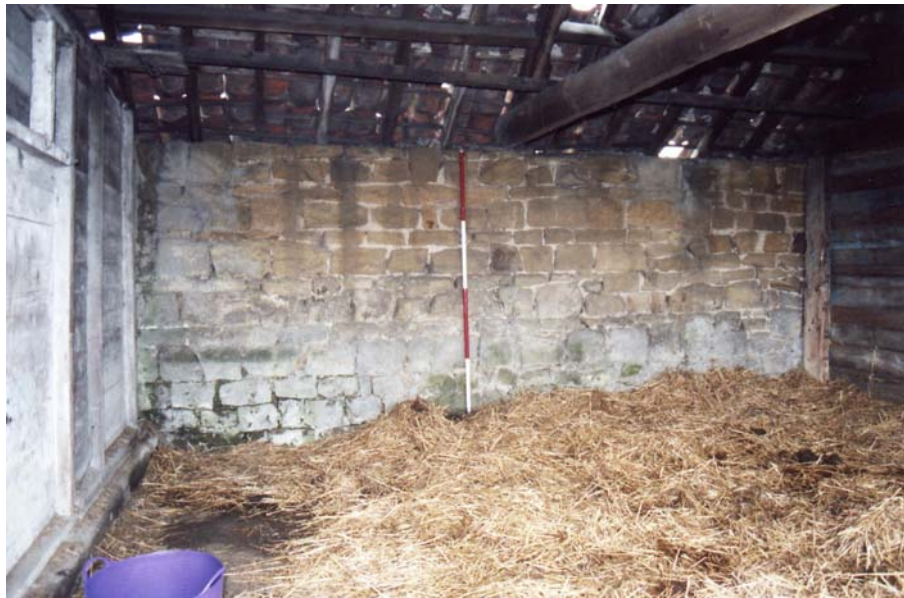
Plate 4. Cart shed, central bays, interior, from the east ( 2m scale ).
