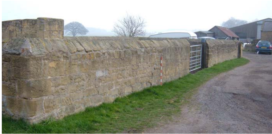
Plate 14. Fold yard, south wall, exterior, from the south-west ( 1m scale ).
