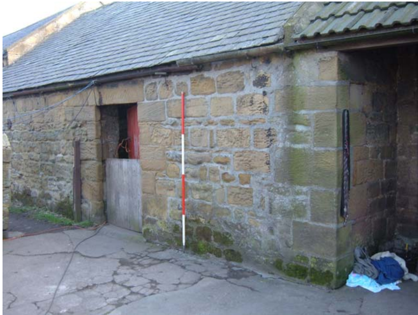
Plate 39. Byre, north elevation, from the north-west (2m scale).
