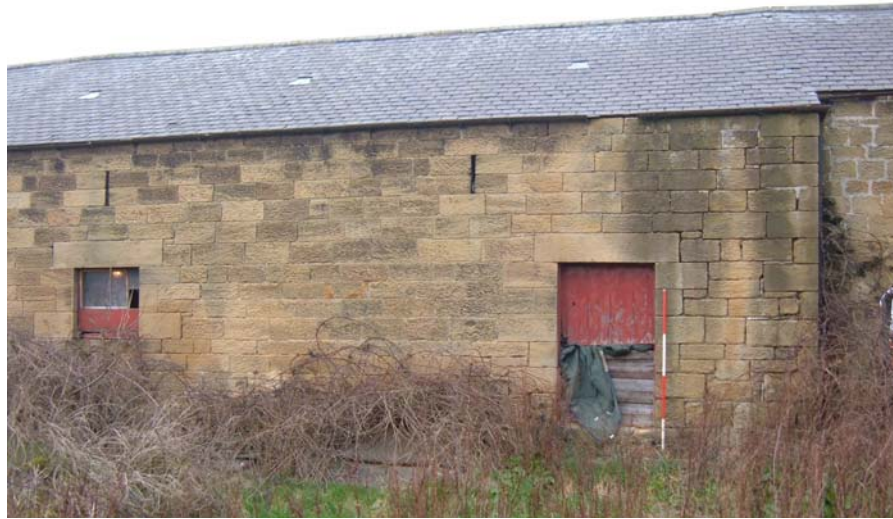
Plate 43. Threshing Barn, south elevation – east part, from the south (2m scale).
