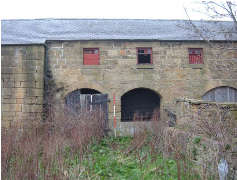
Plate 49. Hemmel/granary, south elevation – west part, from the south (2m scale).
