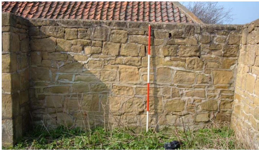
Plate 10. Former building, east bay, interior, from the east (2m scale).
