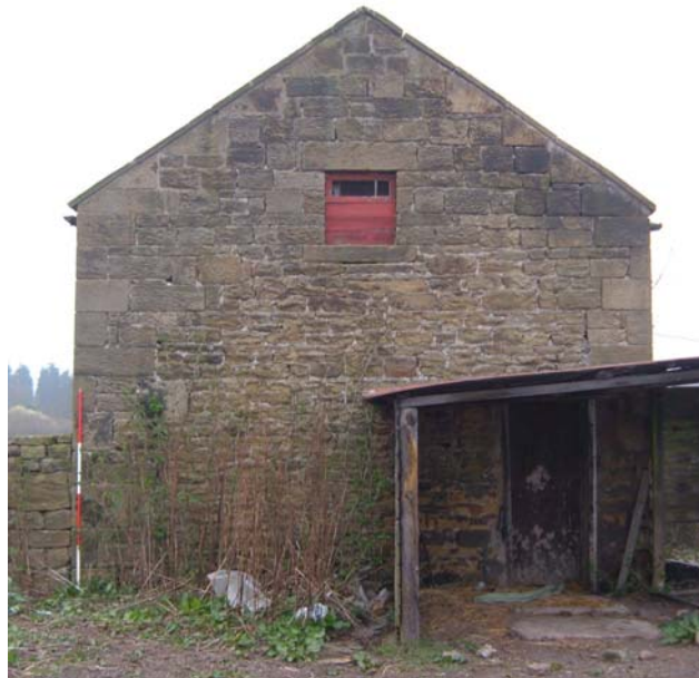
Plate 52. Hemmel/granary, east elevation, from the east (2m scale).
