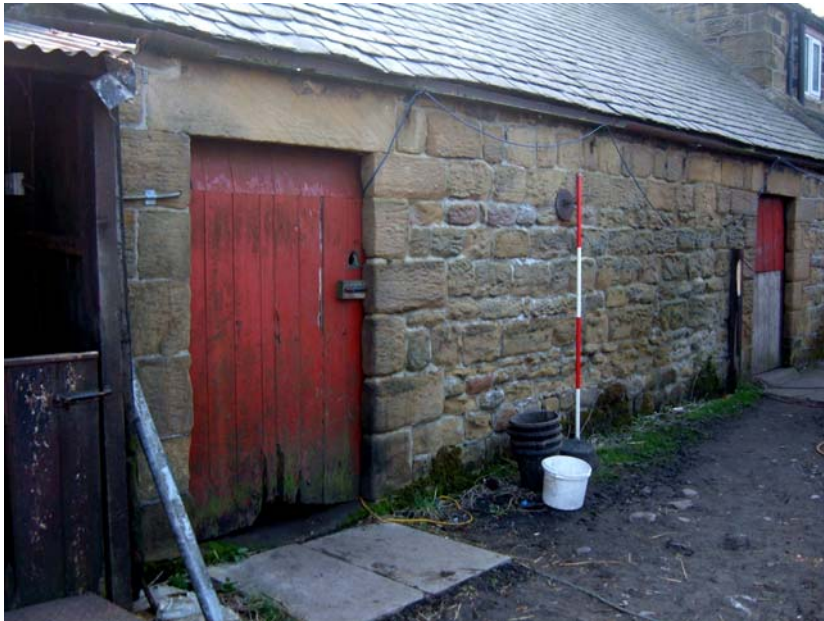
Plate 40. Byre, north elevation, from the north-east (2m scale).
