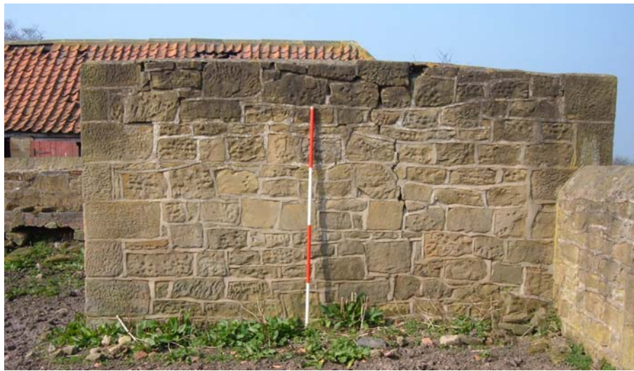
Plate 12. Former building, east elevation, from the east (2m scale).
