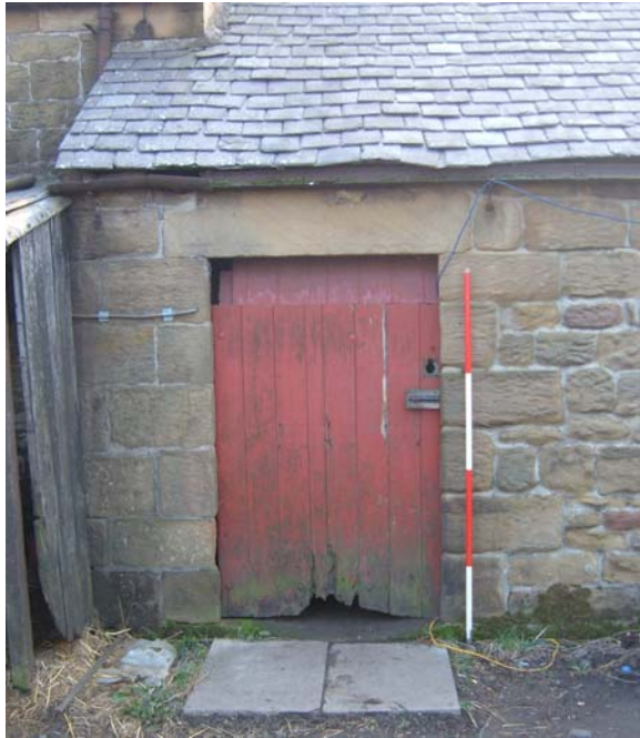
Plate 41. Byre, north elevation, east door, from the north (2m scale).
