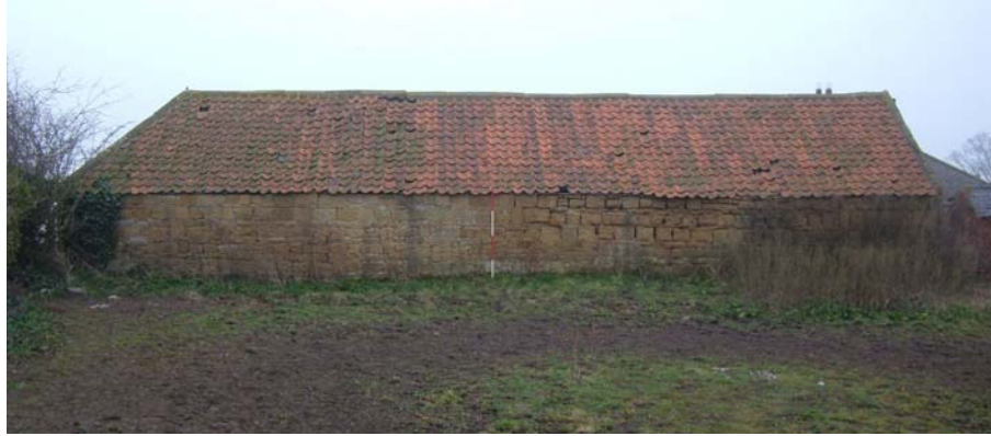
Plate 1. Cart shed, west elevation, from the west (2m scale).
