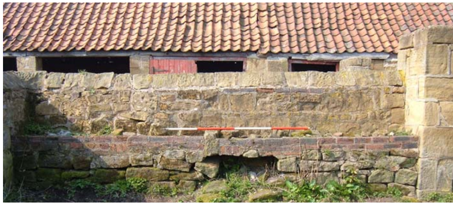
Plate 20. Fold yard, west wall, interior, from the east ( 2m scale ).
