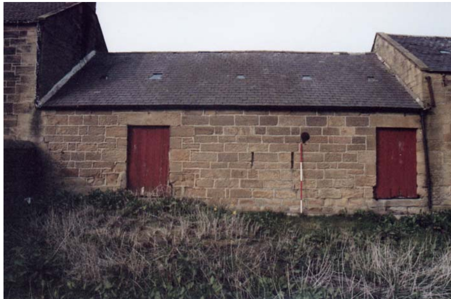
Plate 38. Byre, south elevation, from the south (2m scale).
