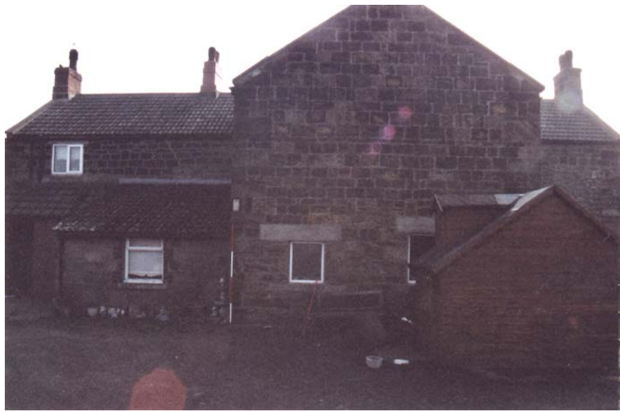
Plate 35. Farmhouse, north elevation – central part, from the north (2m scale).
