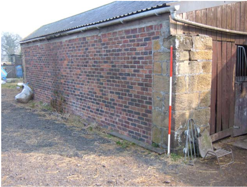
Plate 45. Threshing Barn, north extension, from the north-west ( 2m scale ).
