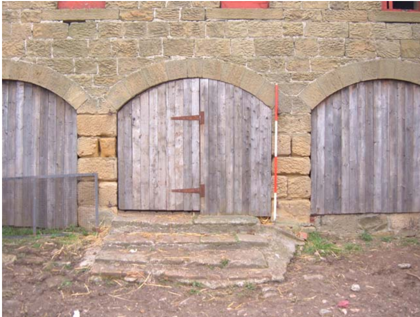
Plate 51. Hemmel/granary, south elevation, arch detail, from the south (2m scale).
