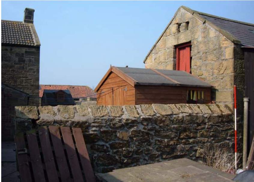
Plate 25. Piggery, south elevation, from the south-east (2m scale).
