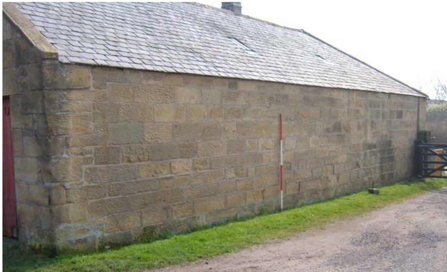
Plate 27. Stable, west elevation, from the north-west (2m scale).
