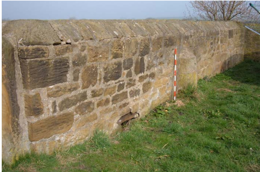
Plate 15. Fold yard, east wall, exterior, from the south-east ( 1m scale ).
