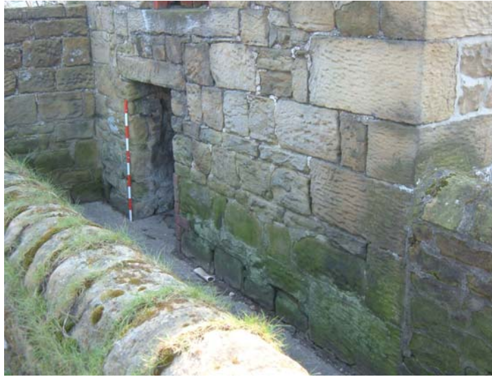
Plate 23. Piggery, north elevation, entrance detail, from the west (1m scale).
