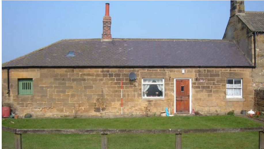
Plate 29. Stable and cottage, south elevation, from the south (2m scale).
