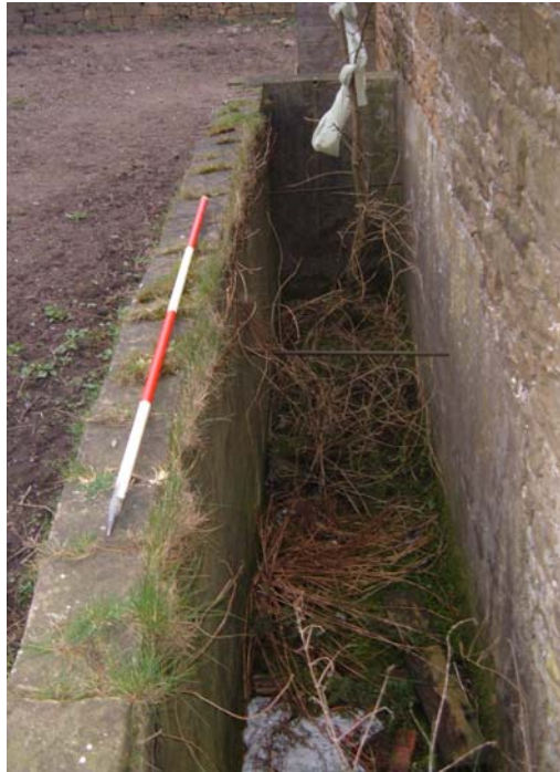
Plate 56. Hemmel/granary, external water tank detail, from the west ( 2m scale ).
