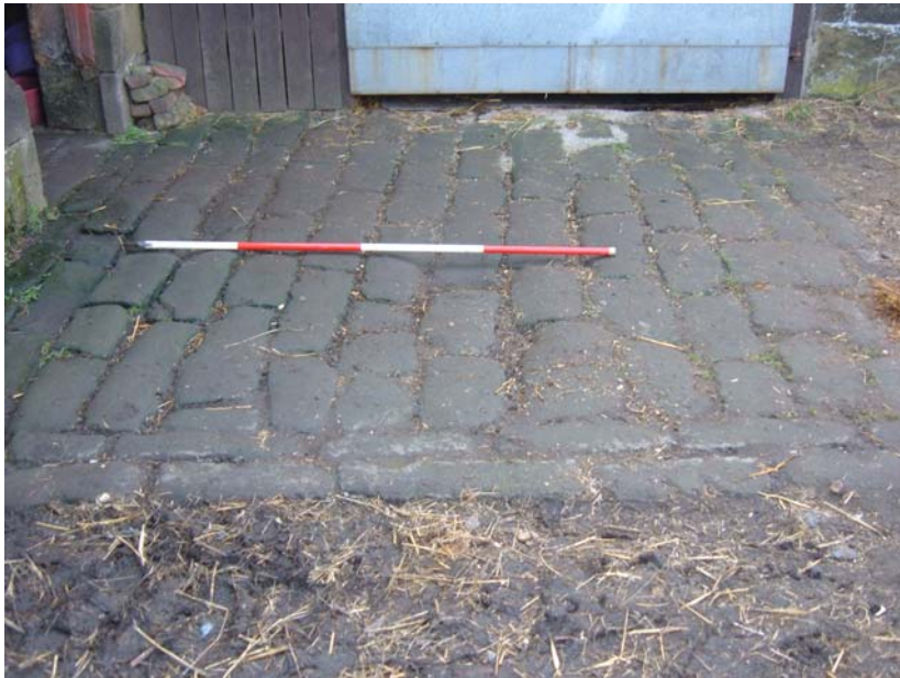
Plate 48. Threshing Barn, east end, exterior surface, from the east (2m scale).
