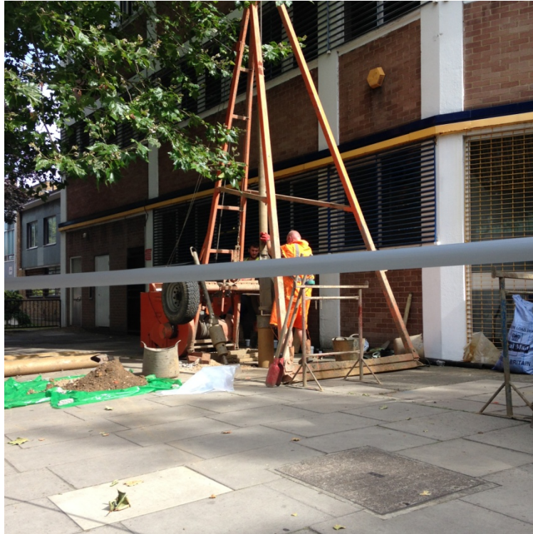
Plate 1: BH1, Working Shot.
