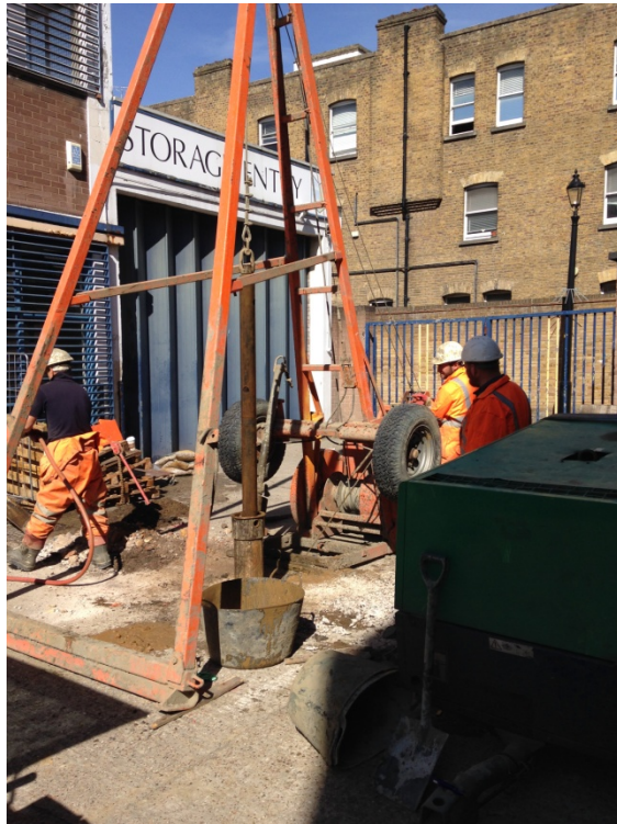
Plate 3: BH2, Working Shot
