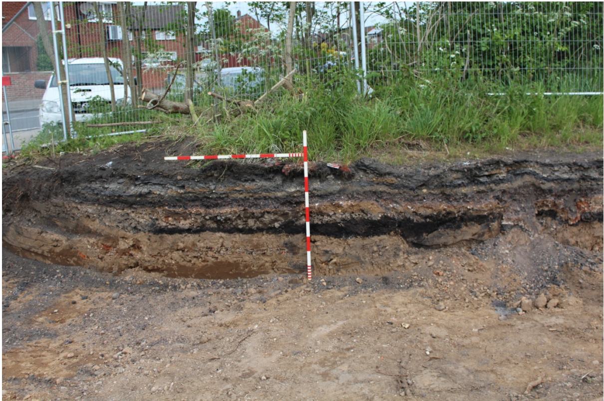
Plate 3: North facing view of Section 3 showing the sequence of tarmac paths and underlying bedding layers
