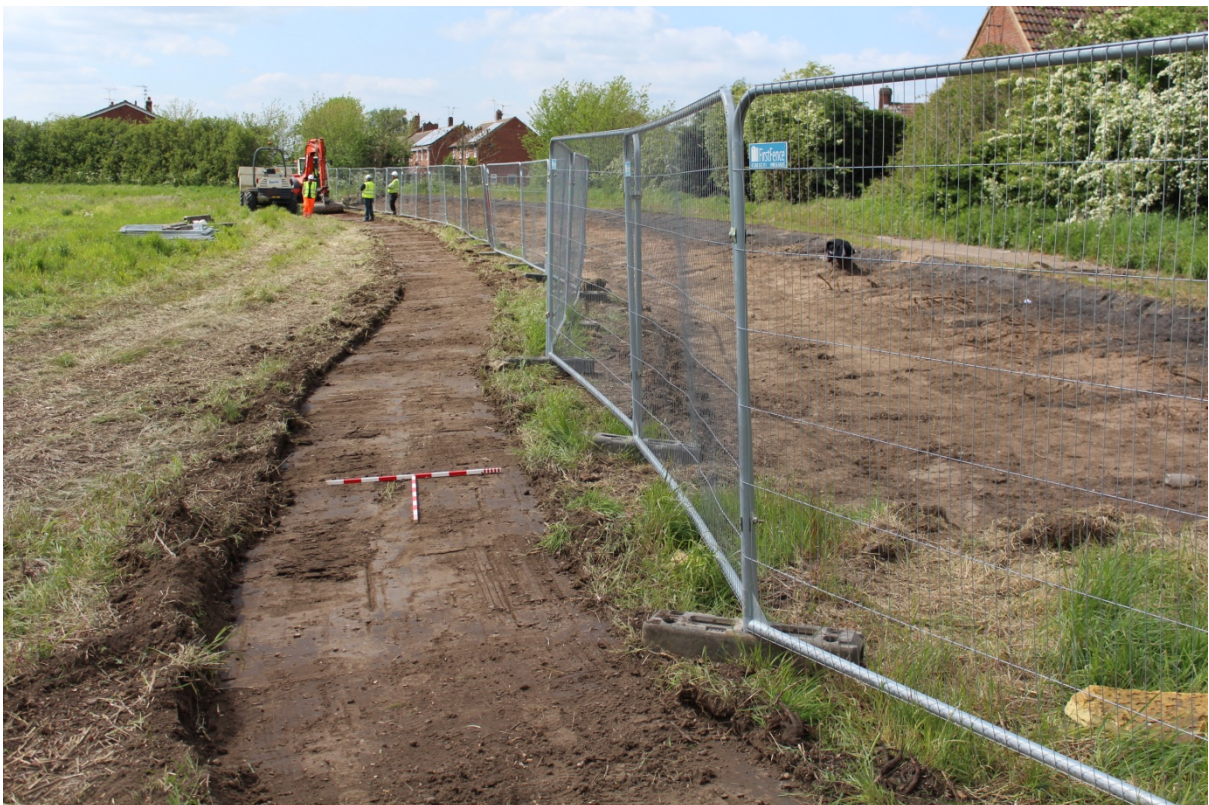
Plate 2: West facing view of topsoil strip along new access road.
