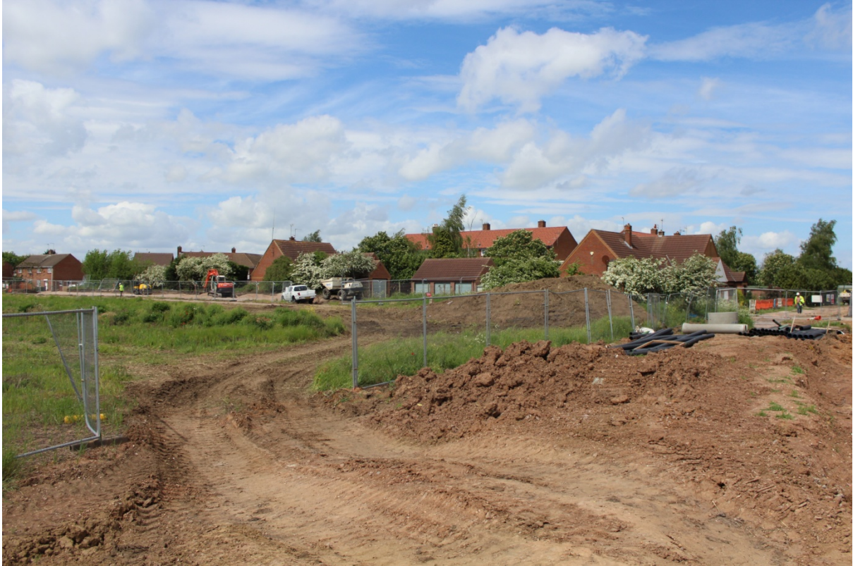
Plate 1: Northwest facing shot Area 11 general location shot
