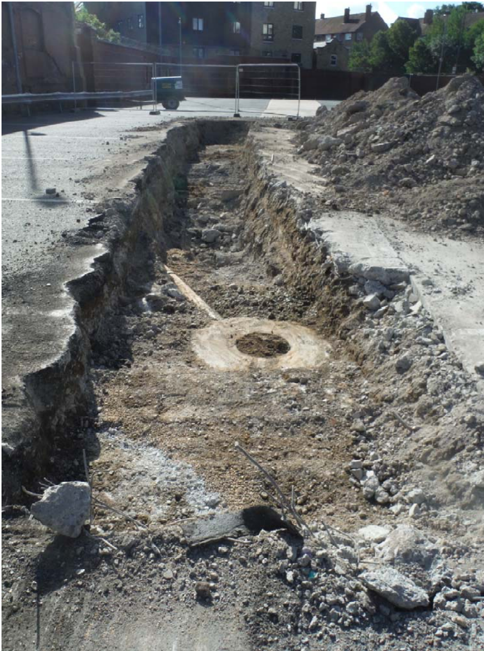
Image 8: East facing view of Trench 6
