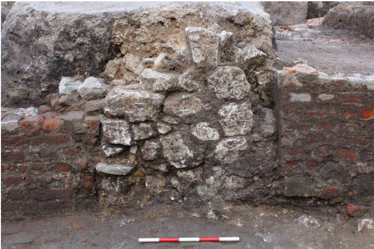
Medieval chalk wall englobed by later walls [1007] left and [898] to the right Scale 0.50m
