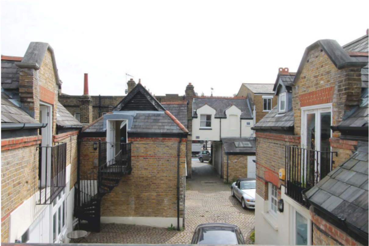
Plate 25 View east to yard from the first floor of Unit 2
