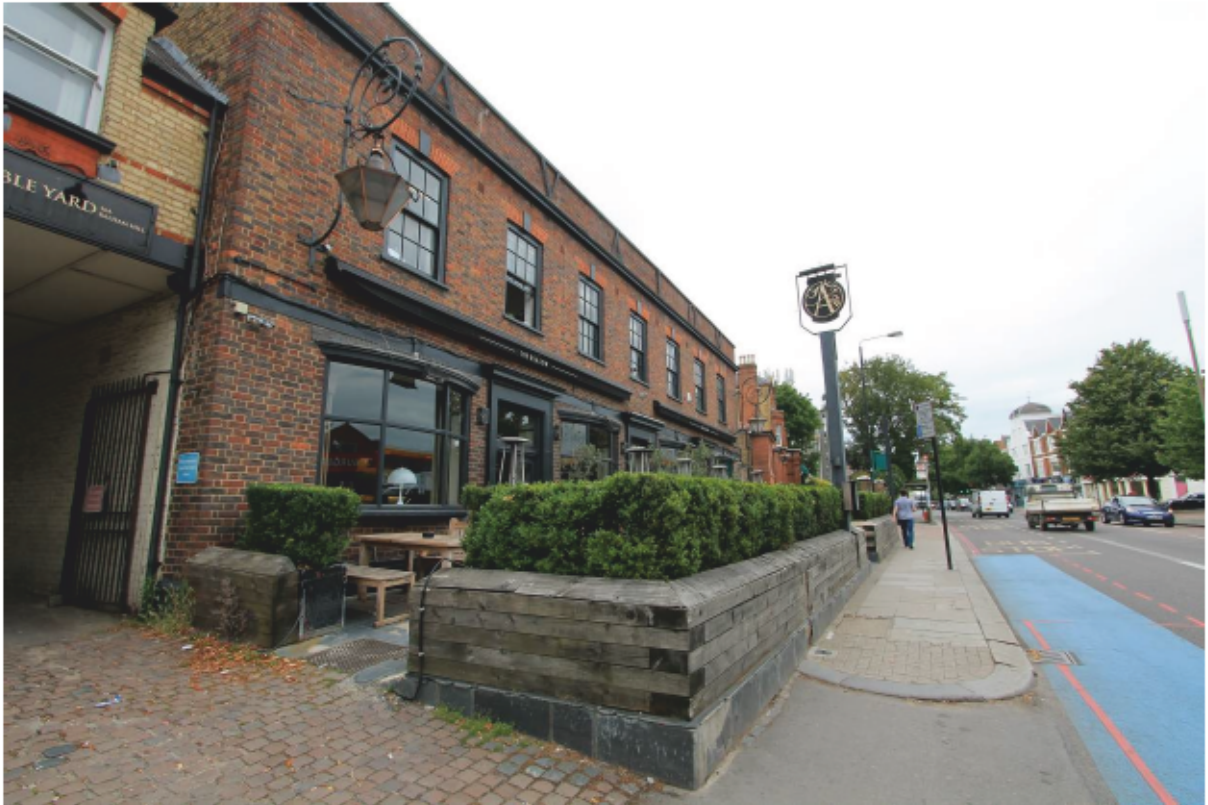
Plate 34 The Avalon looking north
