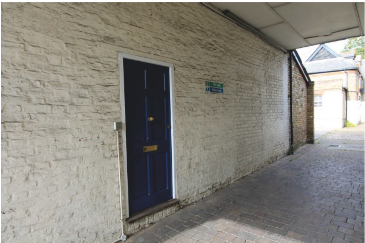
Plate 4 Main entrance to flat and blocked opening to west looking south-west
