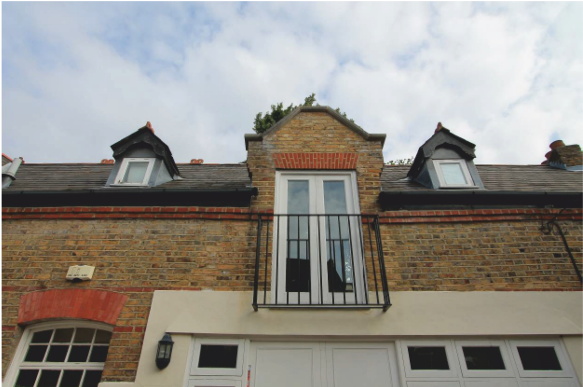
Plate 15 Converted 'taking in' door in the north elevation of Unit 3 looking south
