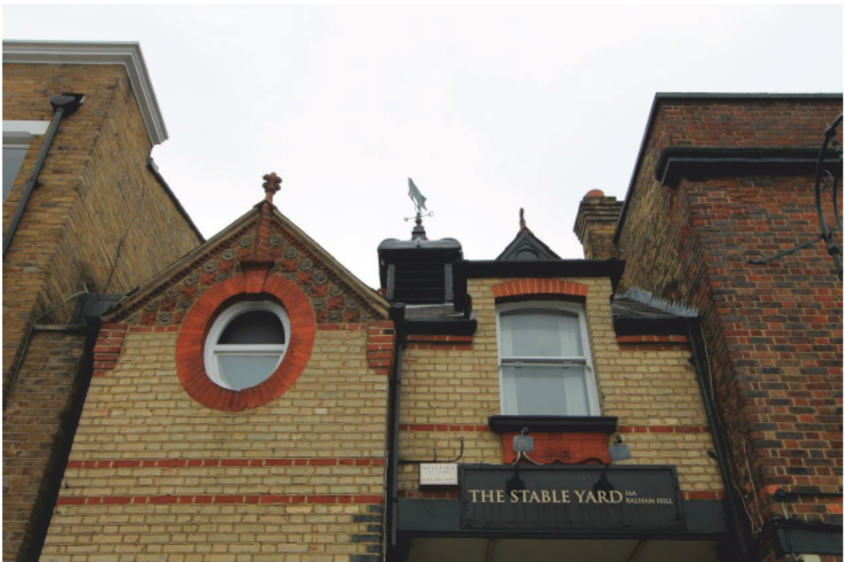
Plate 2 Architectural detailing to facade looking west
