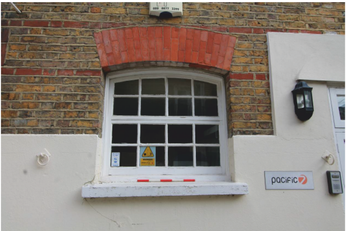
Plate 14 Unit 3, original casement window and tethering ring looking north
