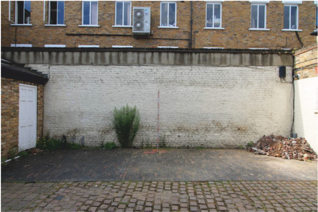
Plate 5 Southern boundary wall, looking south
