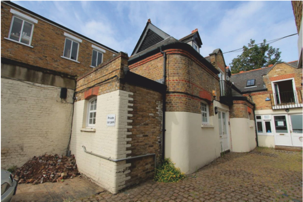
Plate 7 Unit 1 looking south-west, showing later extension
