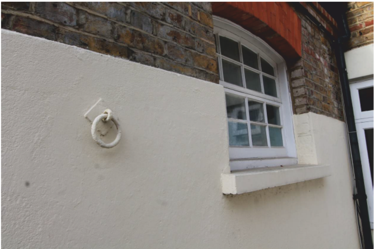
Plate 10 Extant tethering ring, Unit 1 looking south-west
