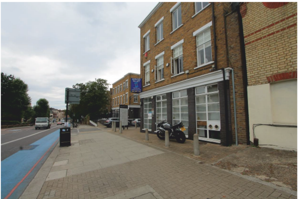
Plate 35 Adjoining Office Building to the south
