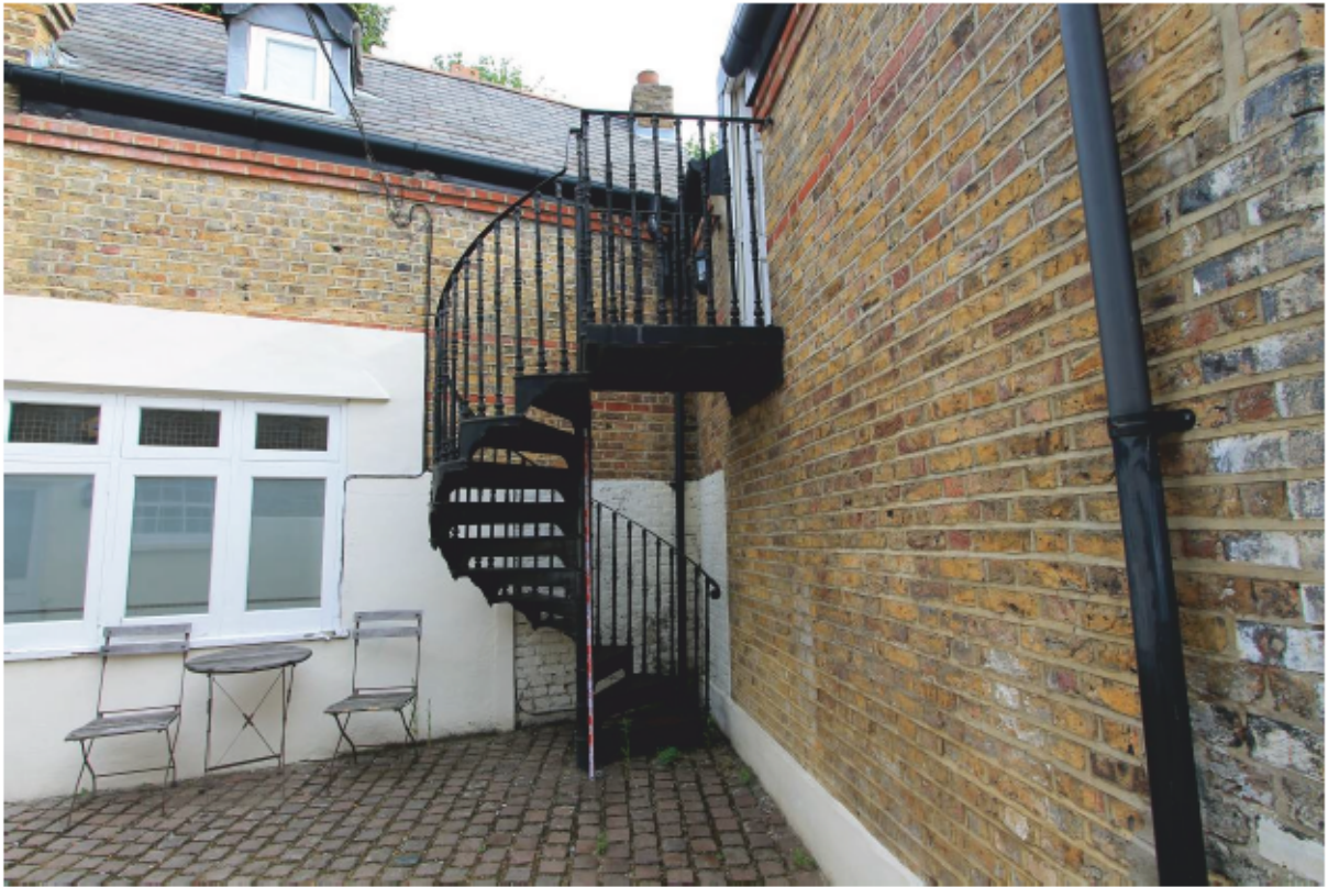
Plate 17 Modern spiral staircase, Unit 4 looking north
