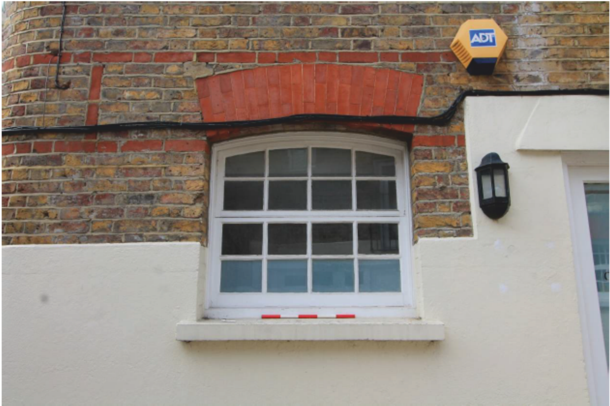
Plate 9 Original casement window with brick segmental arched head looking south
