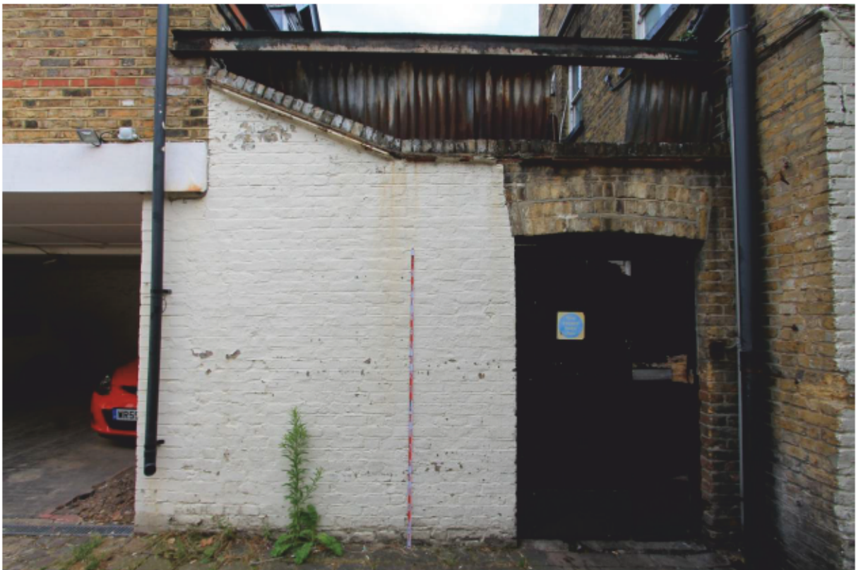
Plate 6 Wall to the rear yard of the public house, looking north
