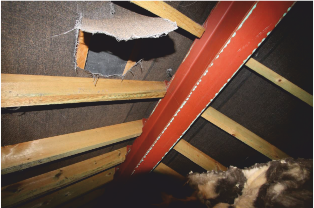
Plate 19 Modern roof structure
