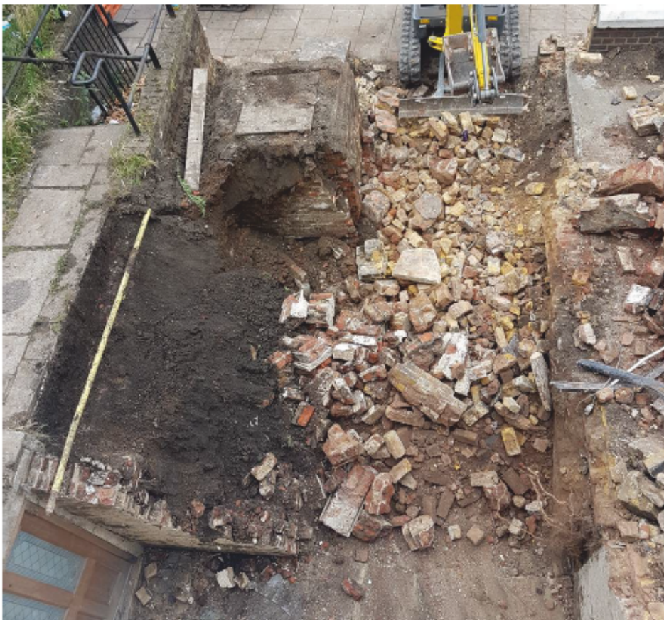
Plate 24 Vault, post demolition
