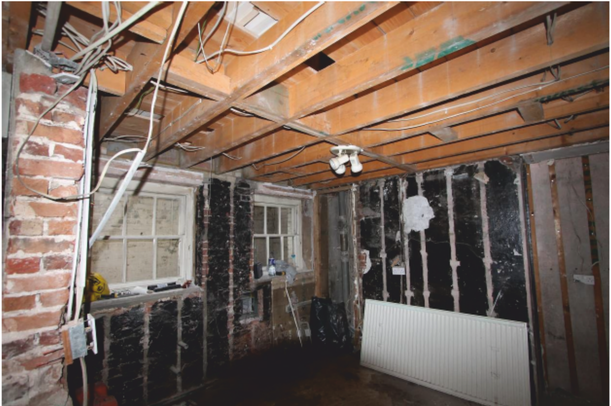
Plate 13 Modern ground floor joists in basement
