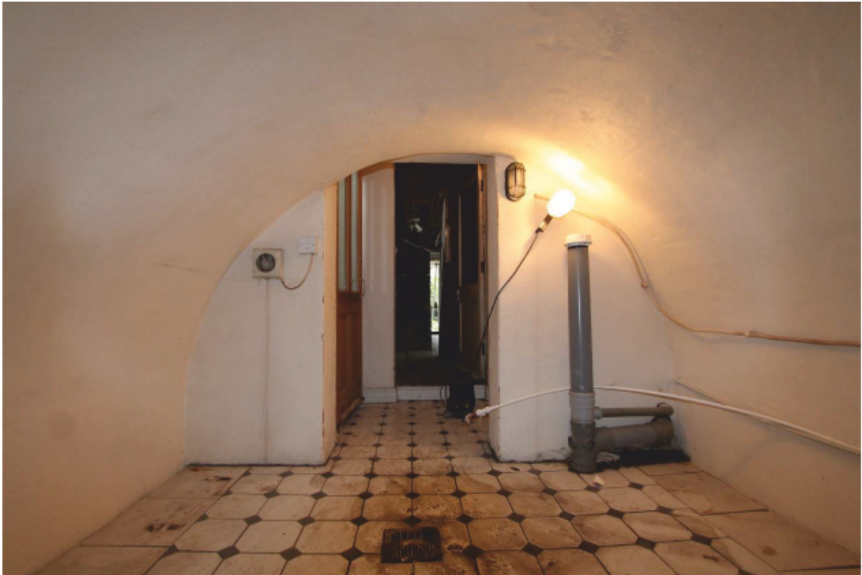
Plate 9 Internal (western) vault, looking south
