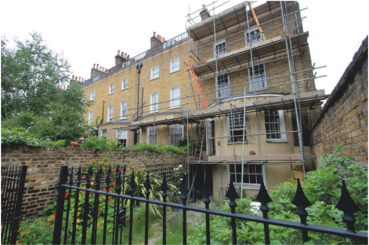
Plate 3 No. 170 New Kent Road, rear elevations
