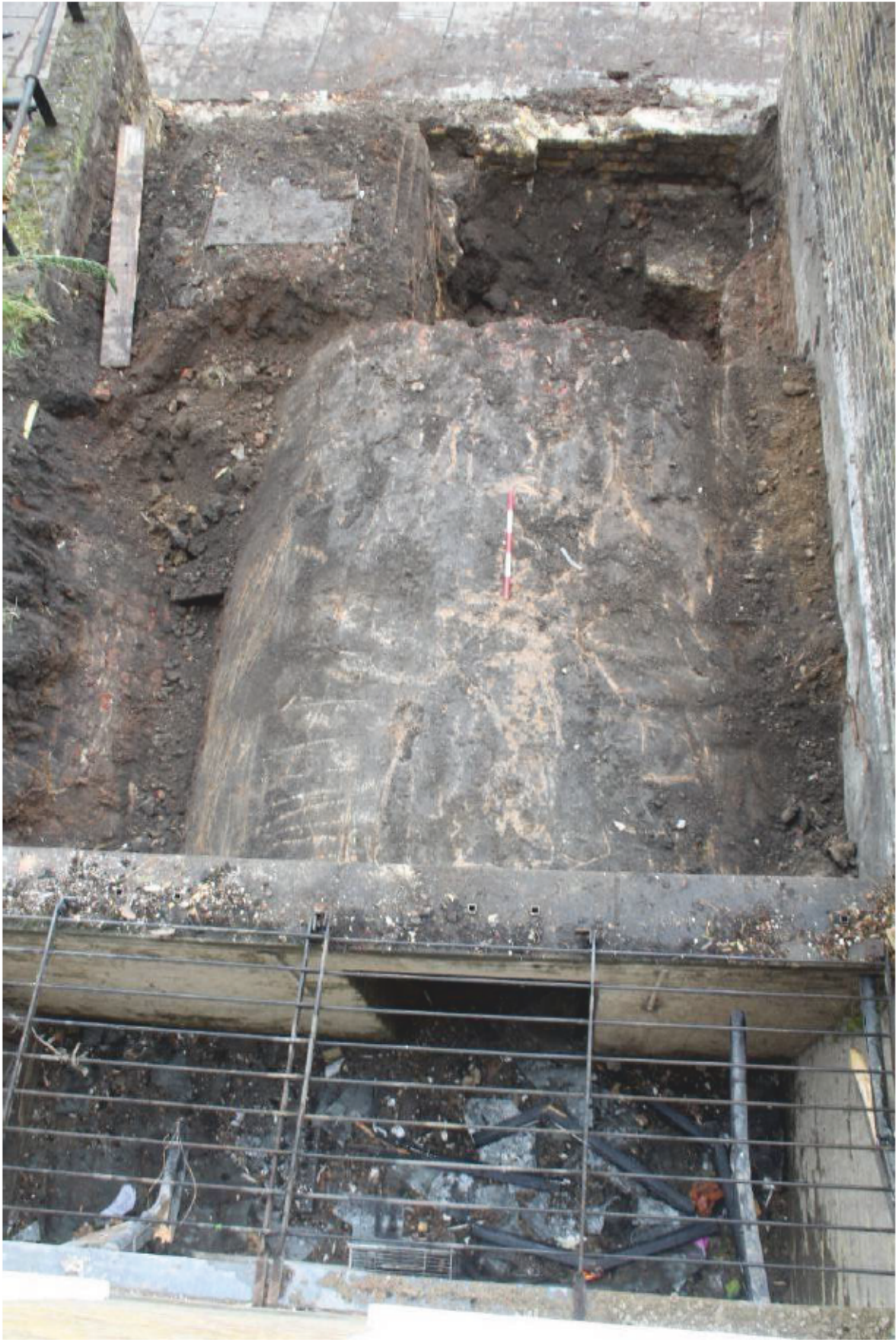
Plate 22 External Vault viewed from first floor
