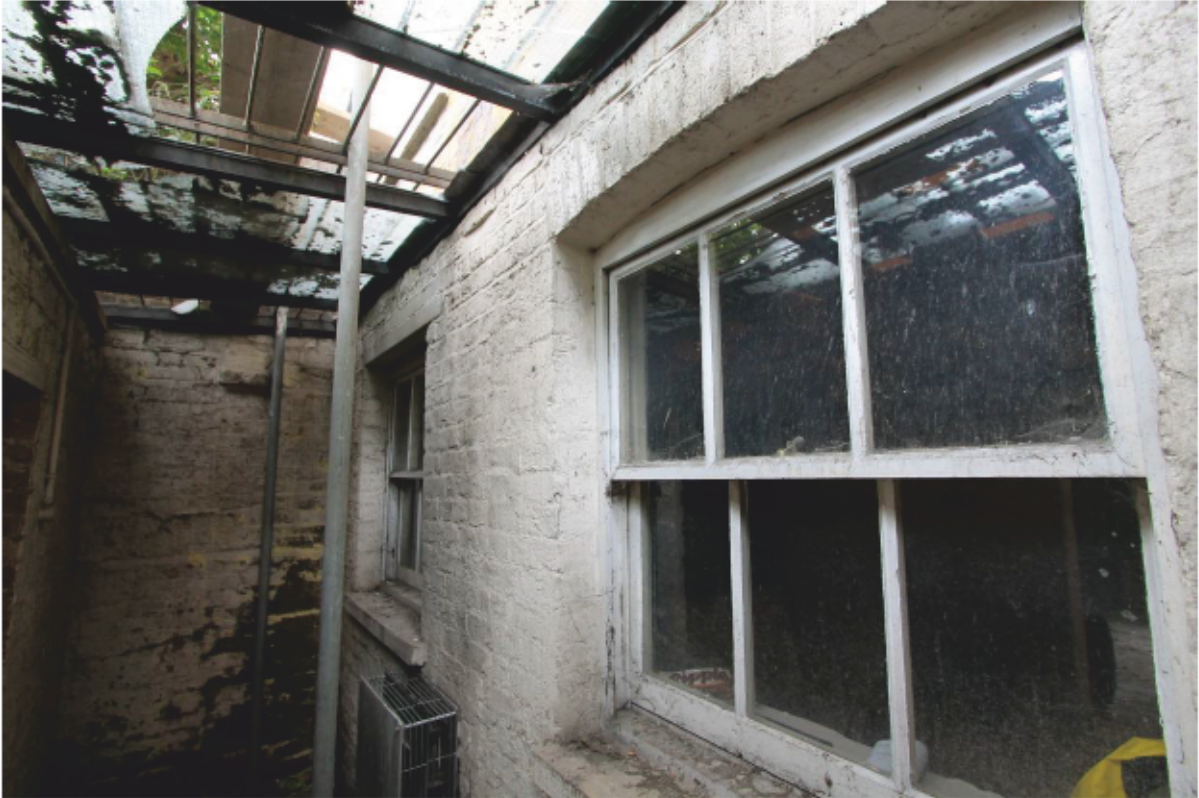
Plate 7 Light well between vaults and basement, looking east
