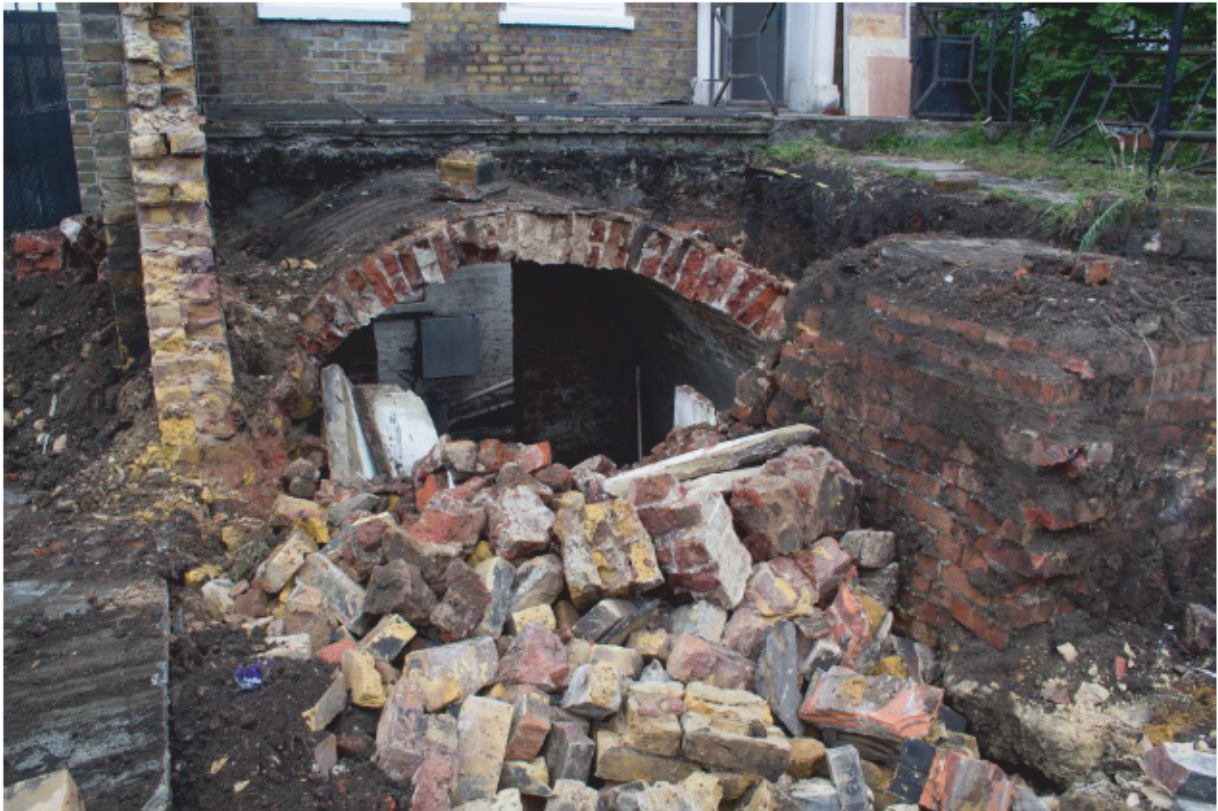
Plate 23 Vault during demolition
