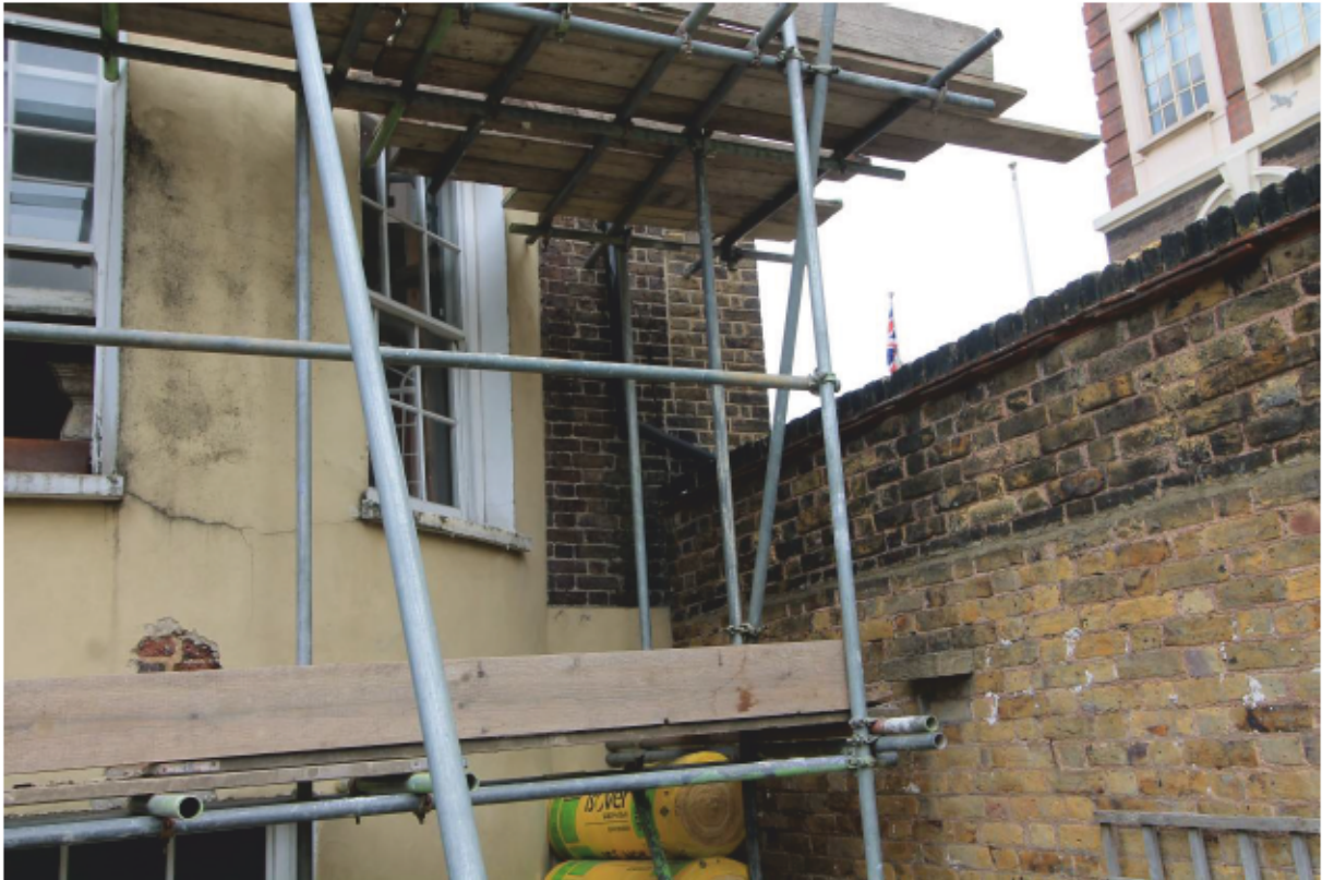
Plate 5 Straight joint to rebuilt eastern gable wall
