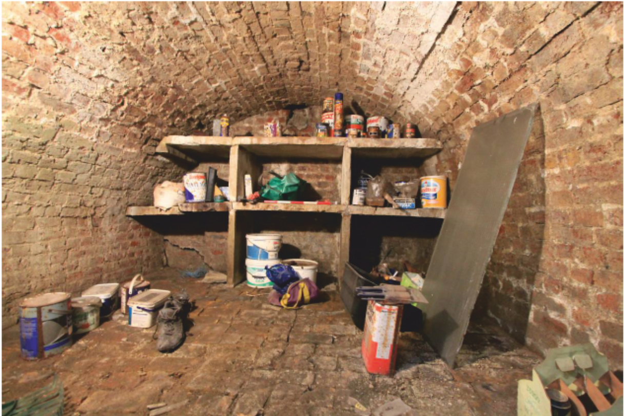
Plate 11 External (eastern) vault, looking south
