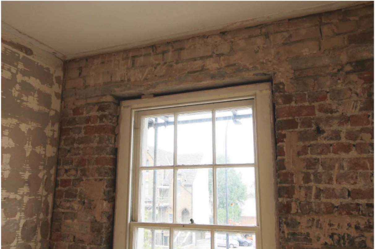
Plate 17 Rebuilt window head using concrete lintel (internal only)
