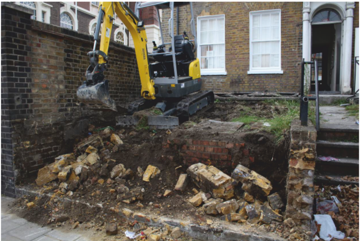
Plate 20 Removal of over-site
