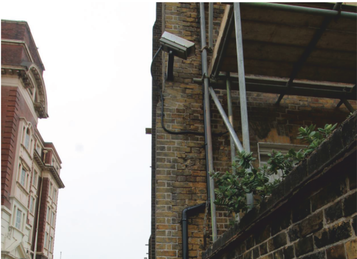
Plate 6 Rebuilt corresponding north-eastern corner
