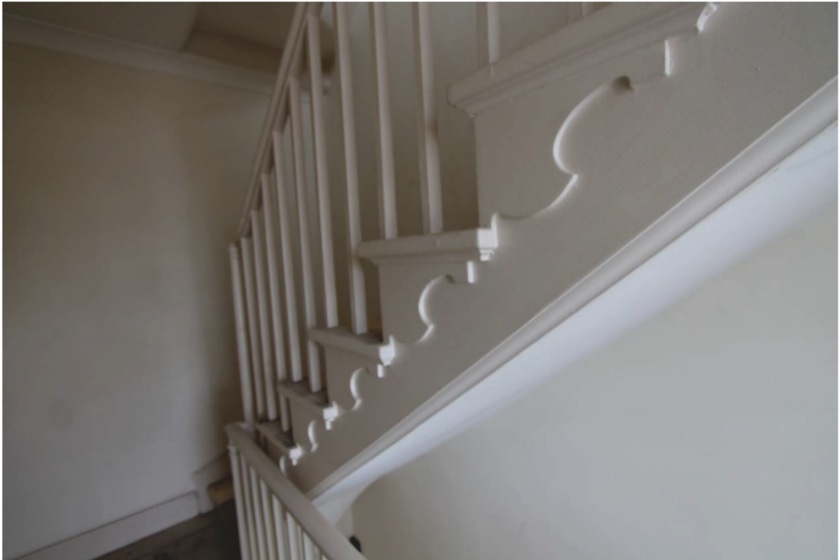
Plate 15 Original stair with moulded string
