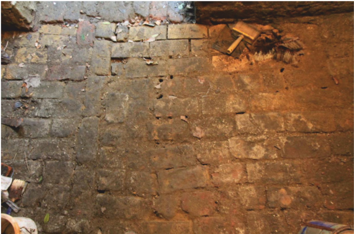
Plate 12 Brick floor (context 11) within external vault
