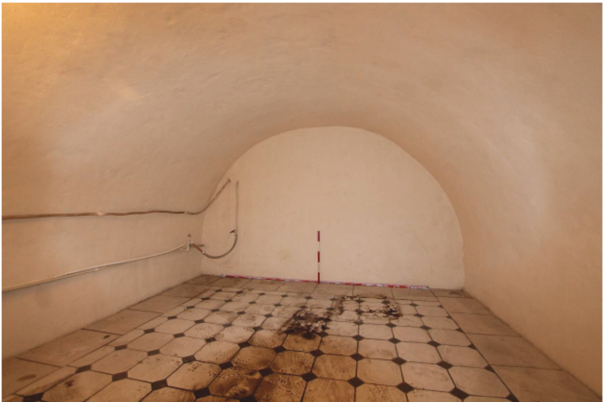
Plate 8 Internal (western) vault, looking north
