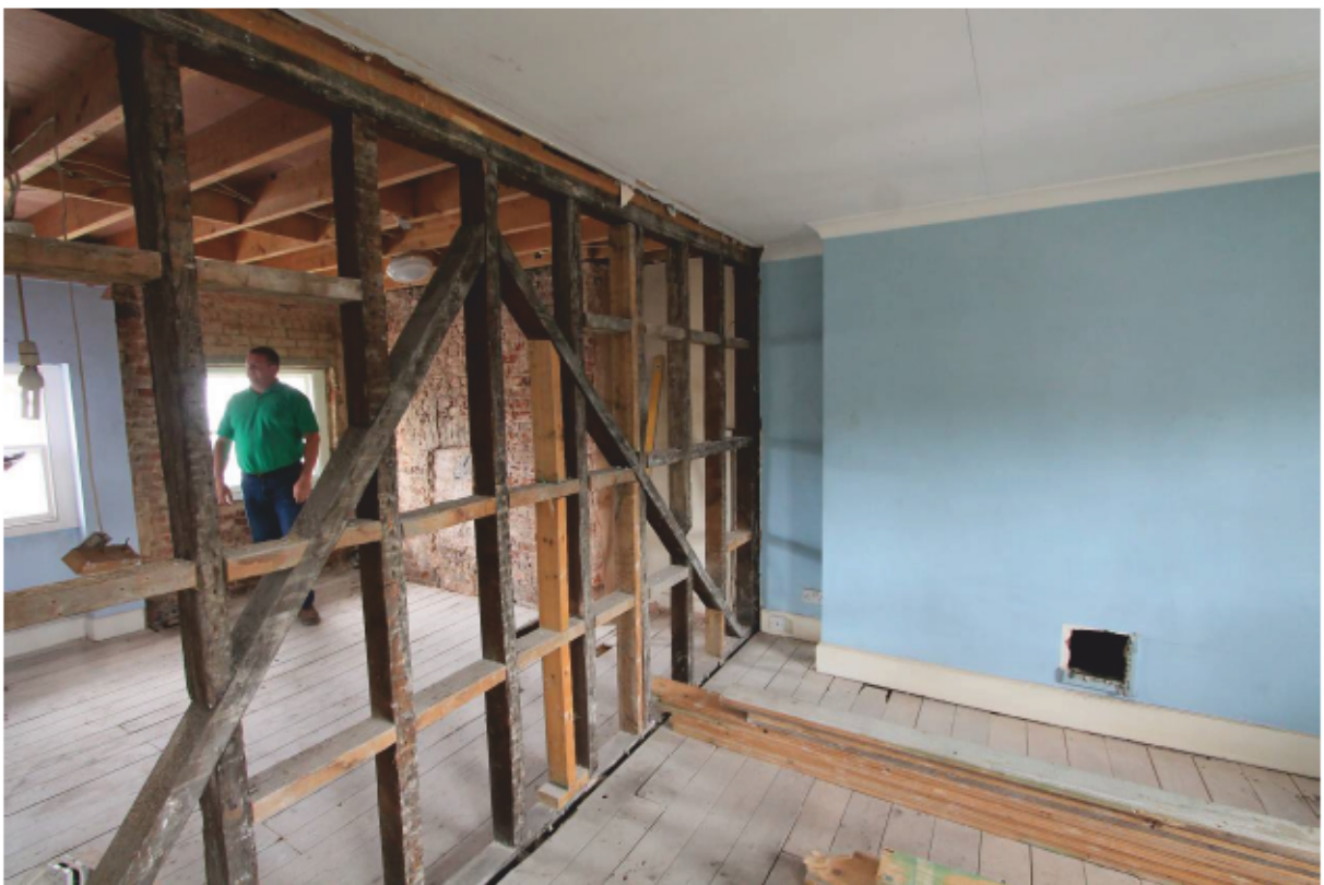
Plate 18 Original Softwood partition on second floor
