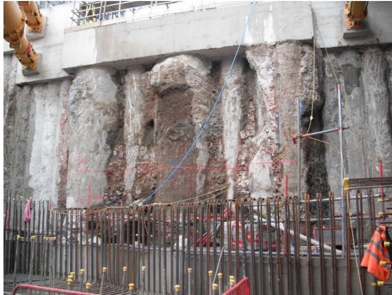
Plate 4: Dock wall truncated by concrete piles
