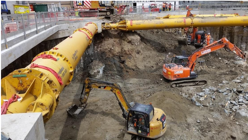
Plate 2: Bulk excavation showing sands
