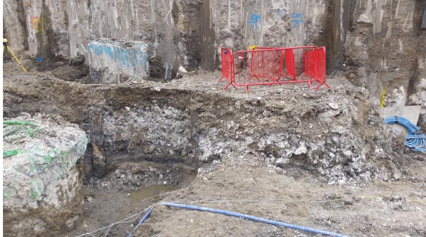
Plate 3: Excavation through chalk deposit [67], view east
