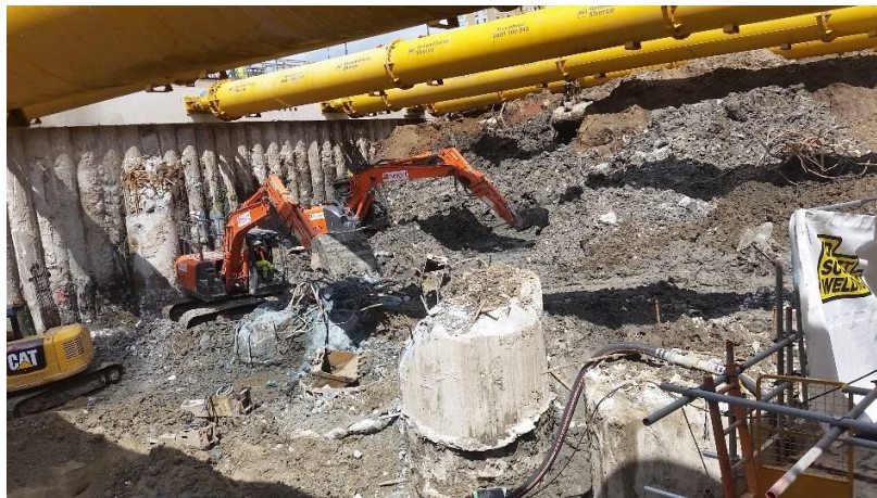
Plate 1: Watching brief excavation area, view northwest
