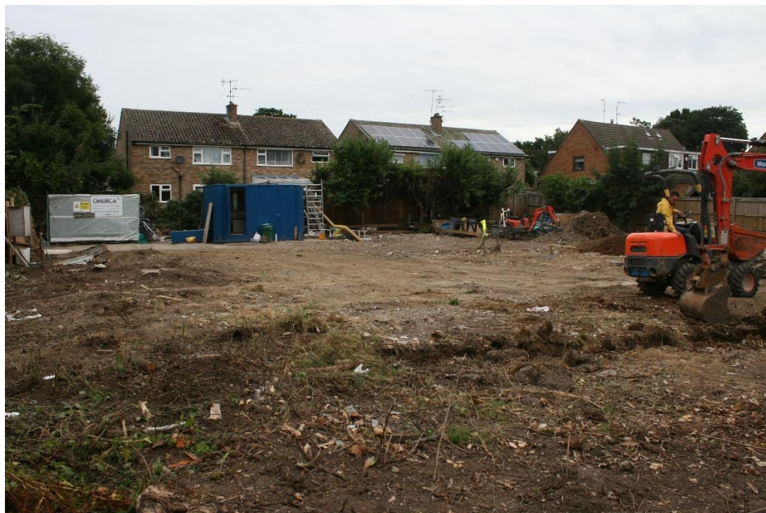
Plate 1: General site shot looking northeast, (KBCE16 (4))
