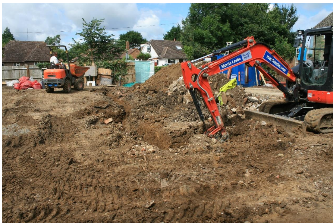
Plate 5: Excavation shot of House 2 (Trench 2), looking southwest (KBCE16 (26))
