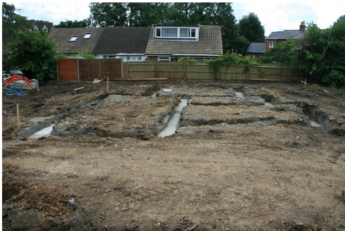
Plate 10: Trench 1 following poured cement foundations, looking south (KBCE16 (29))
