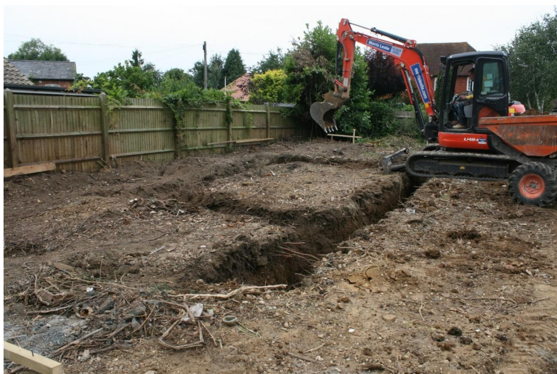
Plate 2: Excavation shot of trench 1, looking southwest, (KBCE16 (6))
