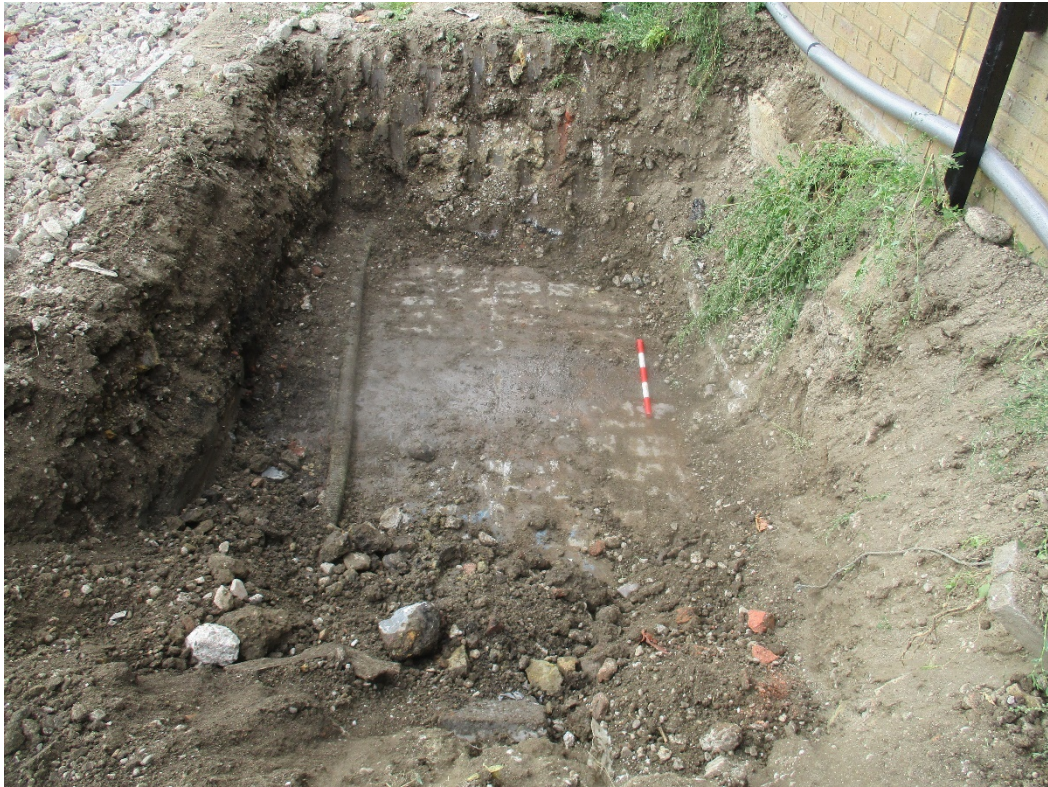
Plate 3. South facing shot of post-med. road surface [63] exposed in Tr. 20
