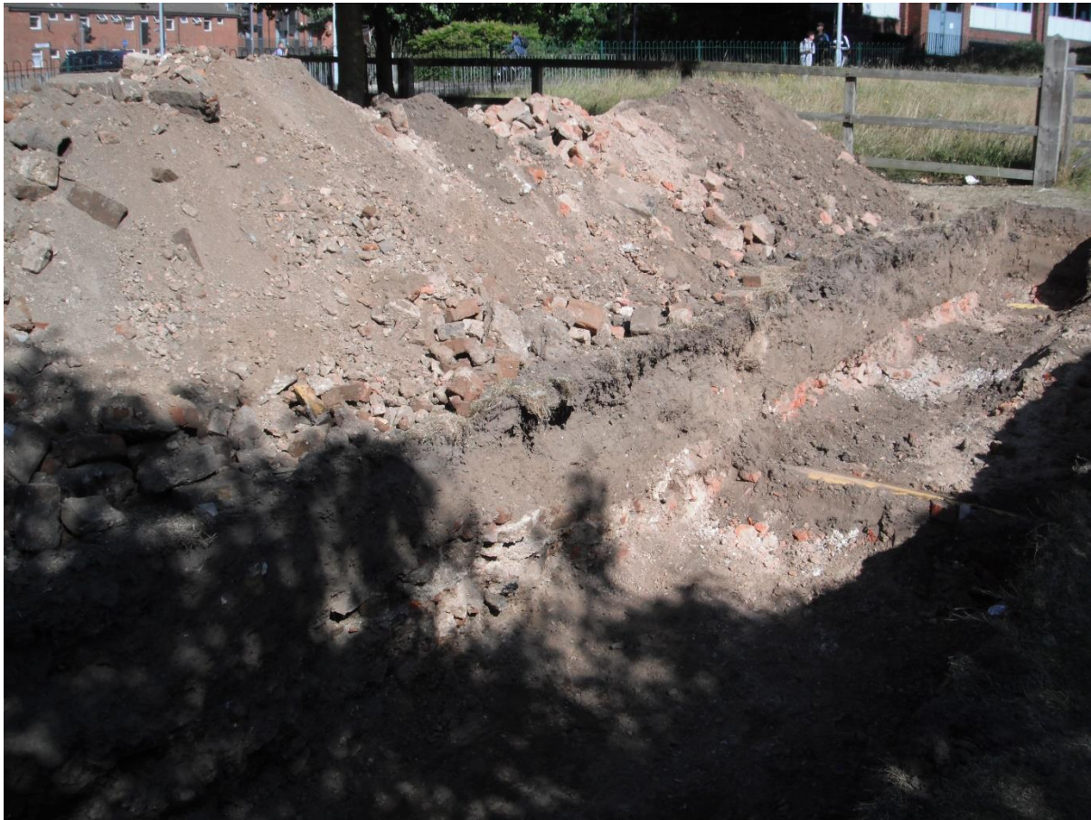
Plate 5: Looking northeast, 1980s demolition and made ground [1] truncated by modern gas pipes
