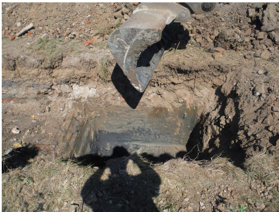
Plate 15: Trench 44 modern made ground [45] to 1.80 m + view north.
