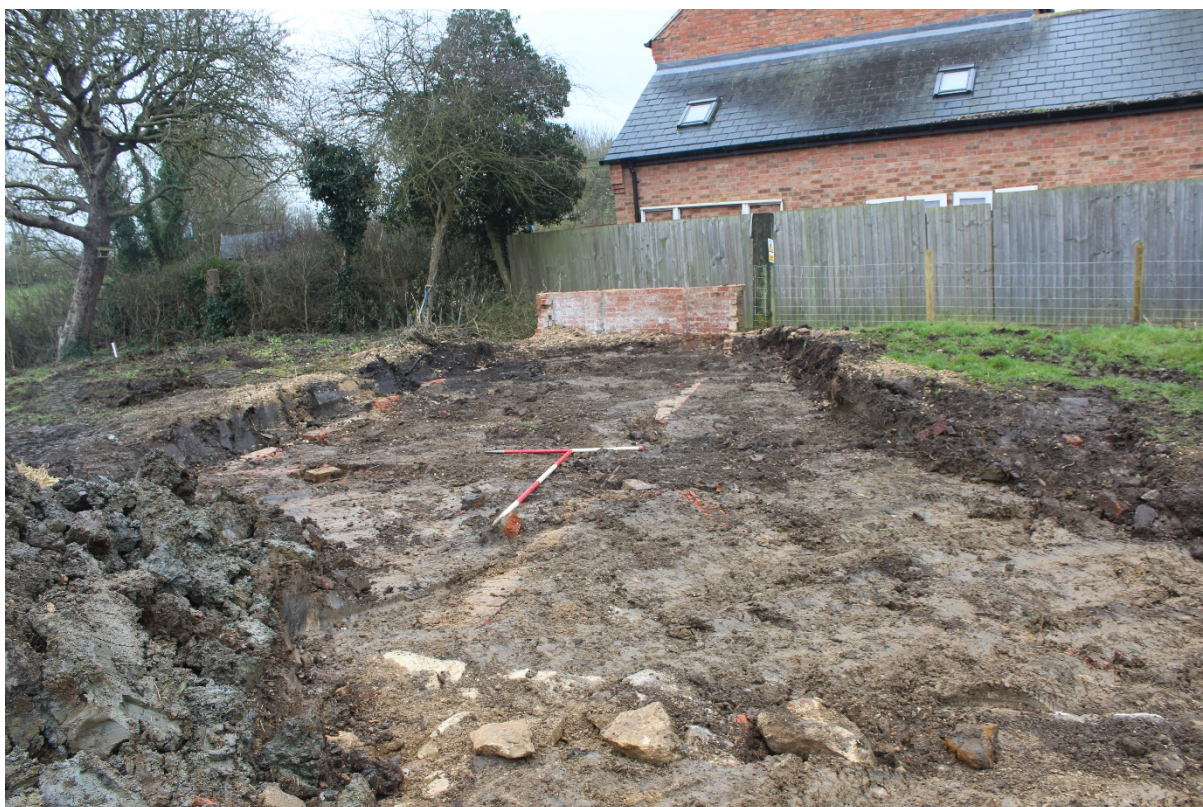
Plate 3: Shot of barn footings (106). Shot is taken from the north.
