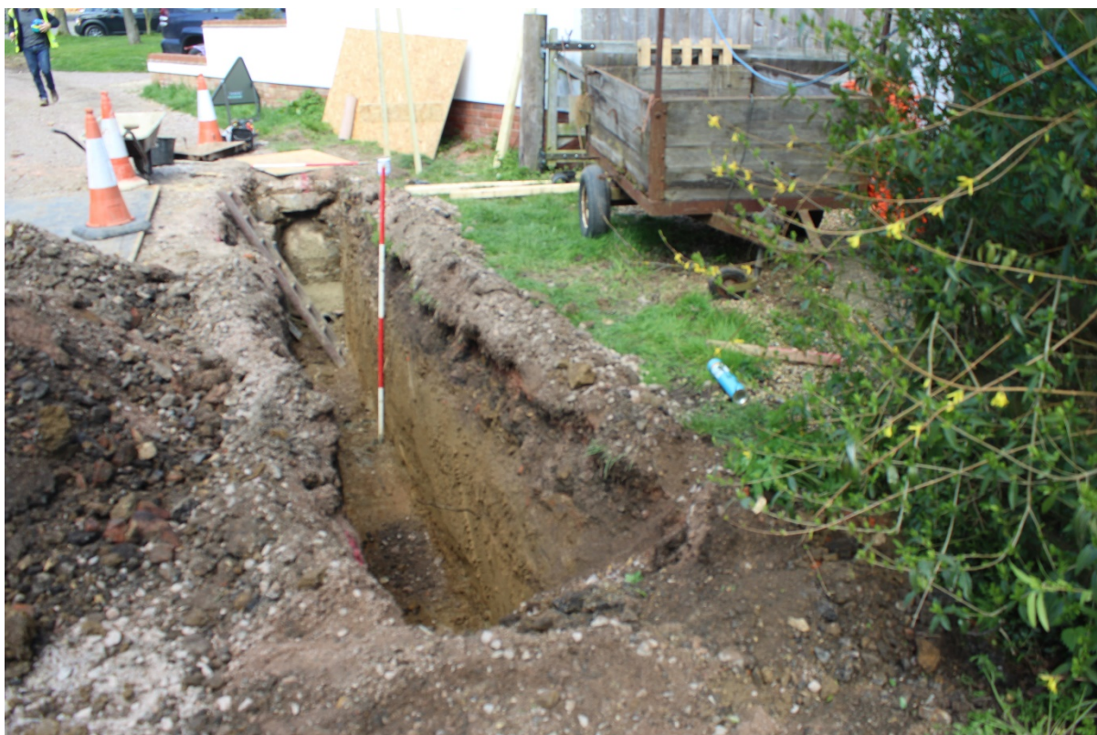
Plate 6: Section 7, drainage trench. Shot is taken from the southeast.
