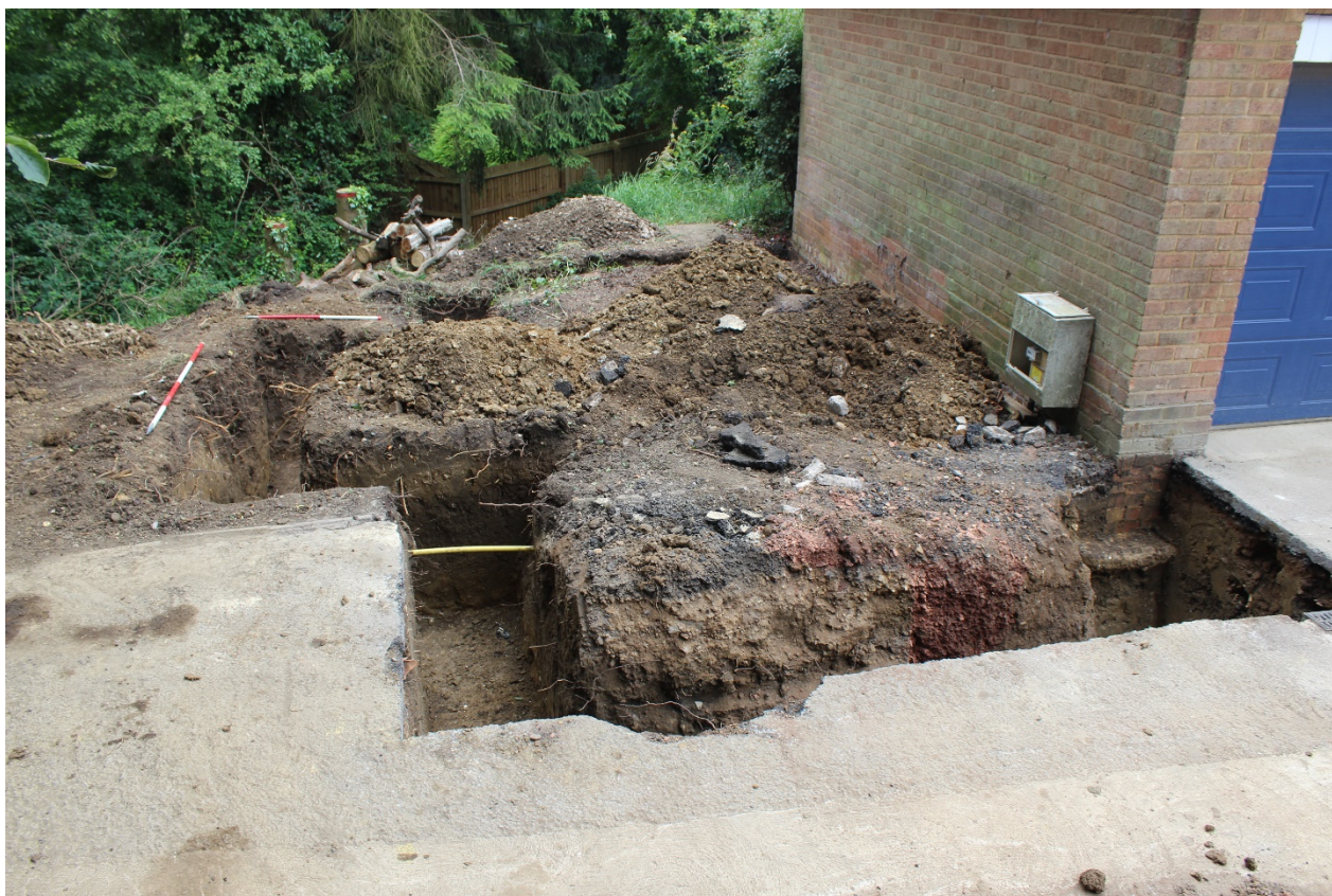
Plate 1: View of garage footings area, taken from south-west.
