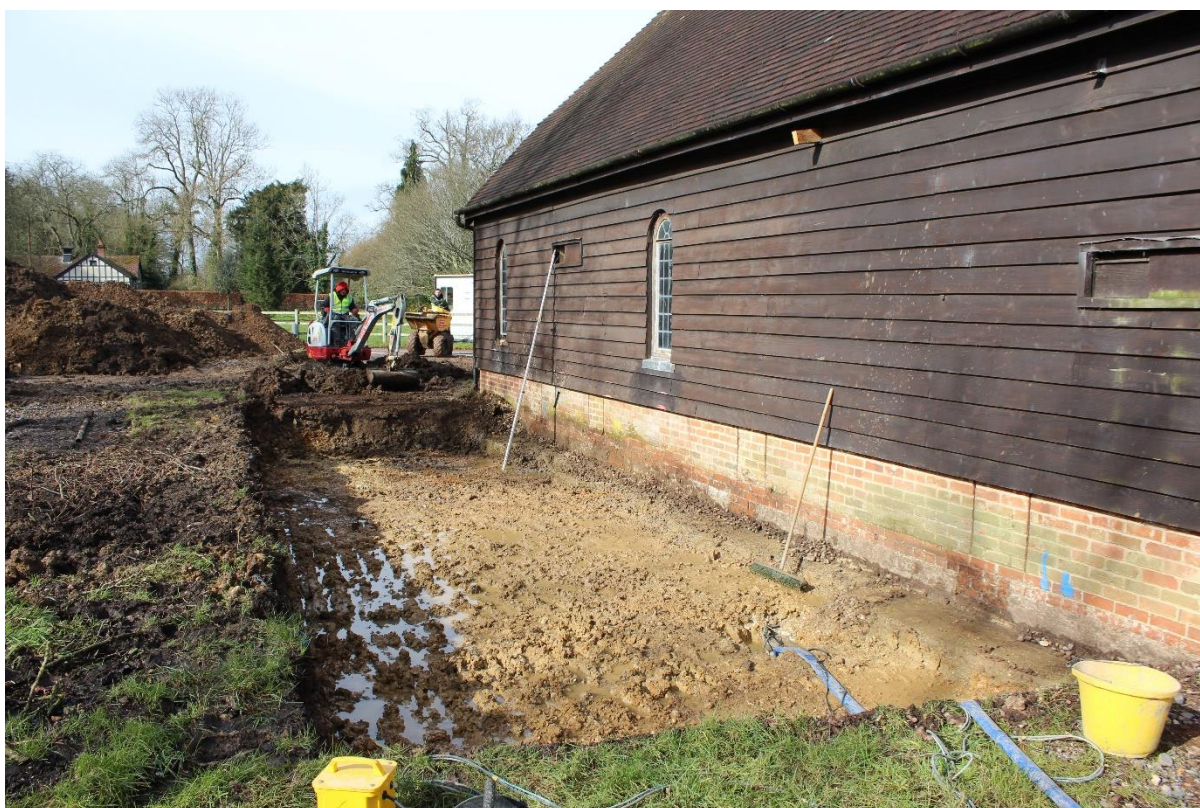
Plate 6 View to the west of Area B (showing lower excavation level)
