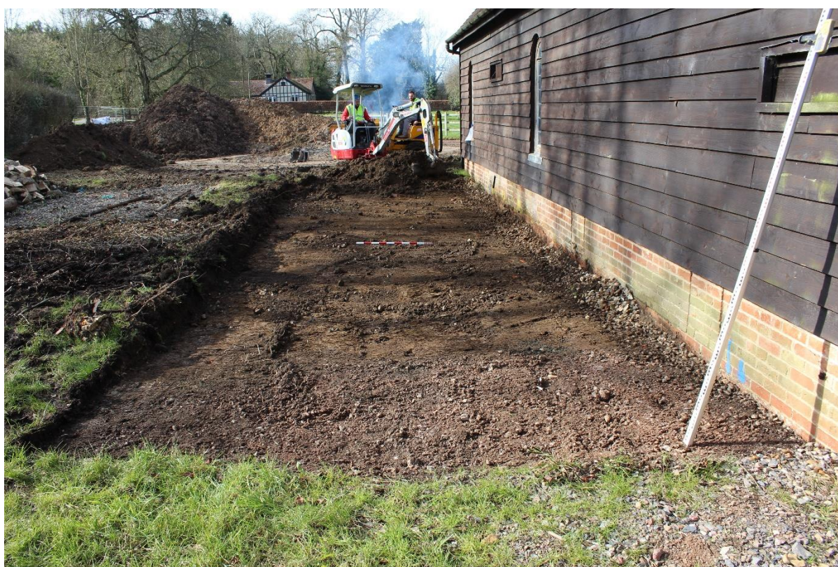
Plate 4 View to the west of Area B
