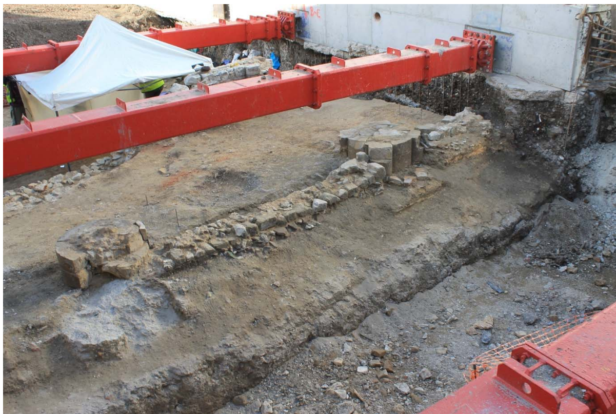
Plate 5: Looking southwest at the post-medieval wall [599]/[600] with the medieval columns [902] and [903] incorporated in the build
