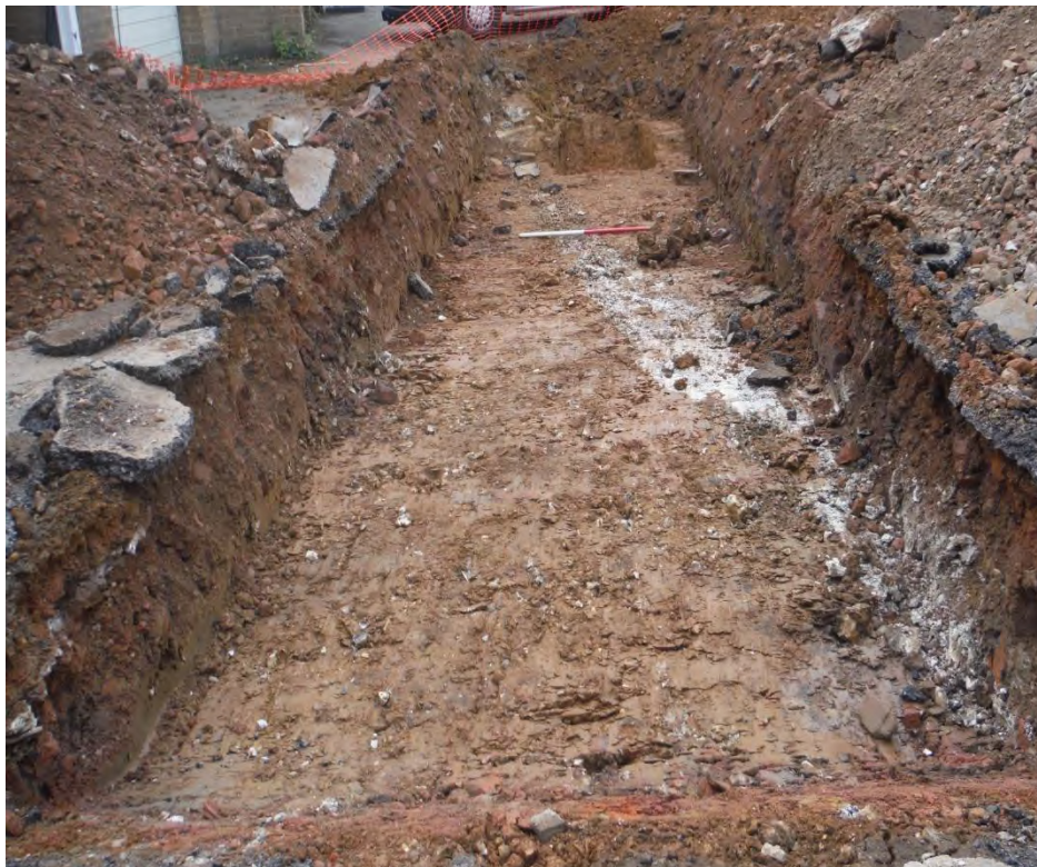
Plate 8: Trench 8 view south
