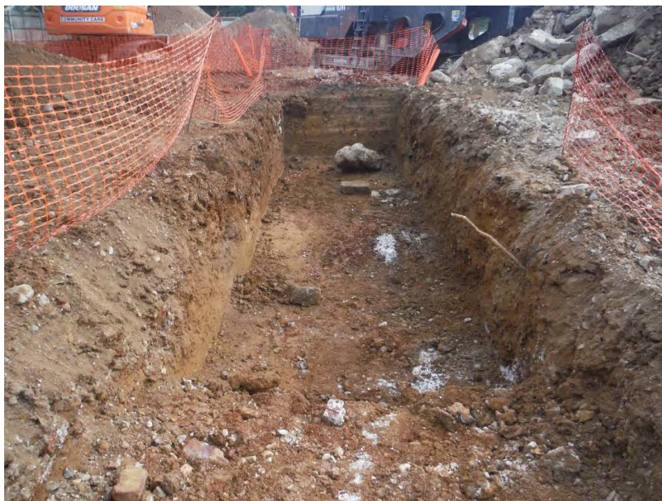
Plate 5: Trench 5 view east
