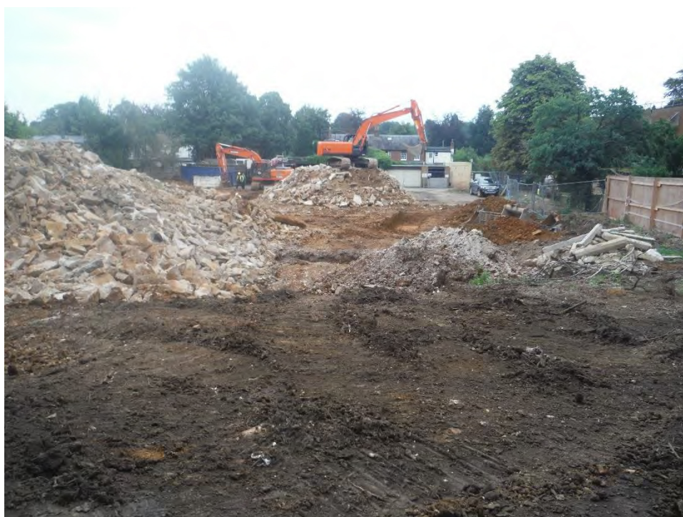
Plate 10: View east towards site entrance.
