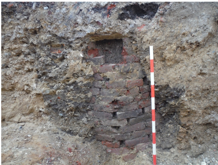
Plate 6: South facing view of soakaway [4] in Trench 4
