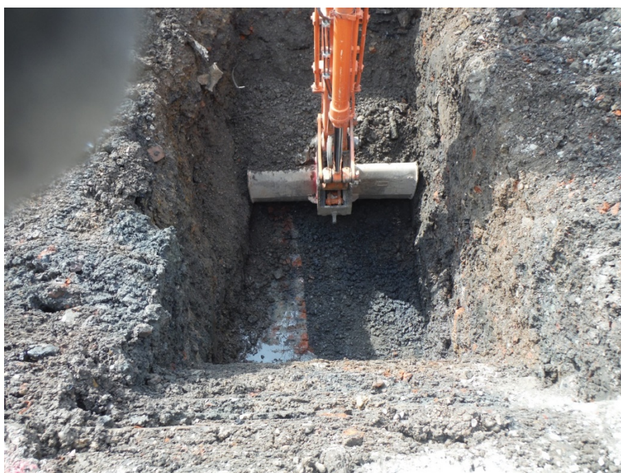
Plate 7: West facing view at east end of Trench 8 showing wall foundation [9]
